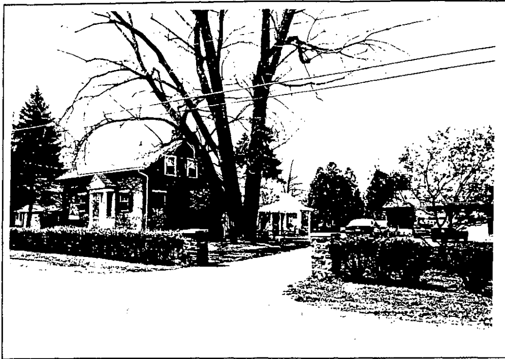
4030 Rensch Road. East and north elevations.
