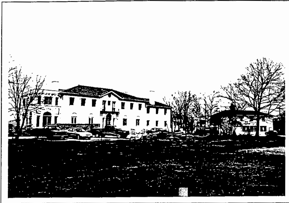
Crouch-Waite Mansion (Rosary Hall) Daemen College Campus, 4380 Main St. West and south elevations.
