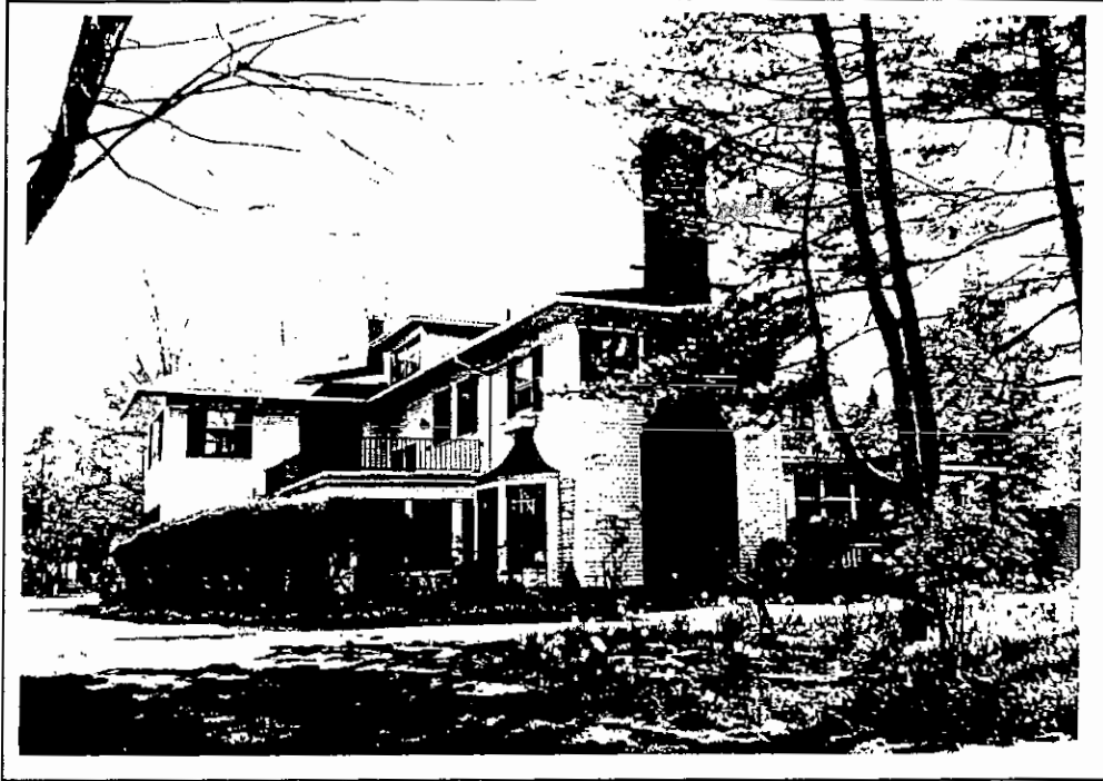
305 Brompton Road, east and north elevations.
