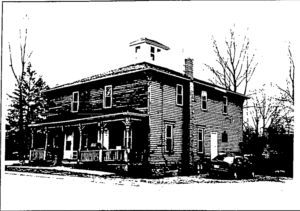
260 Campbell Blvd. East and north elevations.
