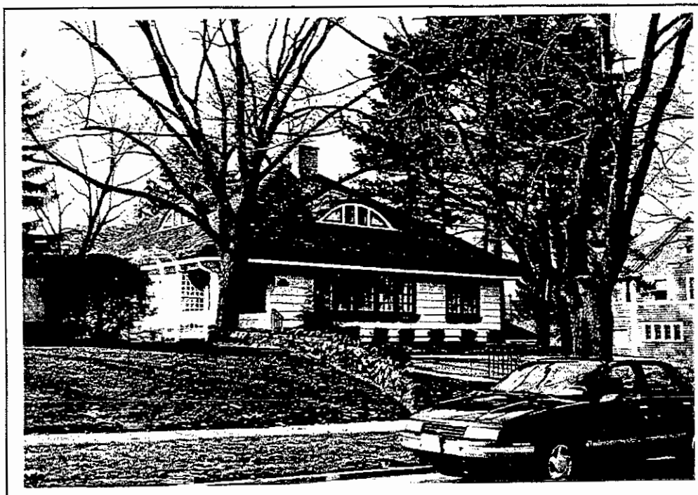
South and east elevations.
