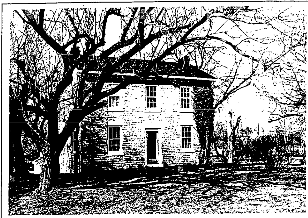
Fogelsonger House, 219 Park Club Lane. South elevation.
