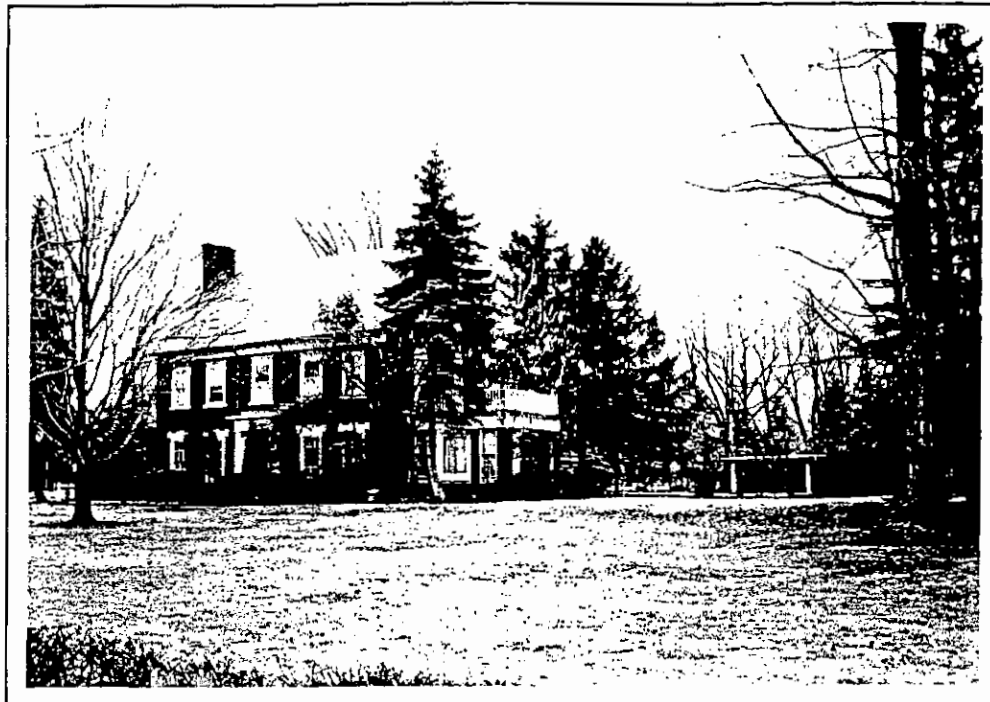
381 LeBrun Rd. North and west elevations.
