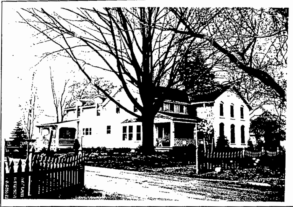
459 South Ellicott Creek Rd. East and north elevations.
