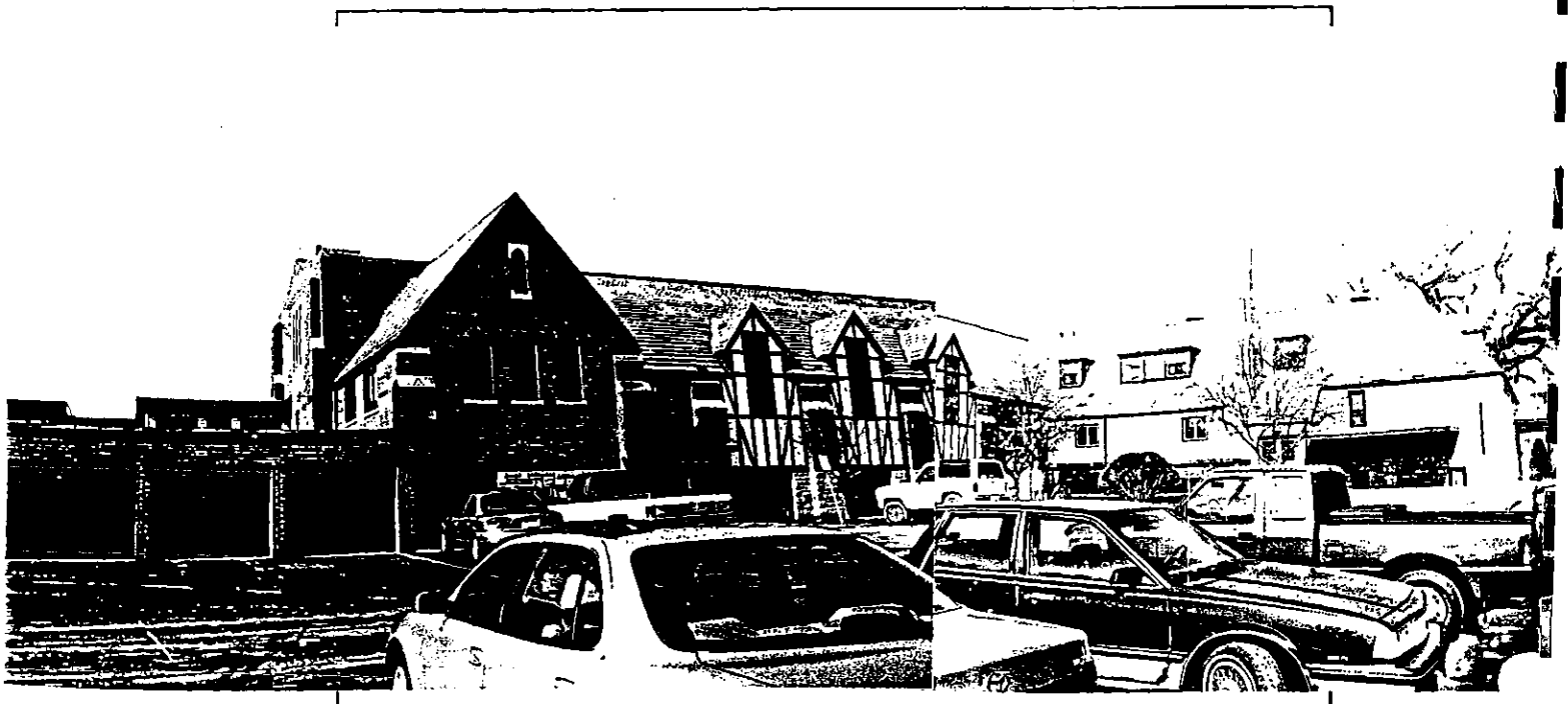
East and south elevations. View from courtyard.
