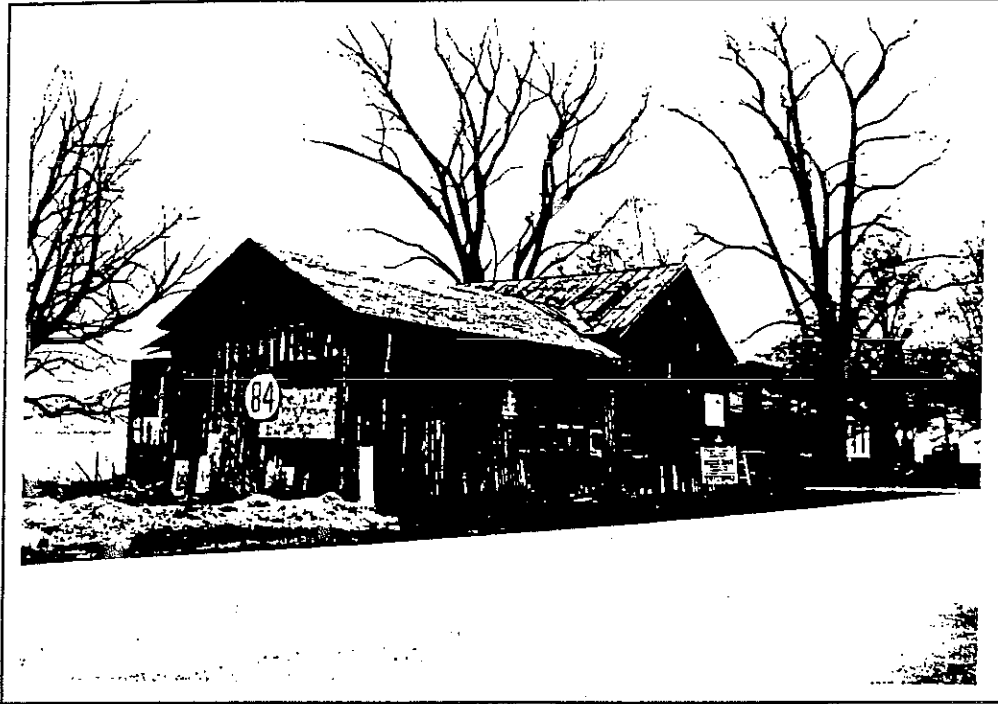
Barn at 1899 Campbell Blvd. North and west elevations.
