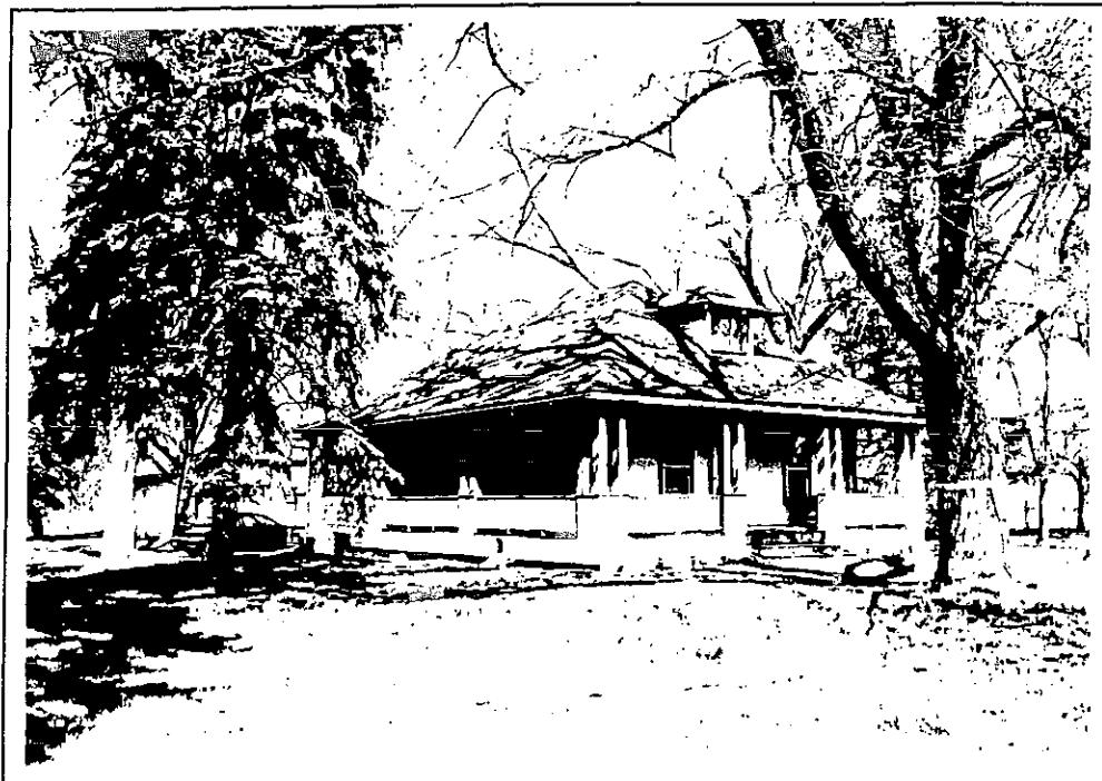
1000 North Forest Rd. South and east elevations.
