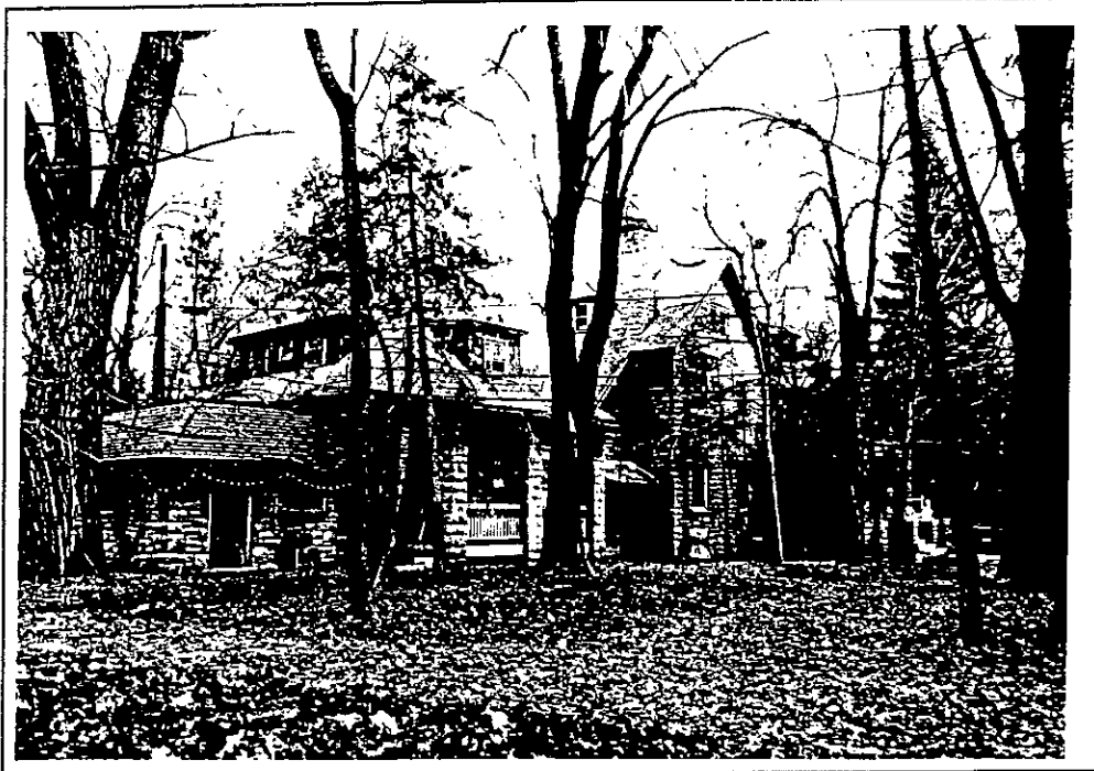
50 Getzville Road. West and south elevations.
