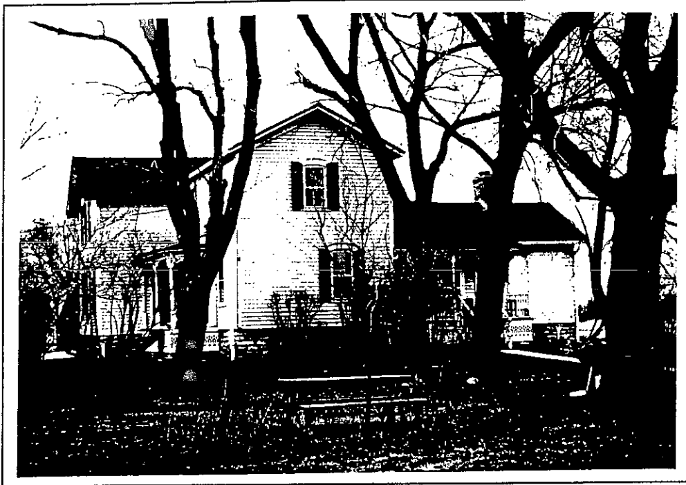
1025 New Road, west and south elevations.
