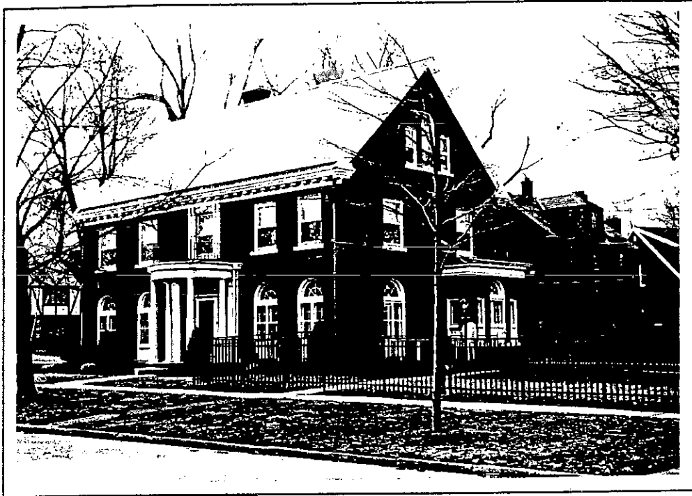
48 Park Circle. East and north elevations.
