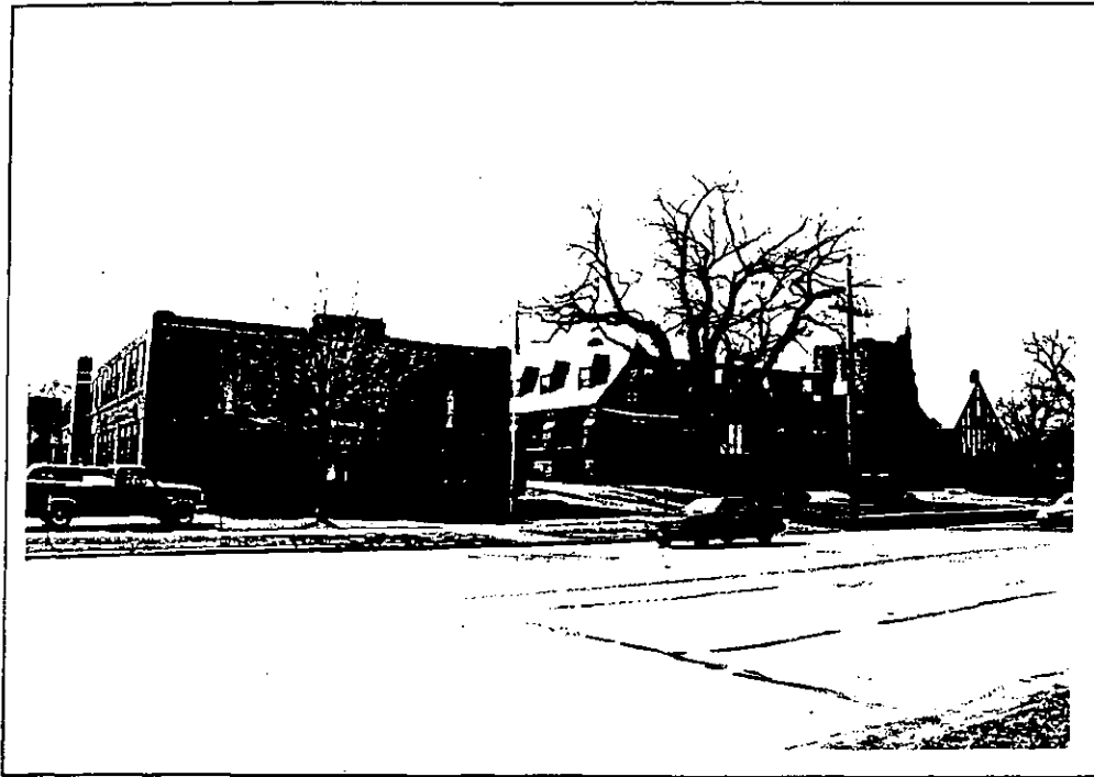
Christ the King School and Church, 30 Lamarck Drive, corner of Main St. East and north elevations.
