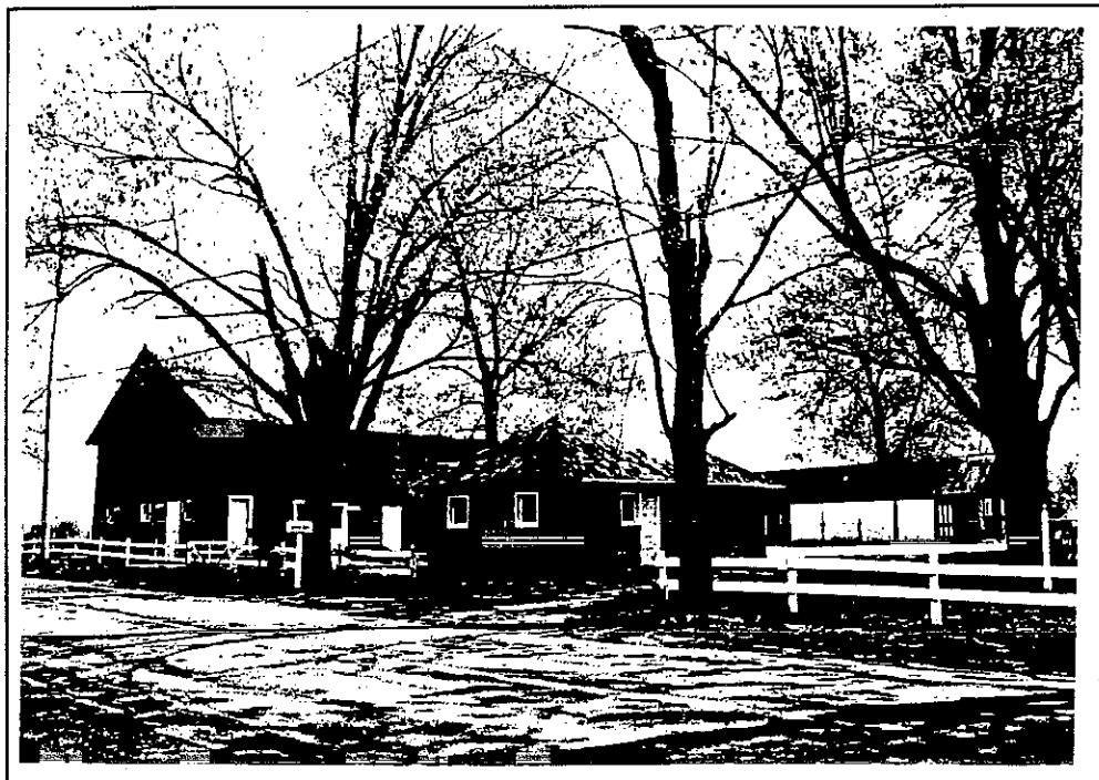
Outbuildings east of the house. North and west elevatons.
