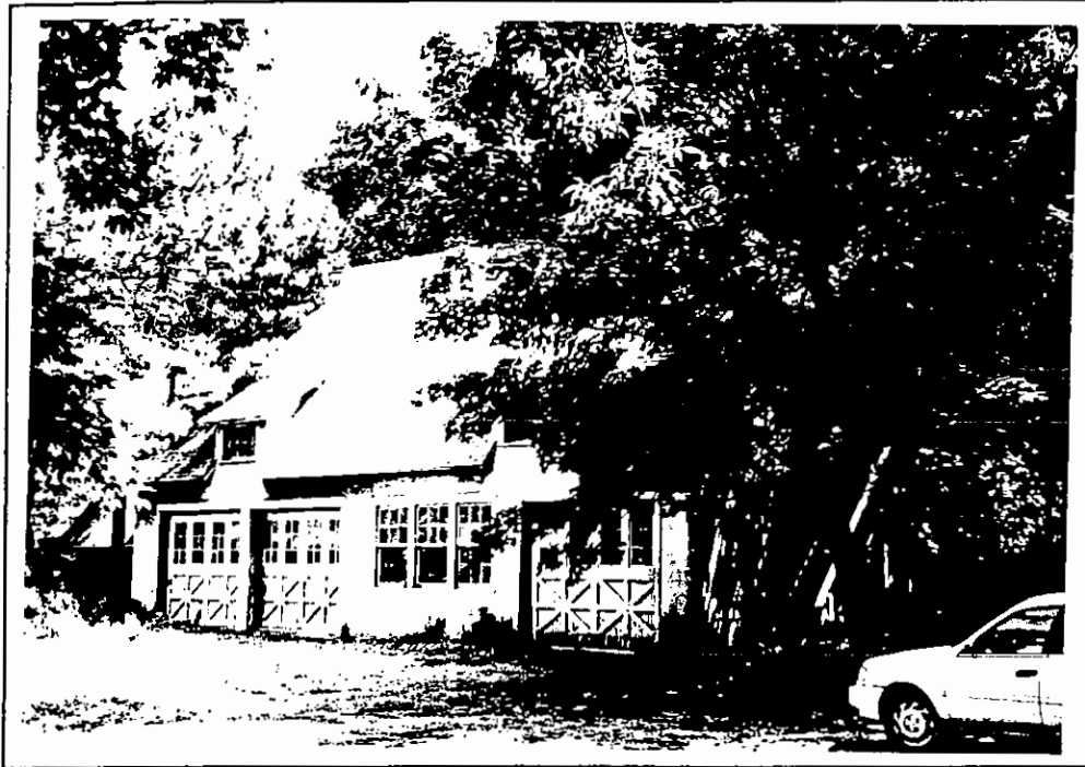
Barn behind 4196-4230 Main Street. West elevation.
