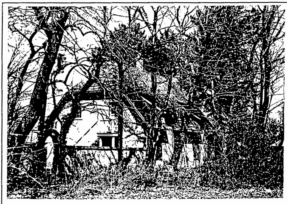
Barn behind 4196-4230 Main Street. South and east elevations.
