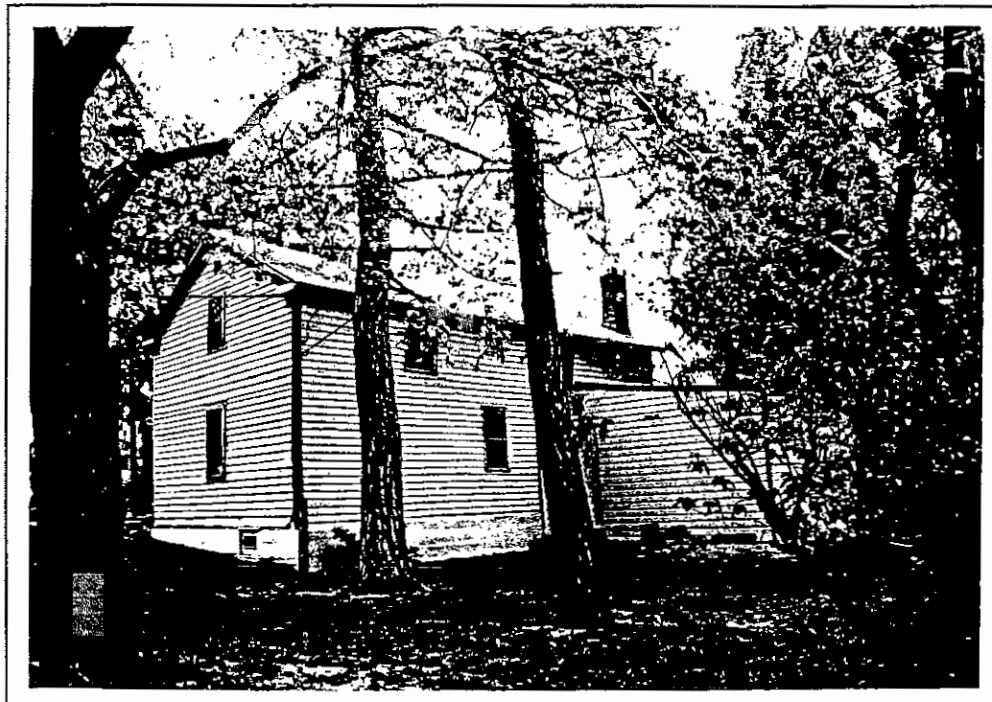
North and west elevations.
