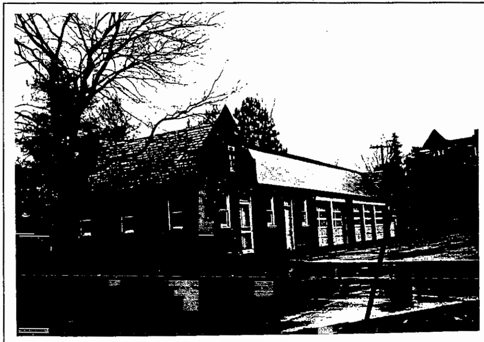
Garage. North and west elevations.
