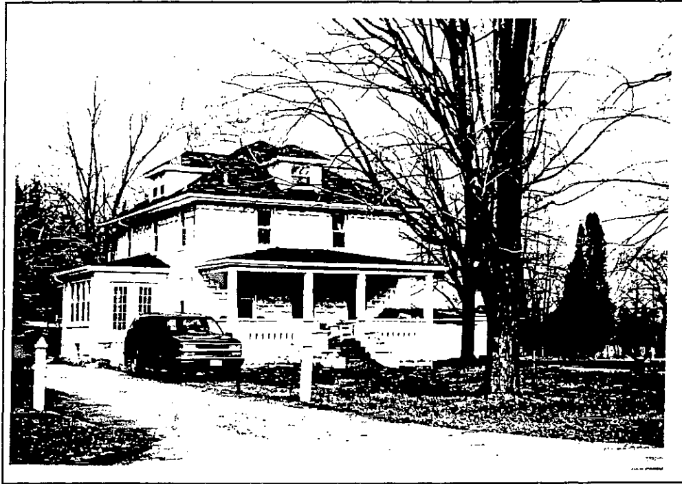
9980 Transit Road. South and east elevations.
