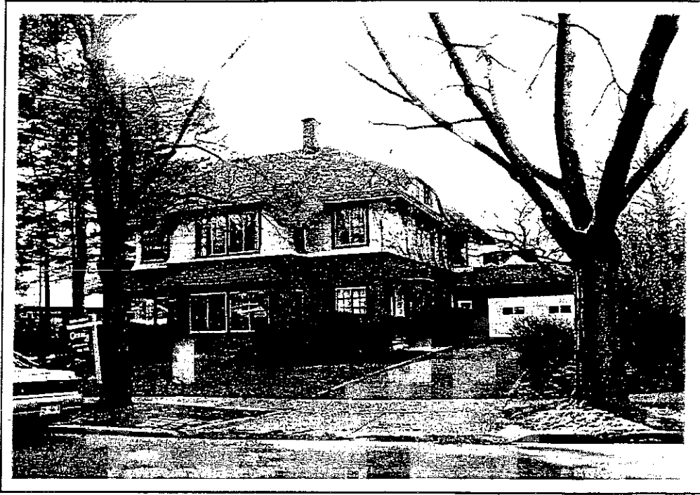
5 Berryman Drive. East and north elevations.
