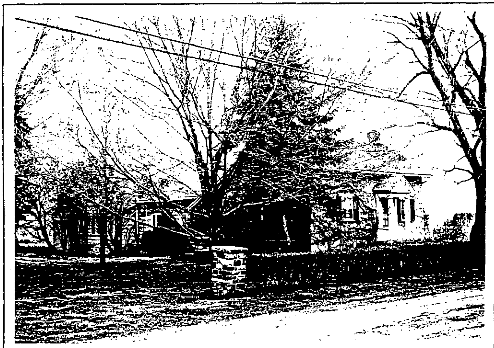
South and east elevations.
