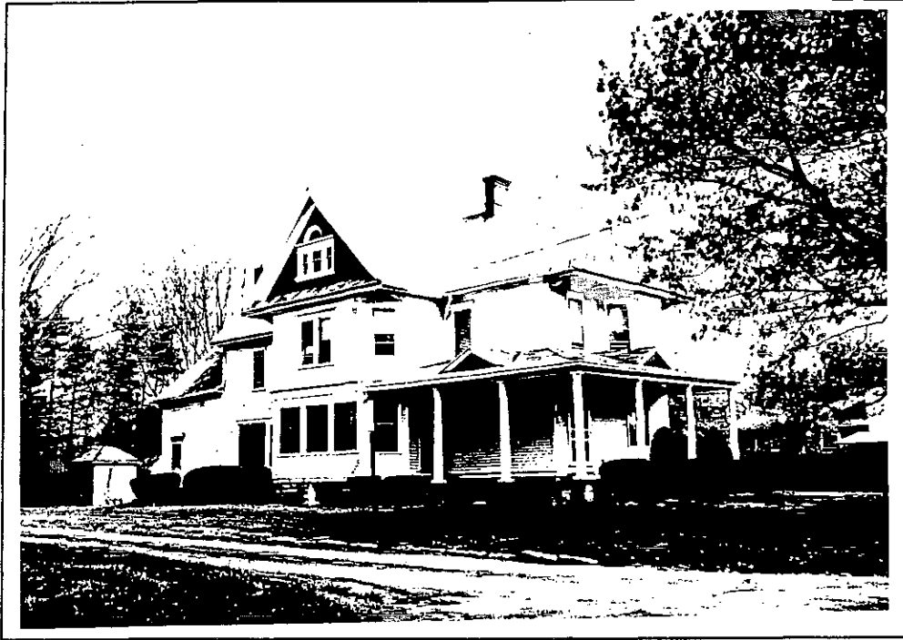
954 North Forest Road. South and east elevations.
