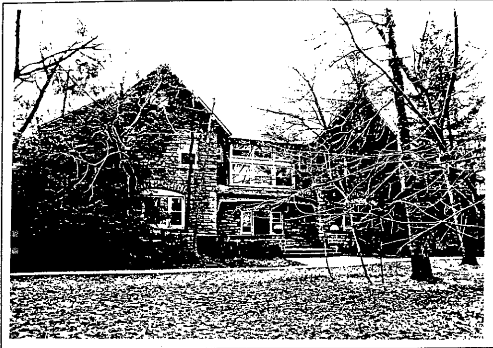
50 Getzville Road. North elevation.
