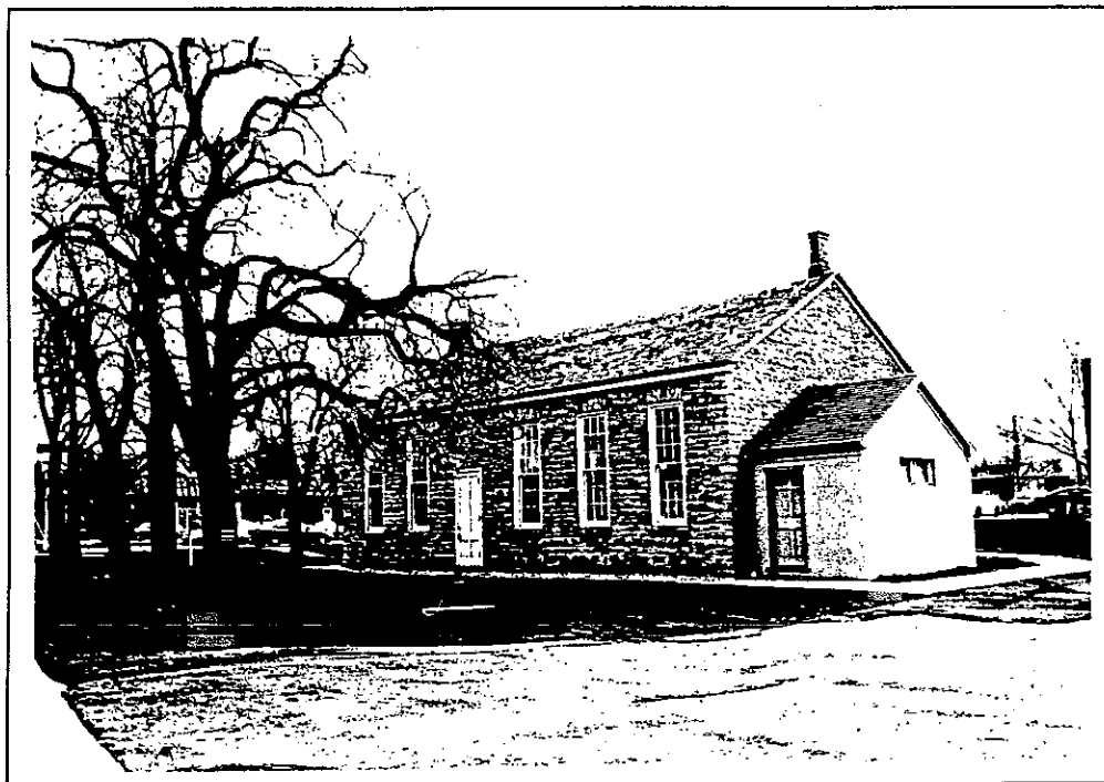
East and north elevations. View from North Forest Rd.
