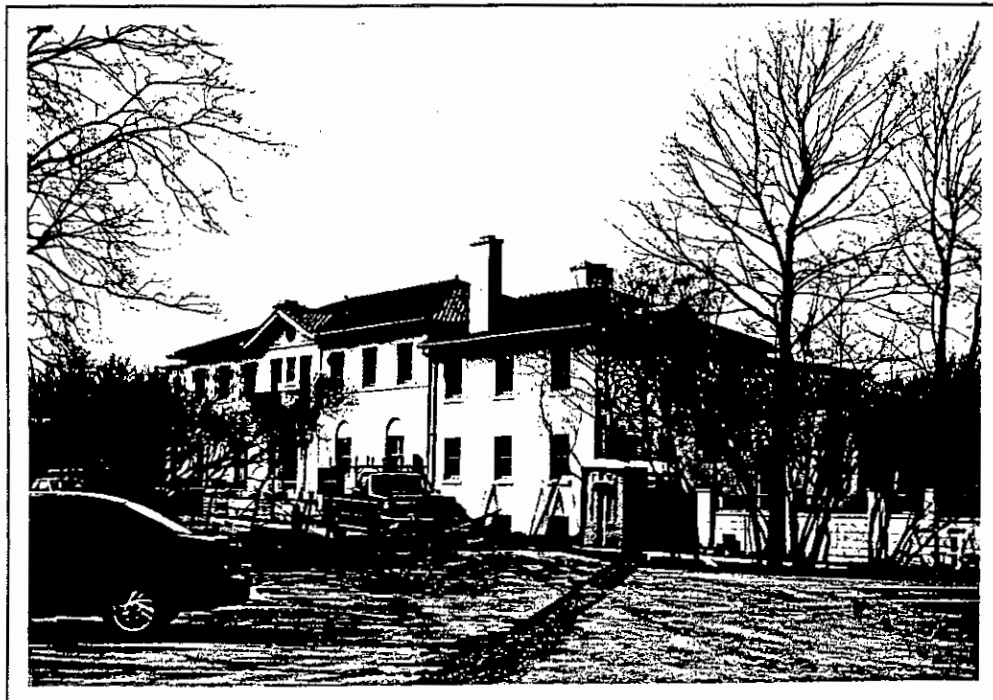
South and east elevations.
