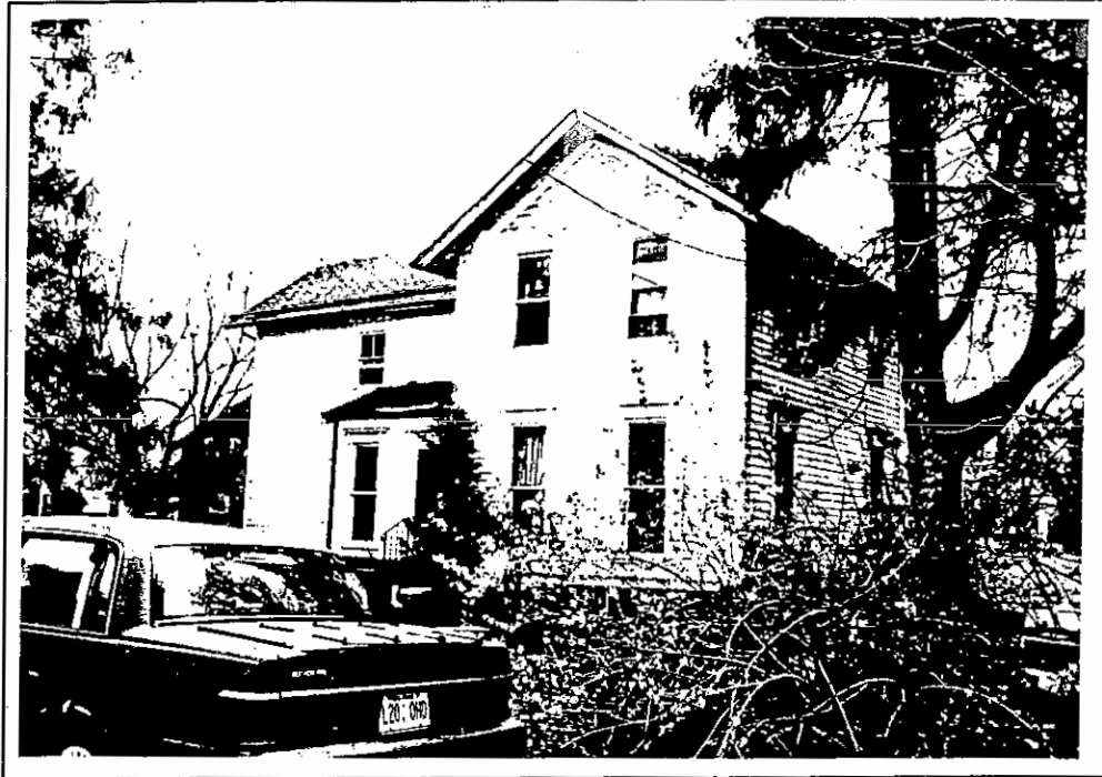
215 Brenon Road. North and west elevations.
