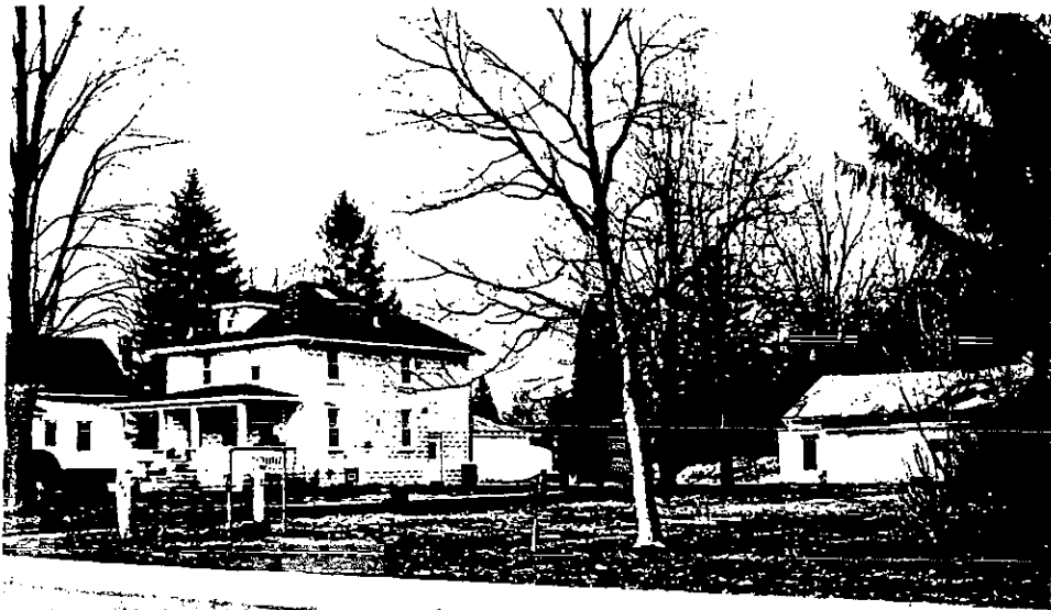
East & north elevations. Garage at right.
