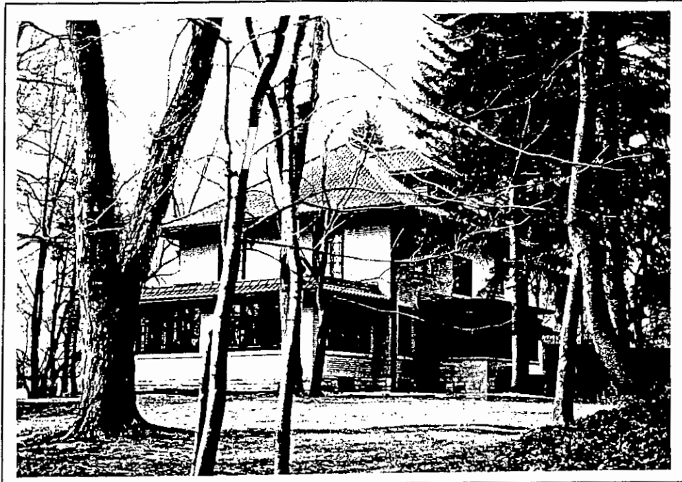
32 Ivyhurst Road. East and north elevations.
