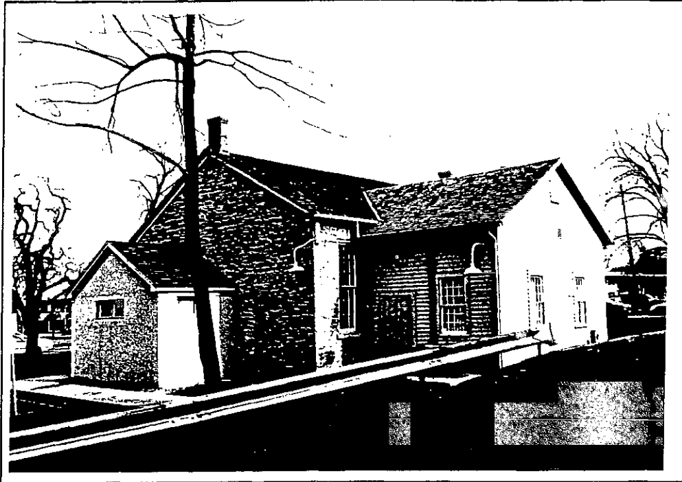
Mennonite Meeting House, 5178 Main St. North and west elevations.
