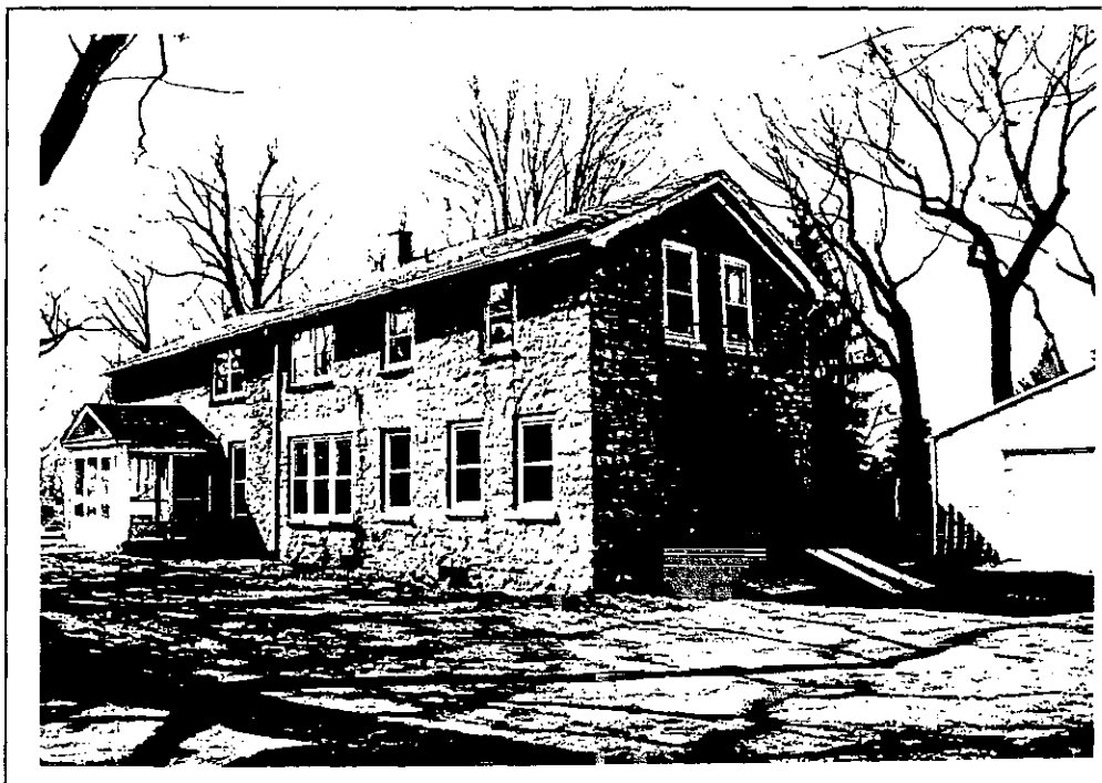
South and east elevations.
