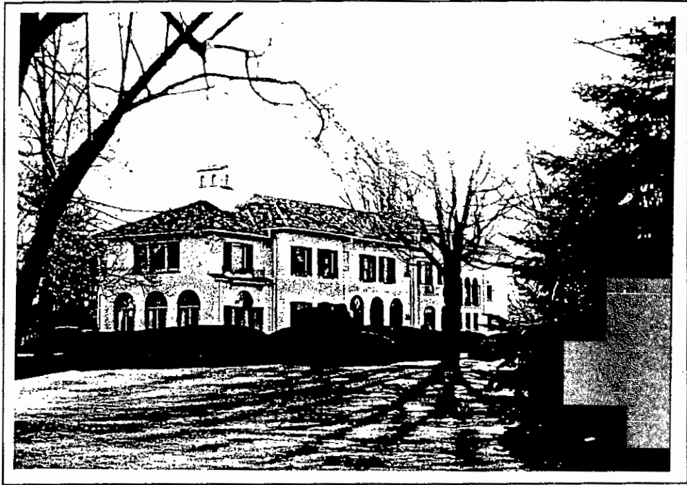
726 LeBrun Road. East and north elevations.
