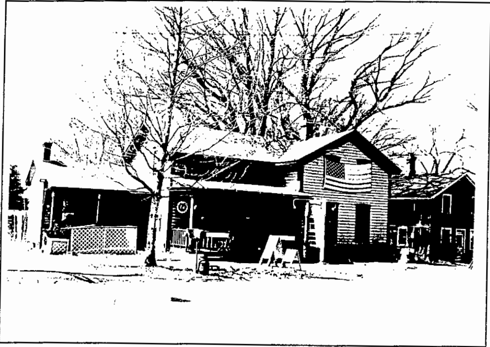
9920 Transit Road. South and east elevations.
