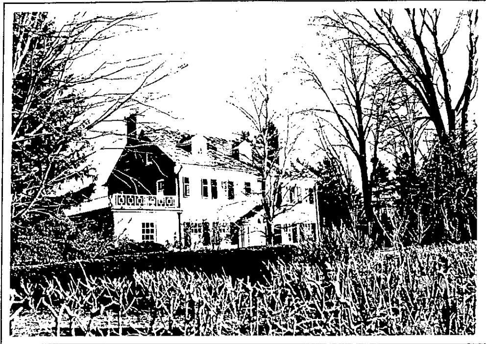
725 LeBrun Rd. North and west elevations.
