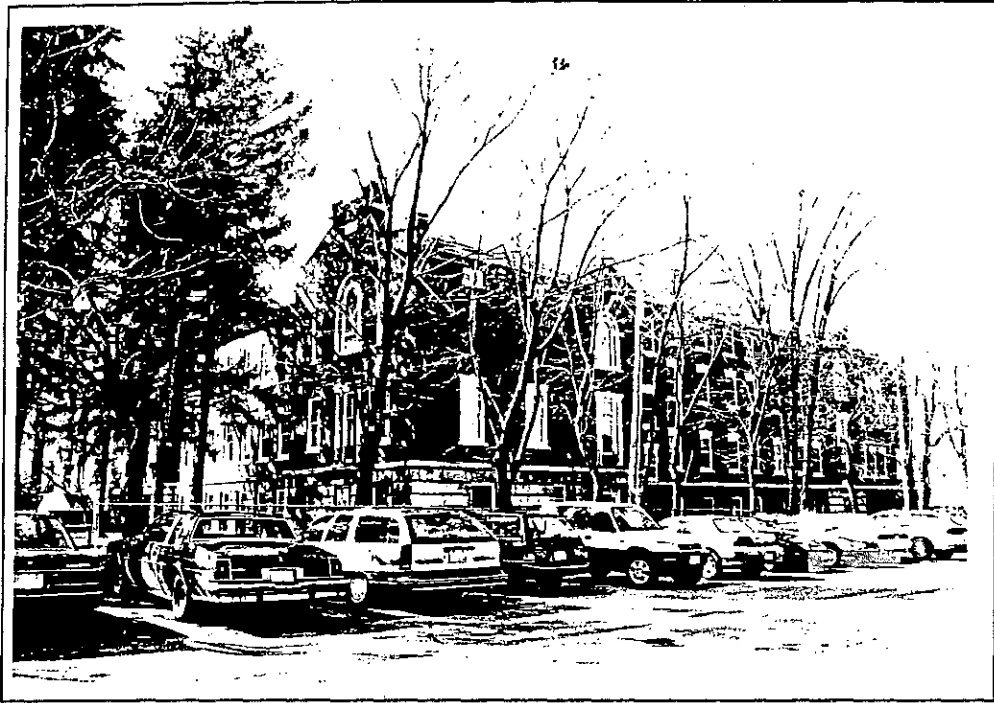
Buffalo Academy of the Sacred Heart, 3860 Main Street. South and east elevations.
