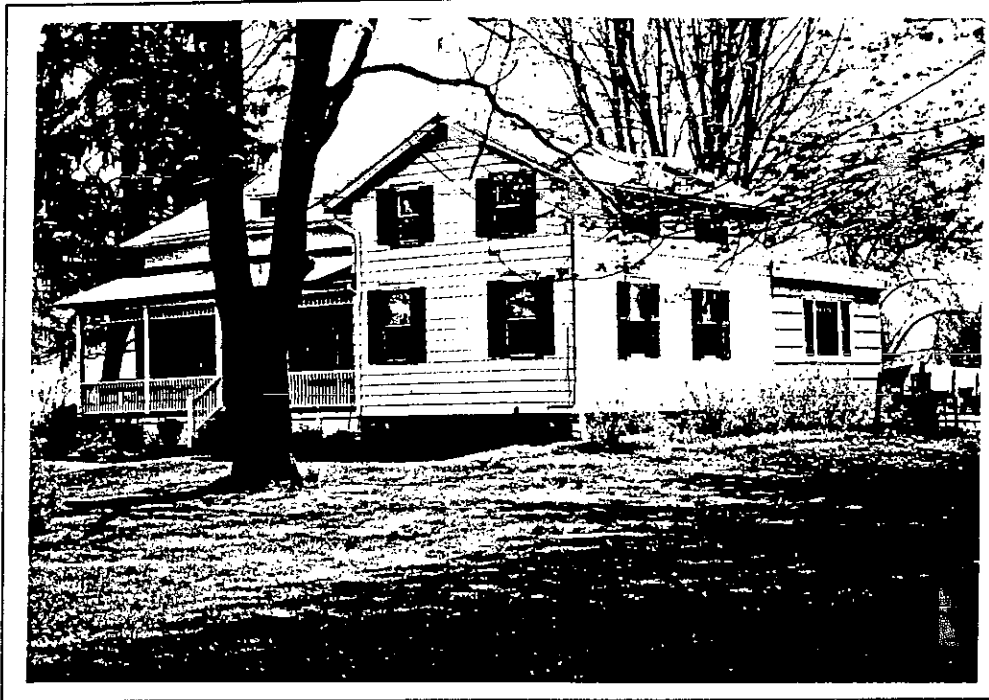
405 Schoelles Road. North and west elevations.
