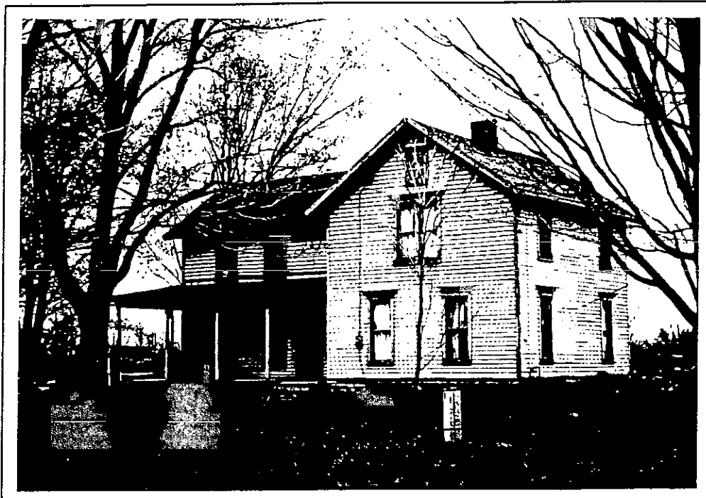
1899 Campbell Blvd. West and south elevations.
