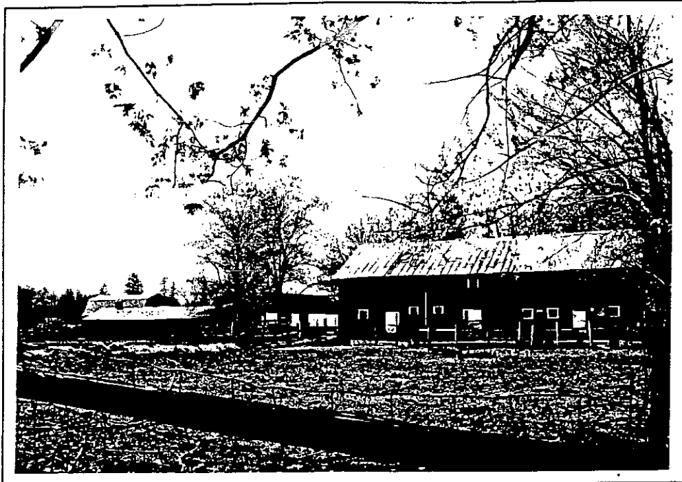
Outbuildings at 405 Schoelles Rd. located east of the house. East and north elevation.
