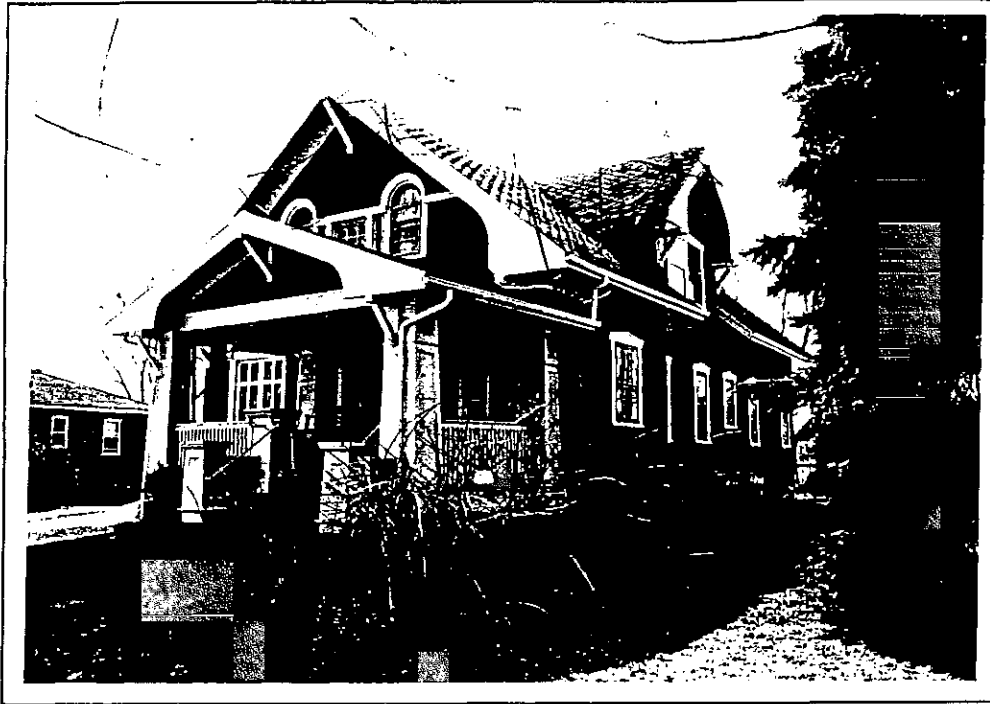
89 Royal Parkway. East and north elevations.
