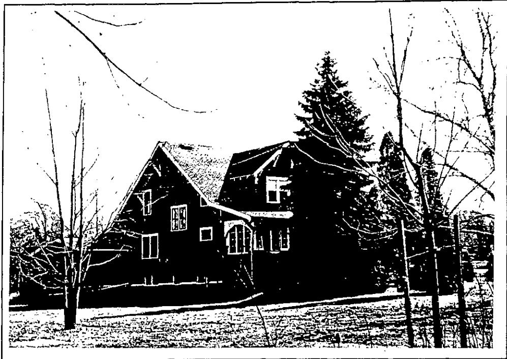
4655 Harlem Road. North and west elevations.
