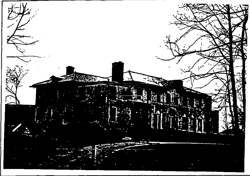
Crouch-Waite Mansion (Rosary Hall), Daemen College Campus. East and north elevations.
