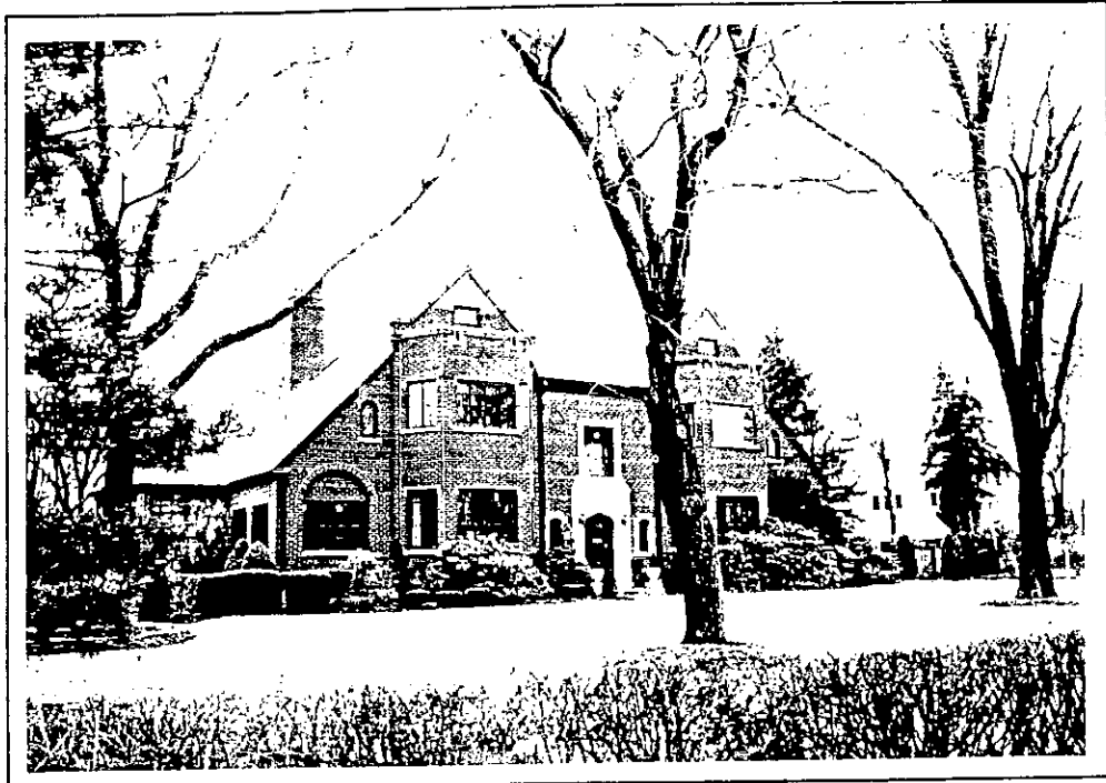
655 LeBrun Rd. North and west elevations.
