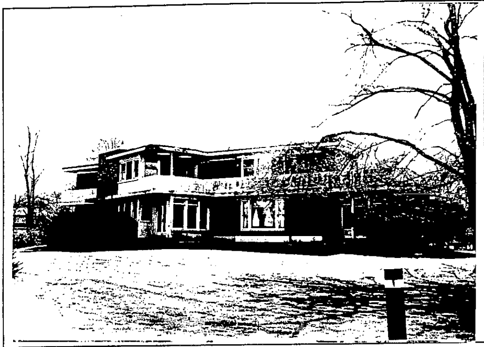
895 North Forest Rd. West and south elevations.
