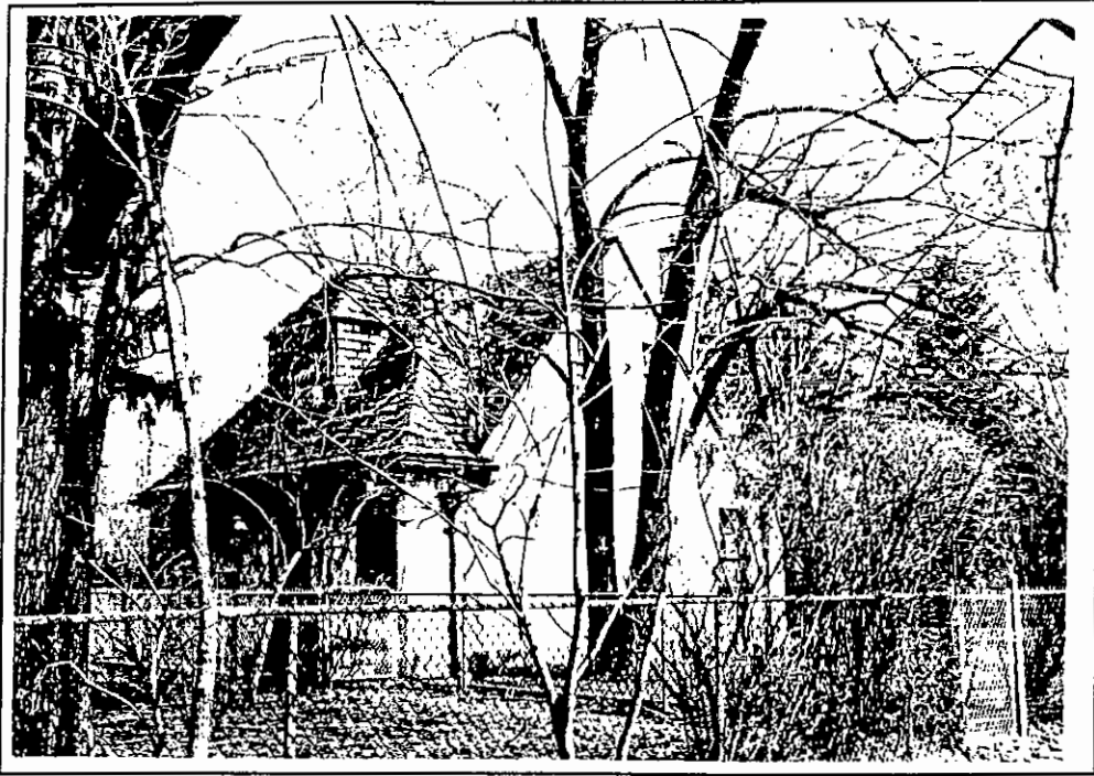
Garage at 697 LeBrun Rd. West and south elevations.
