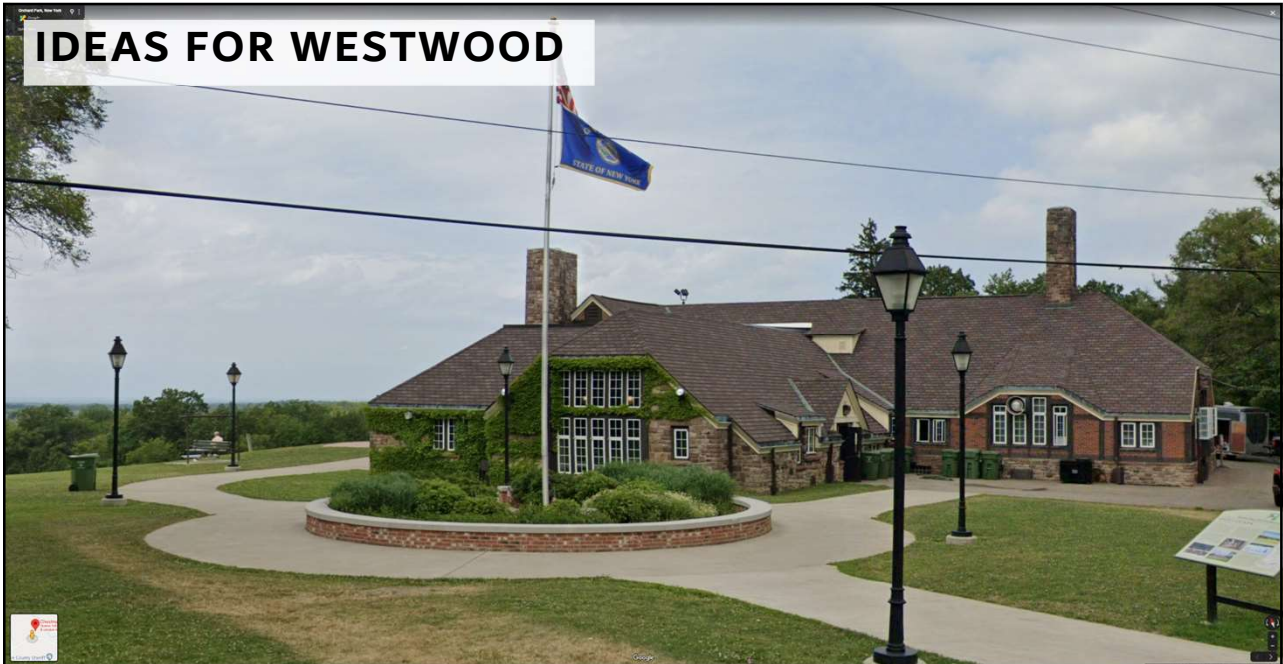
CHARACTER OF WPA ERA PARK BUILDINGS: CONTINUE THAT TRADITION?
