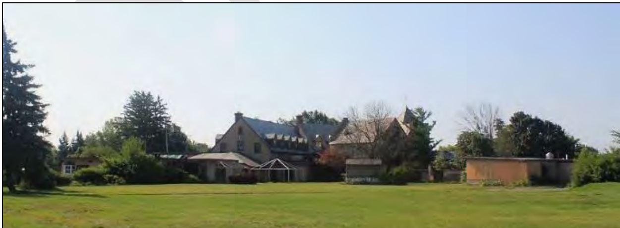
The former Westwood Clubhouse provides reuse opportunities possibly as a Town Arts and Cultural Center.
