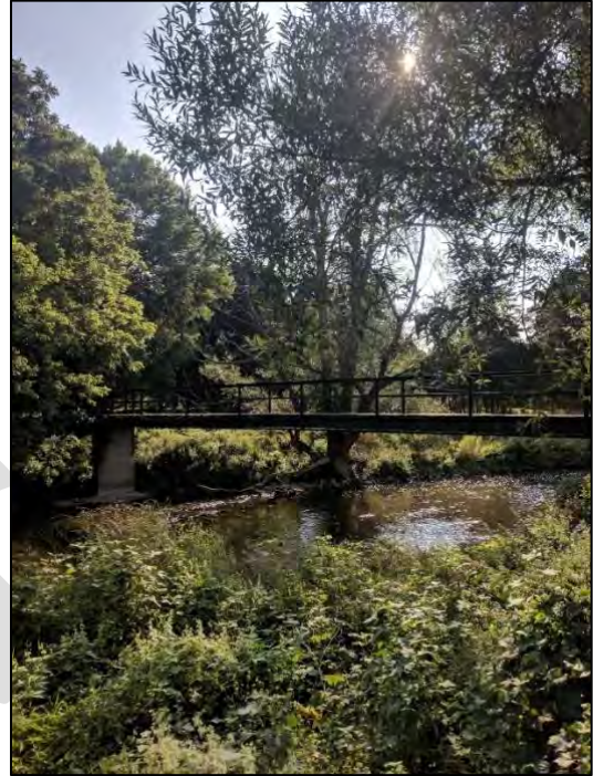
The existing Westwood pedestrian bridge over Ellicott Creek
