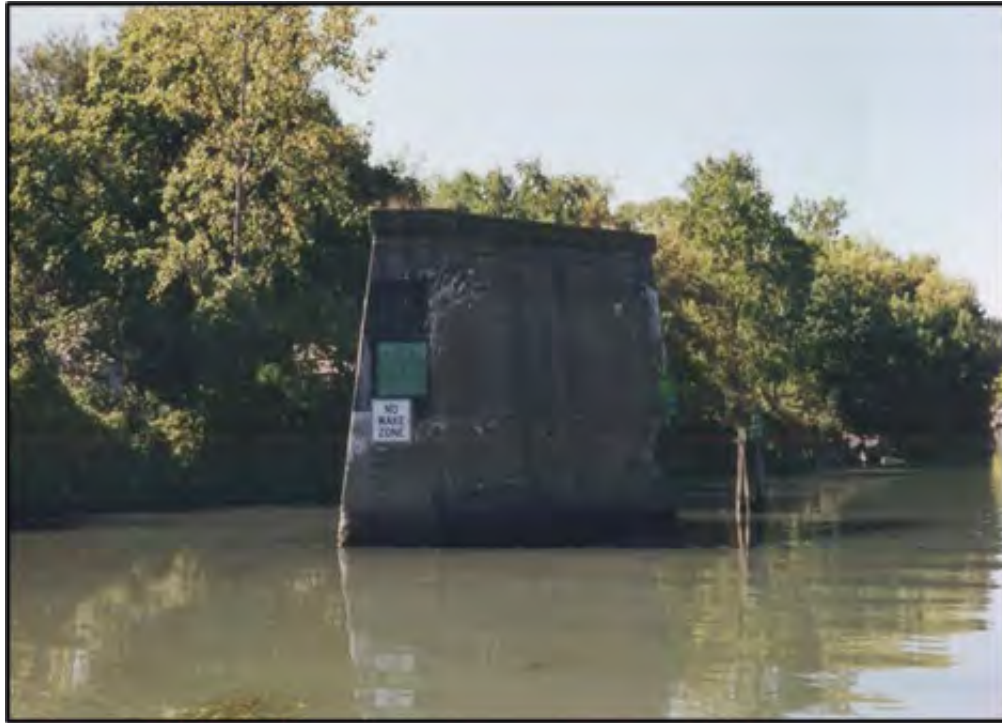
Source: Old Bridge Abutment. Town Staff Photo Taken 2002.
