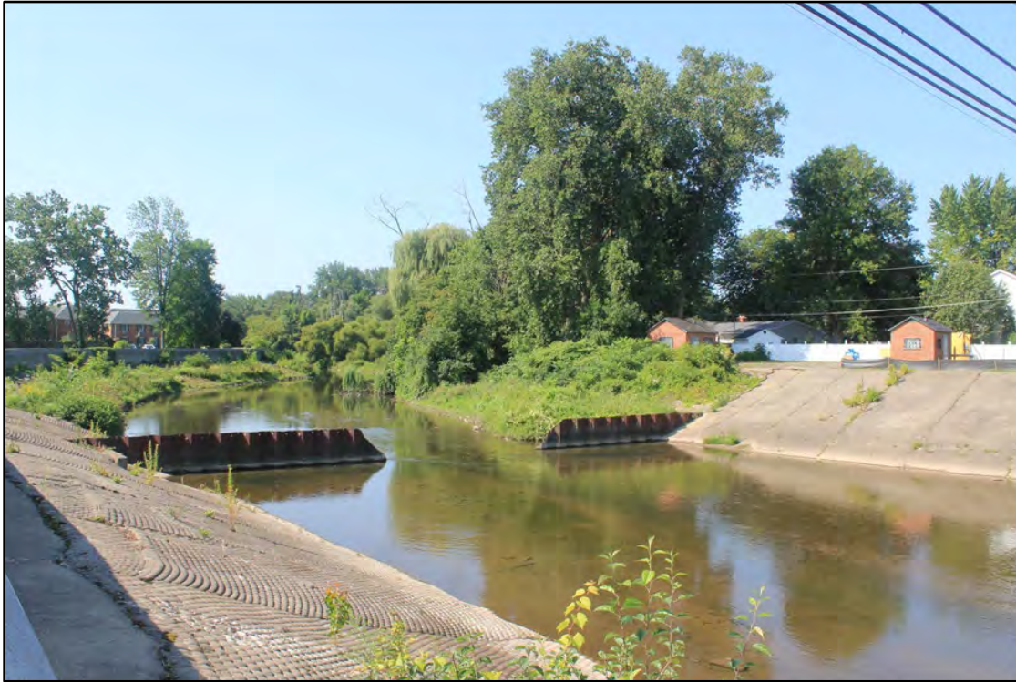
Figure 2.38 - USACE Channelized Creek at Bottom of Channel 579.0' Elevation, south of Maple St.
