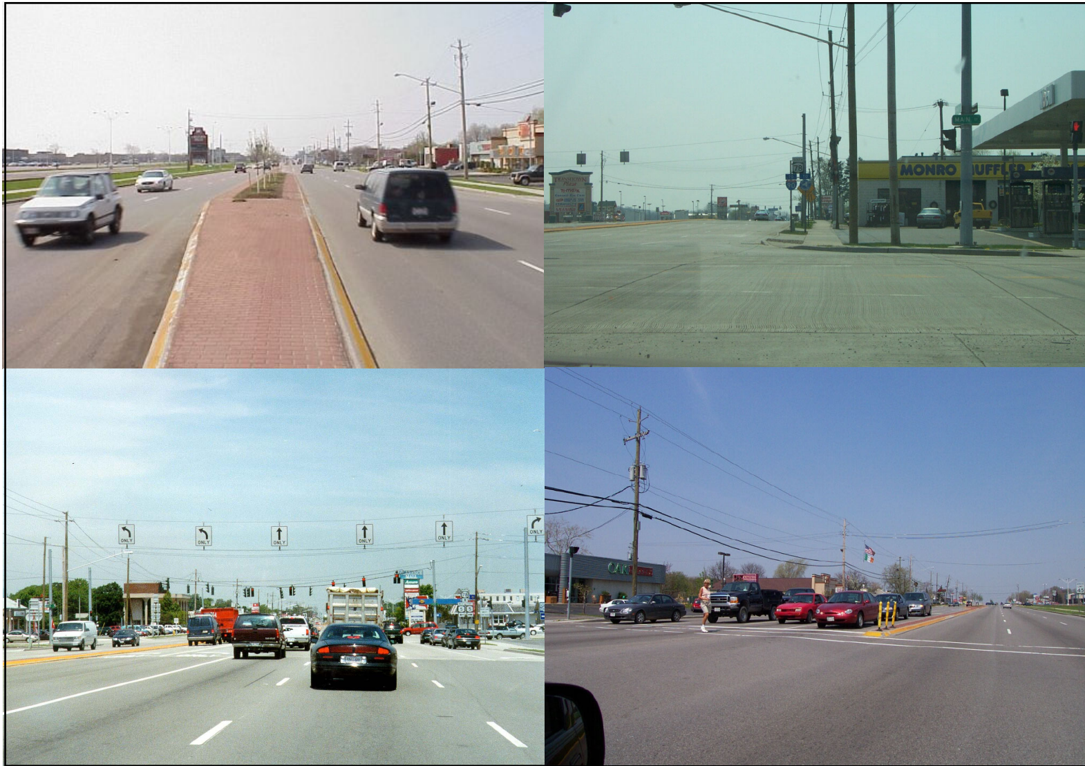
Figure III-29: These pictures illustrate the existing cross sections within Focus Area IV. The typical cross section is sidewalk, planting strip, right turn lane, three through travel lanes in each direction with a raised, landscaped median.
