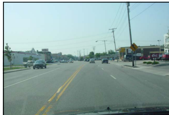
Commercial development and driveways along Bailey Avenue (between Eggert Rd. and Sheridan Dr.)
