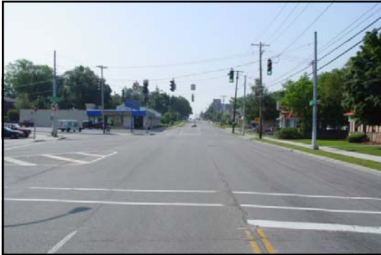
Consideration of driveway consolidation is needed within the functional area of intersections. (Bailey and Grover Cleveland)
