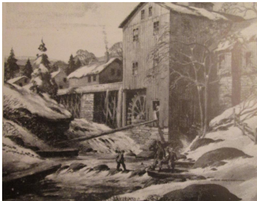
Figure 5: The Williamsville Water Mill was constructed in 1811 by Jonas Williams. This illustration shows the raceway that brought the water from Ellicott Creek to turn the large waterwheel in the 1850s. Courtesy Amherst Museum/from Glancing Back: A Pictorial History of Amherst, New York by Joseph A. Grande [page 17].
