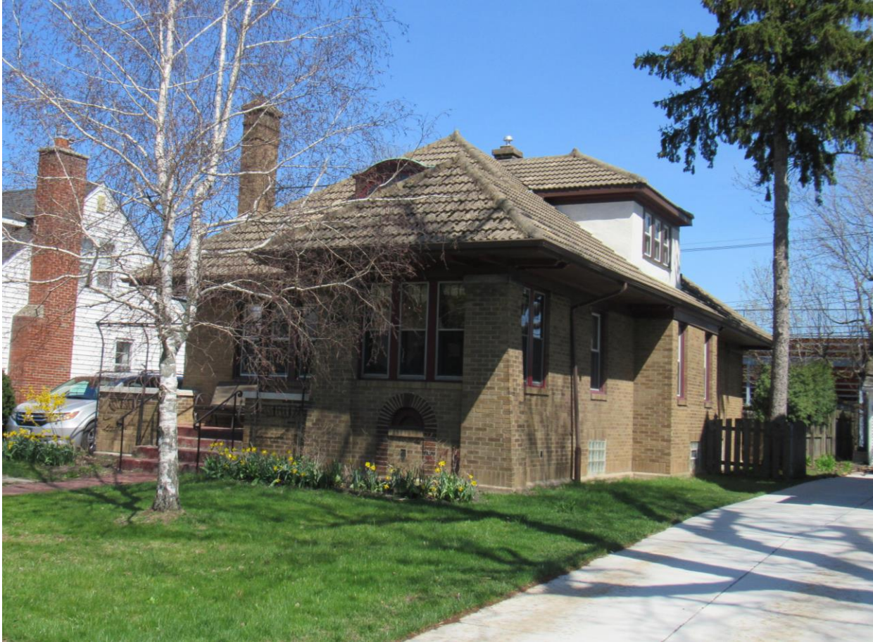
NY_Erie County_Town of Amherst_130 Berryman Drive_South and West Elevations
