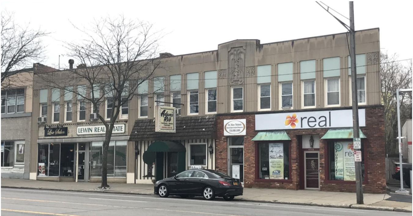
NY_Erie County_Town of Amherst_4511-4521 Main Street_North and West Elevations
