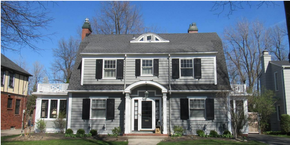
NY_Erie County_ Town of Amherst _90 Darwin Drive_ West Elevation
