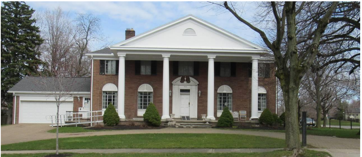
NY_Erie County_ Town of Amherst _3736 Main Street_South Elevation
