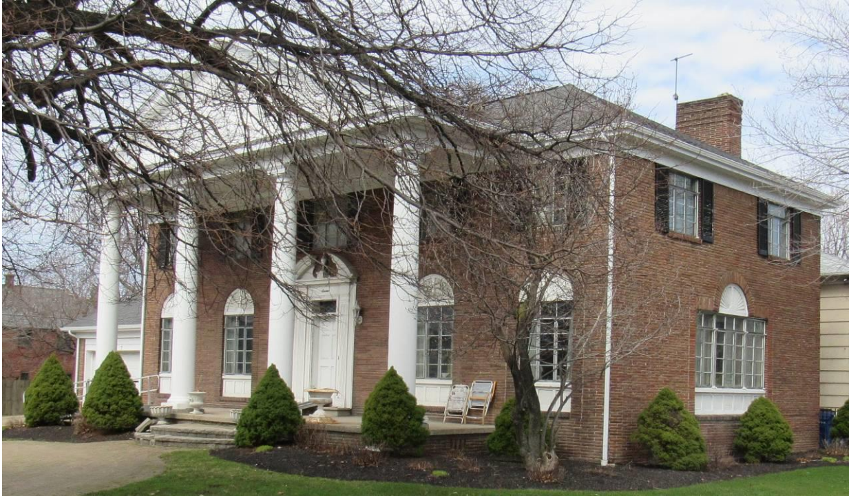
NY_Erie County_ Town of Amherst _3736 Main Street_South and East Elevations
