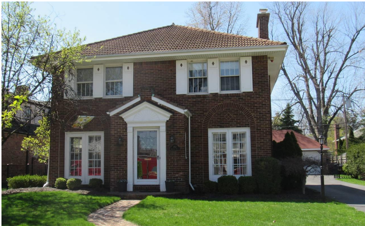
NY_Erie County_ Town of Amherst _253 Berryman Drive_East Elevation
