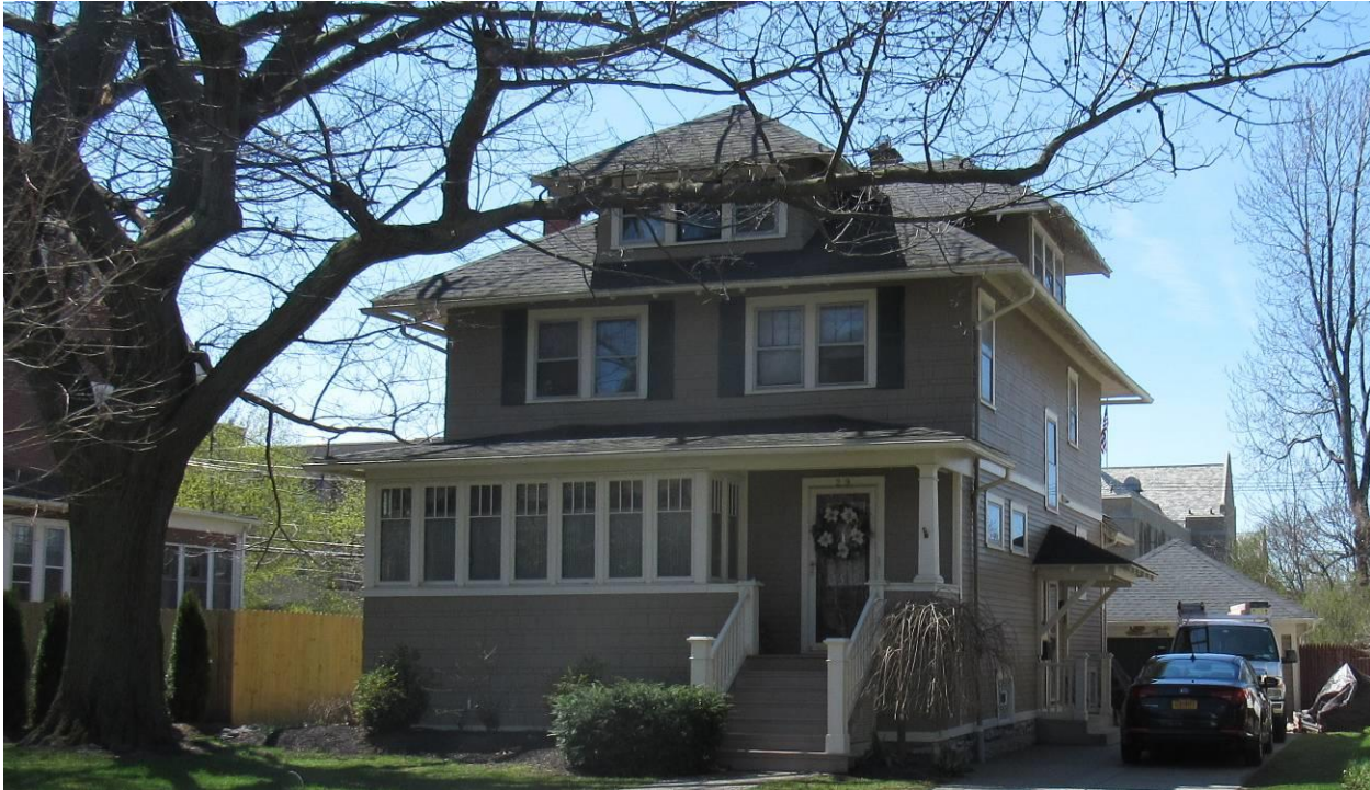
NY_Erie County_ Town of Amherst _29 Washington Highway_ North and East Elevations
