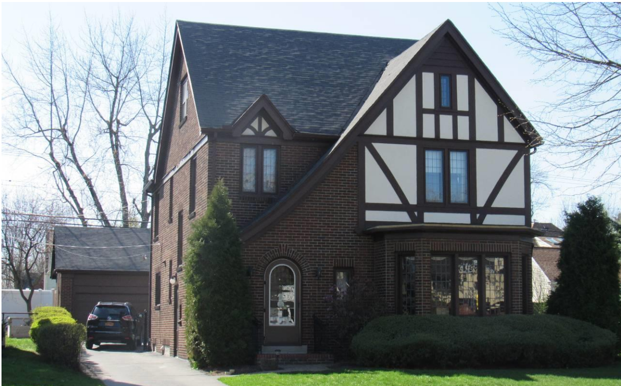
NY_Erie County_ Town of Amherst _93 Darwin Drive_South and East Elevations
