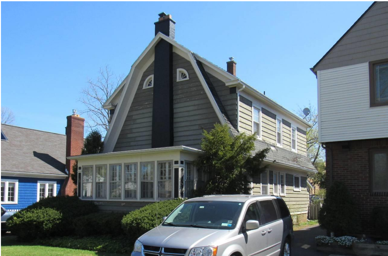
NY_Erie County_ Town of Amherst _48 Berryman Drive_ South and West Elevations
