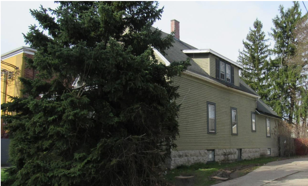
NY_Erie County_ Town of Amherst _26 Callodine Avenue_North and East Elevations
