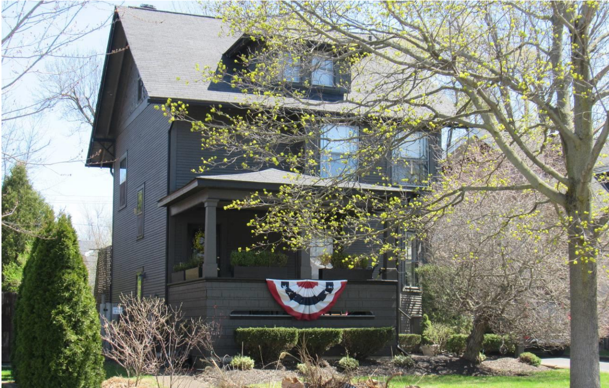
NY_Erie County_ Town of Amherst _278 Washington Highway_North and West Elevations
