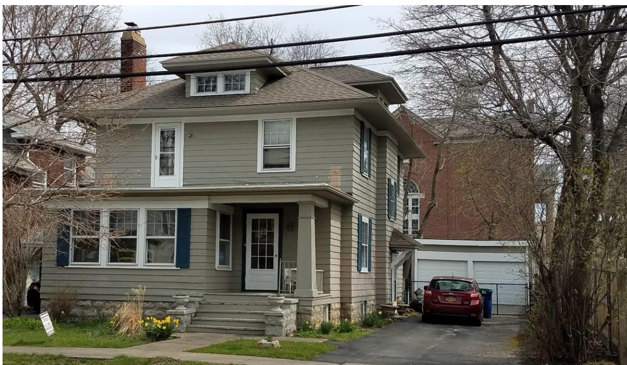
NY_Erie County_ Town of Amherst _17 Maynard Drive_South and West Elevations
