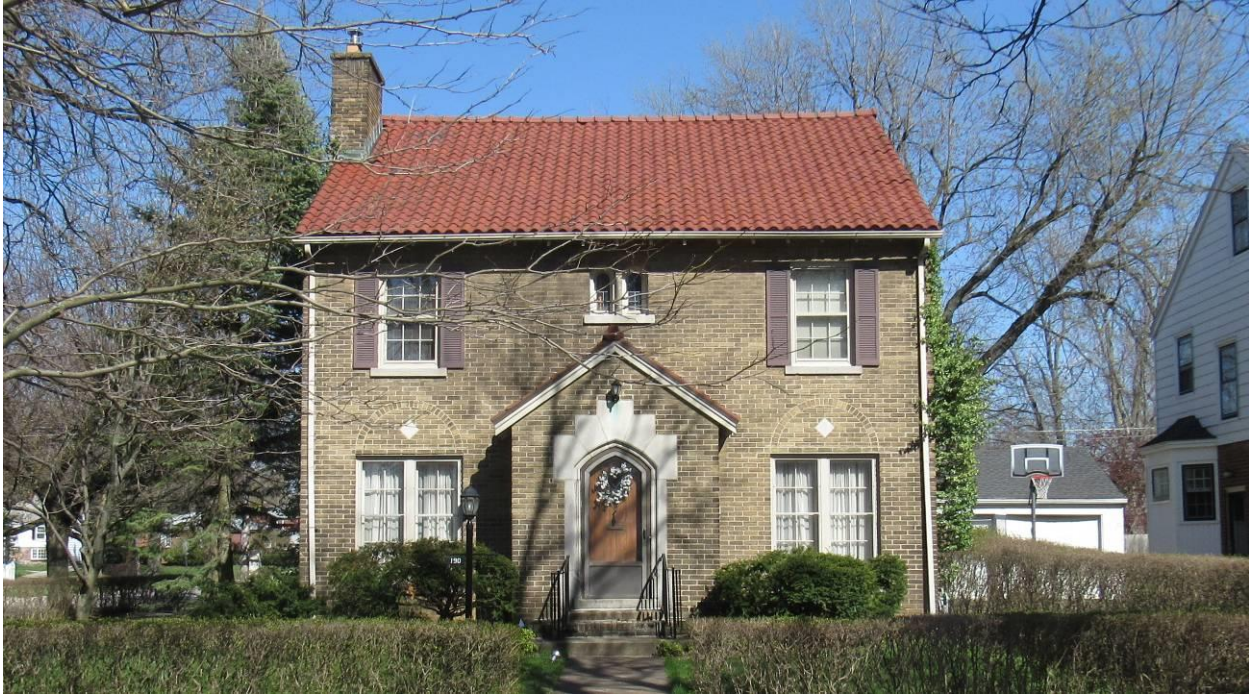
NY_Erie County_ Town of Amherst _190 Darwin Drive_ West Elevation
