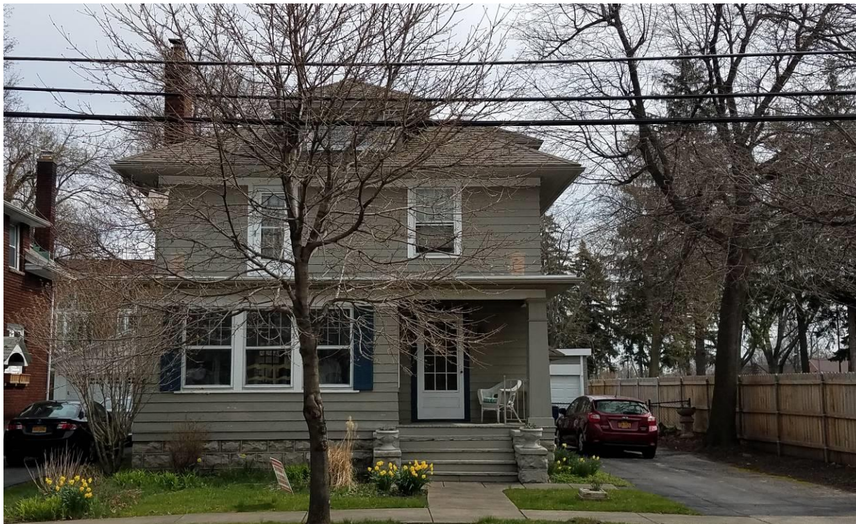
NY_Erie County_ Town of Amherst _17 Maynard Drive_West Elevation
