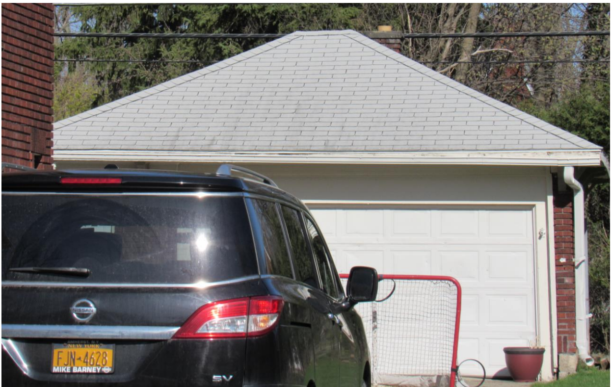
NY_Erie County_ Town of Amherst _38 Roycroft Boulevard_Detached Garage
