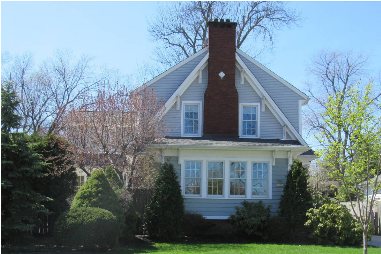
NY_Erie County_ Town of Amherst _339 Berryman Drive_East Elevation
