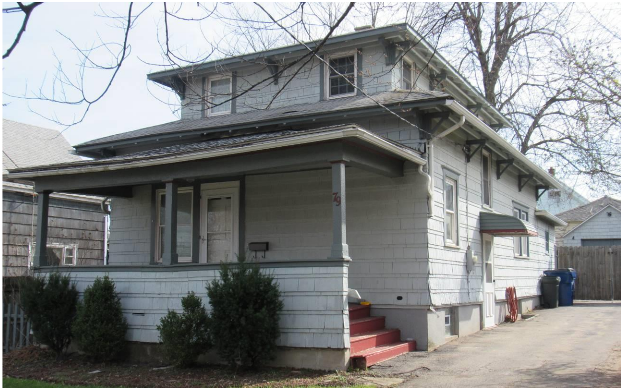
NY_Erie County_ Town of Amherst _79 Callodine Avenue_South and West Elevations
