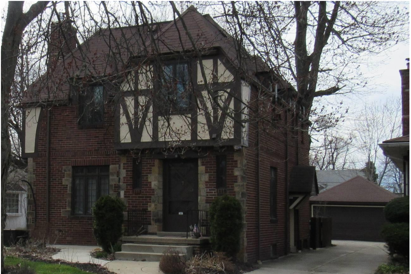
NY_Erie County_ Town of Amherst _8 Hendricks Boulevard_North and West Elevations
