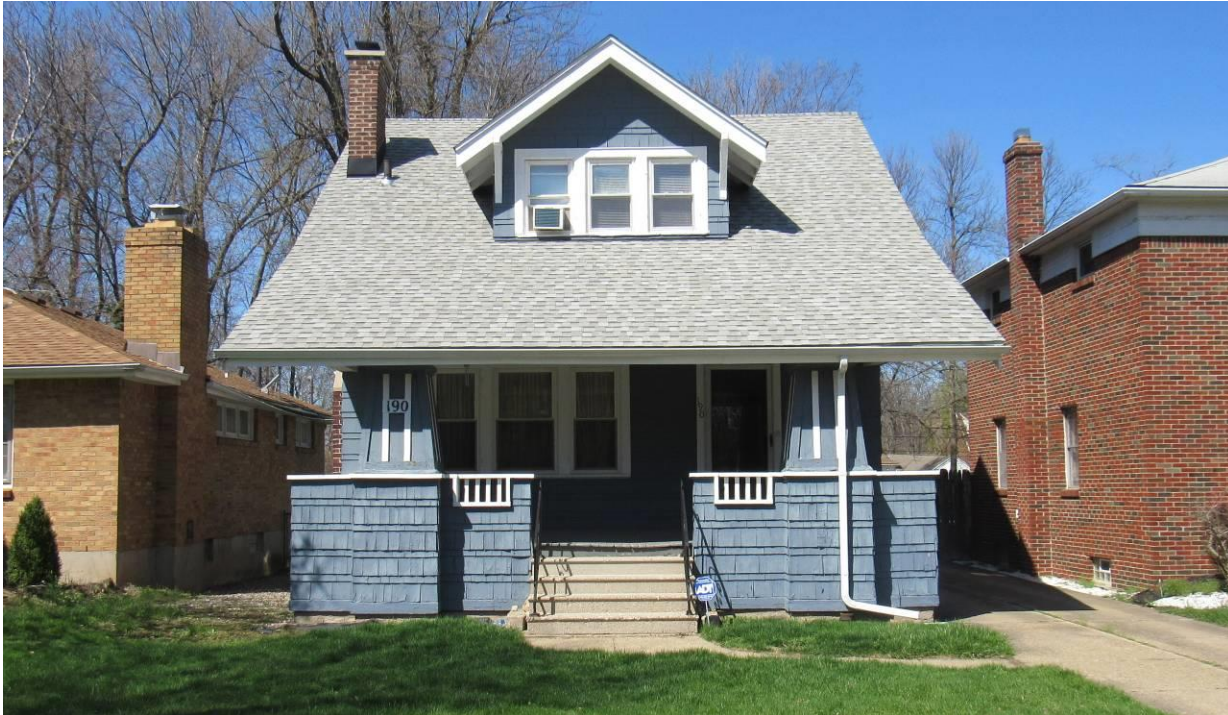
NY_Erie County_ Town of Amherst _190 Kings Highway_South Elevation
