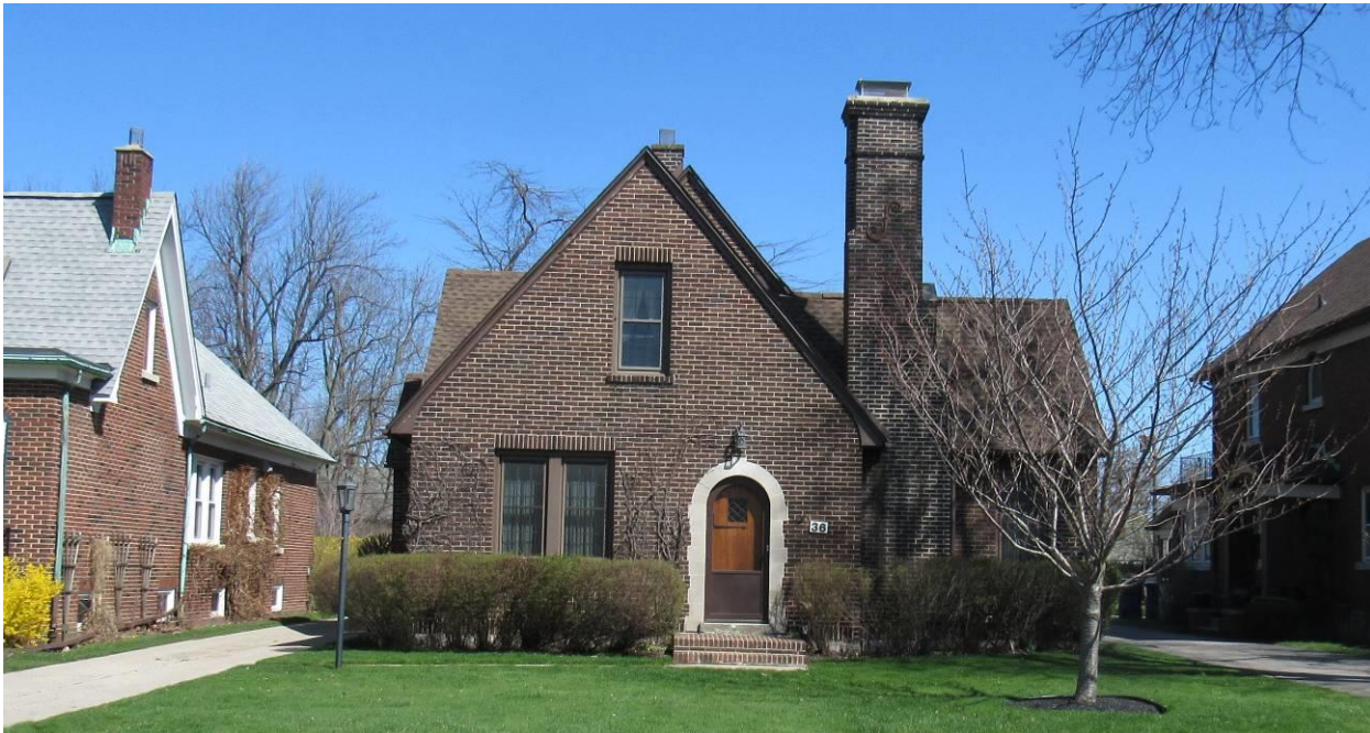
NY_Erie County_ Town of Amherst _36 South Drive_South Elevation
