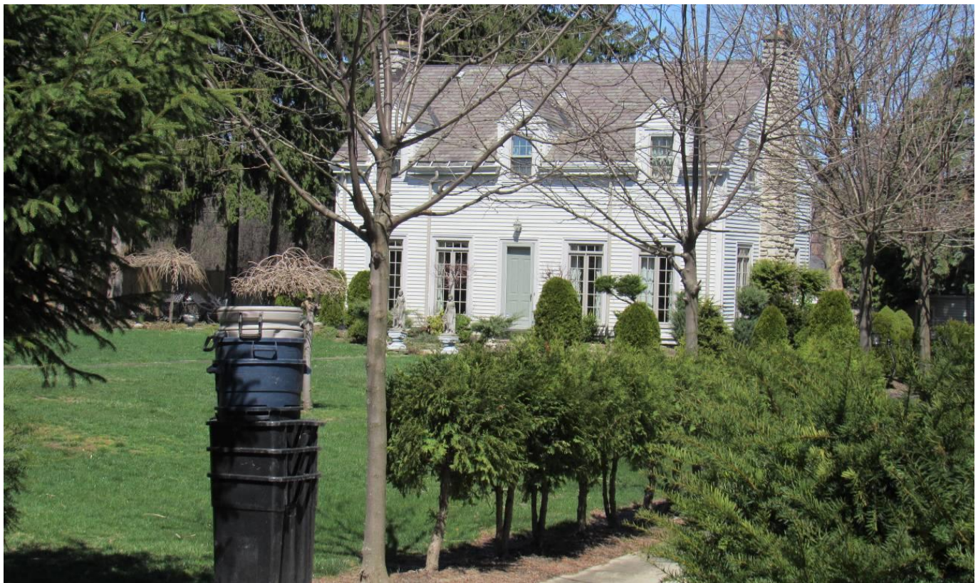
NY_Erie County_ Town of Amherst_24 Lyman Road_South and East Elevations
