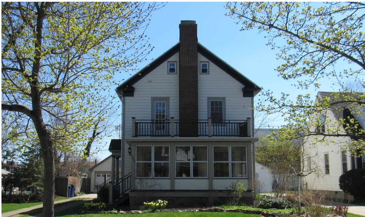
NY_Erie County_ Town of Amherst _120 Berryman Drive_West Elevation
