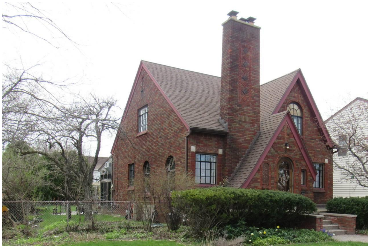
NY_Erie County_ Town of Amherst _38 Endicott Drive_ Northeast and Southeast Elevations
