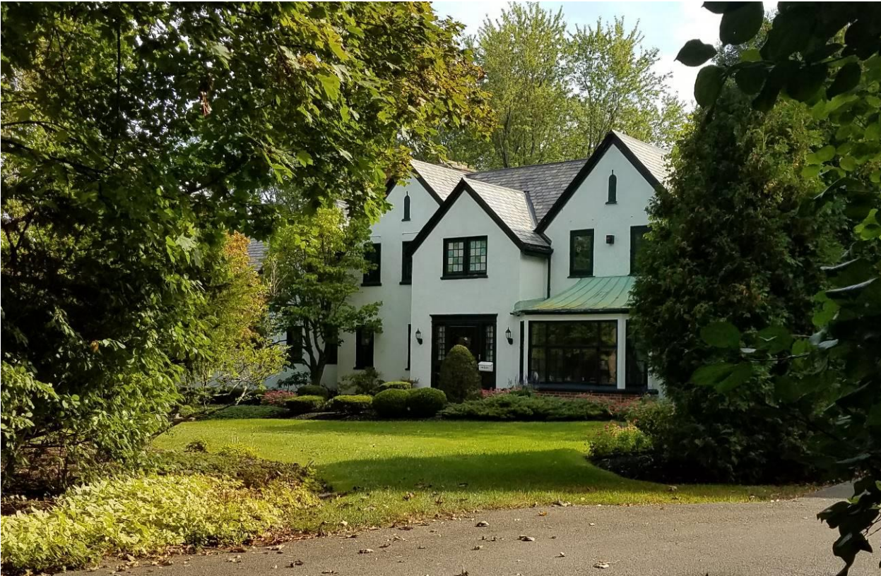
NY_Erie County_ Town of Amherst _50 Lyman Road_ West Elevations
