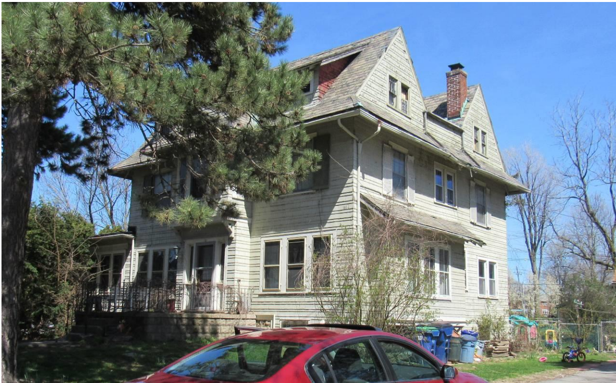
NY_Erie County_ Town of Amherst _6 Washington Highway_ South and West Elevations
