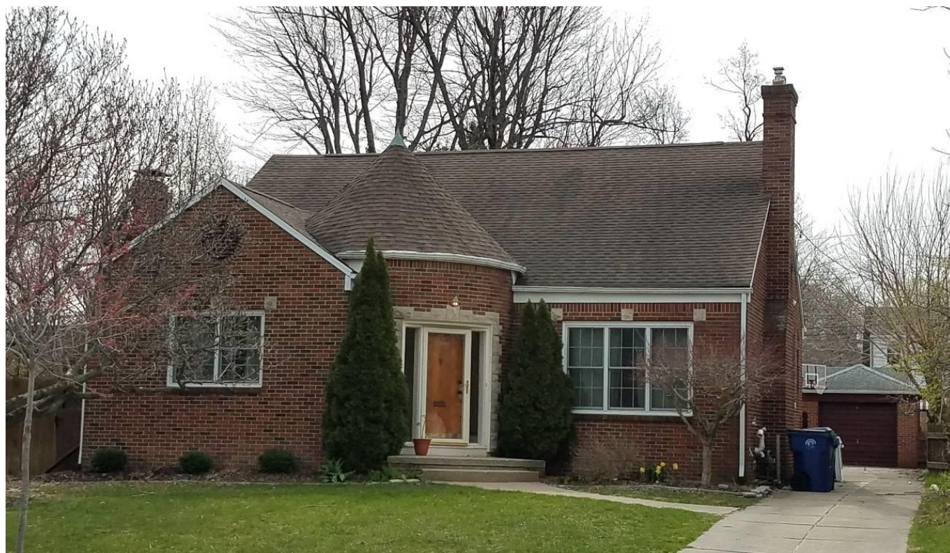
NY_Erie County_ Town of Amherst _127 Crosby Boulevard_ Northwest and Southwest Elevations
