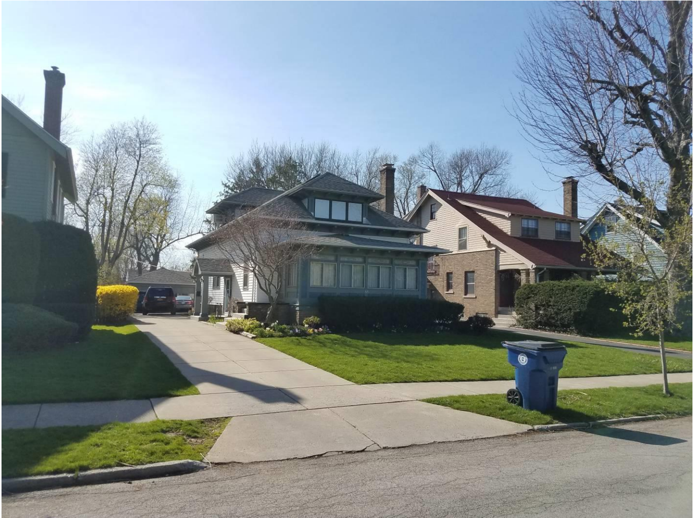
NY_Erie County_ Town of Amherst _55 Roycroft Boulevard_South and East Elevations
