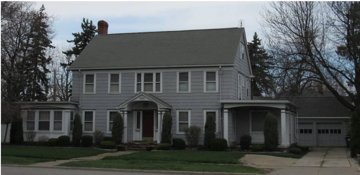
NY_Erie County_ Town of Amherst _3690 Main Street_South and East Elevations
