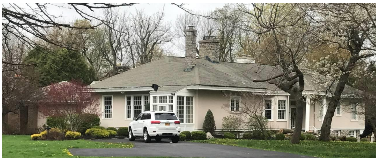
NY_Erie County_ Town of Amherst _300 Brompton Road_North and East Elevations
