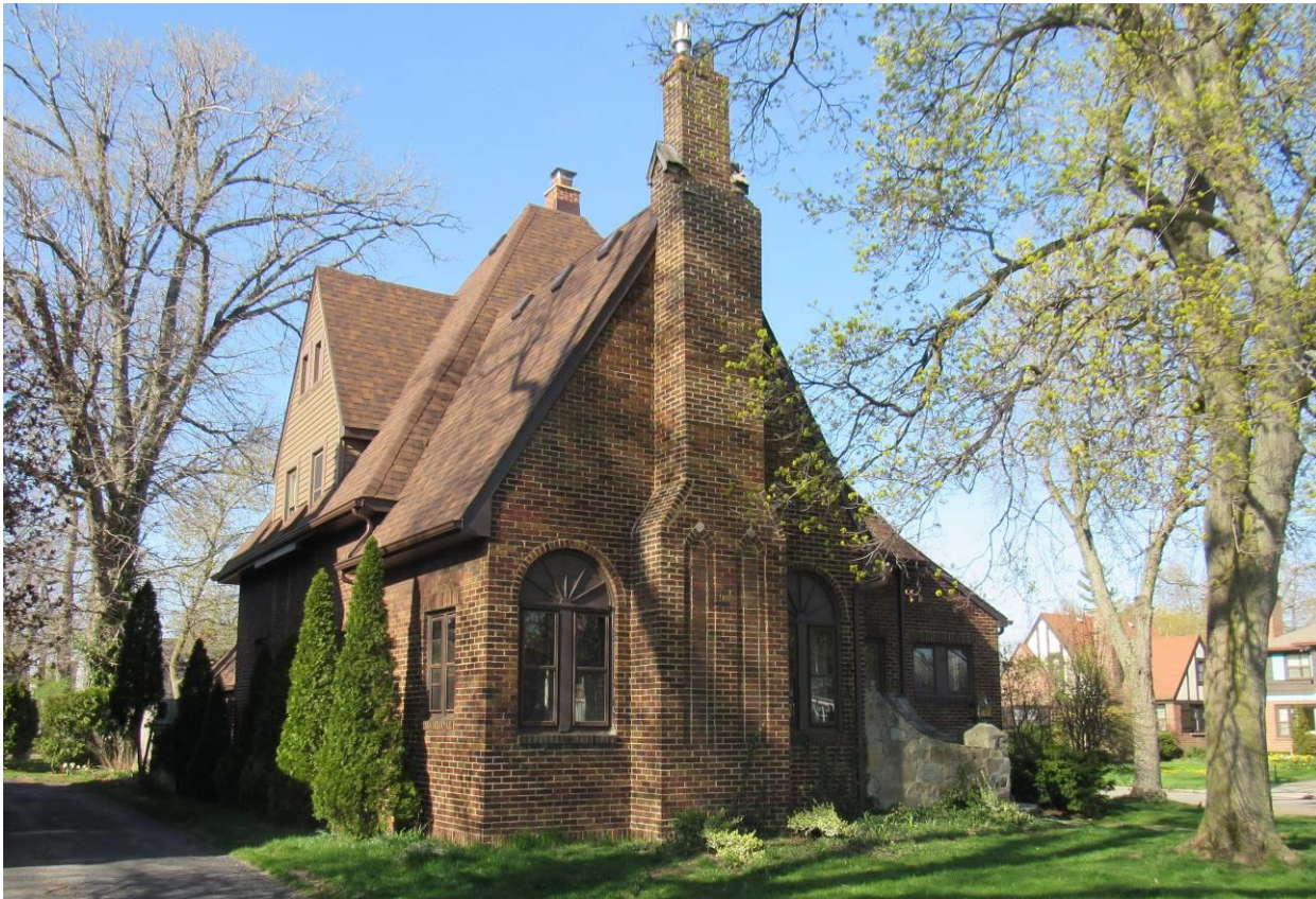
NY_Erie County_ Town of Amherst _114 Saratoga Road_South and East Elevations
