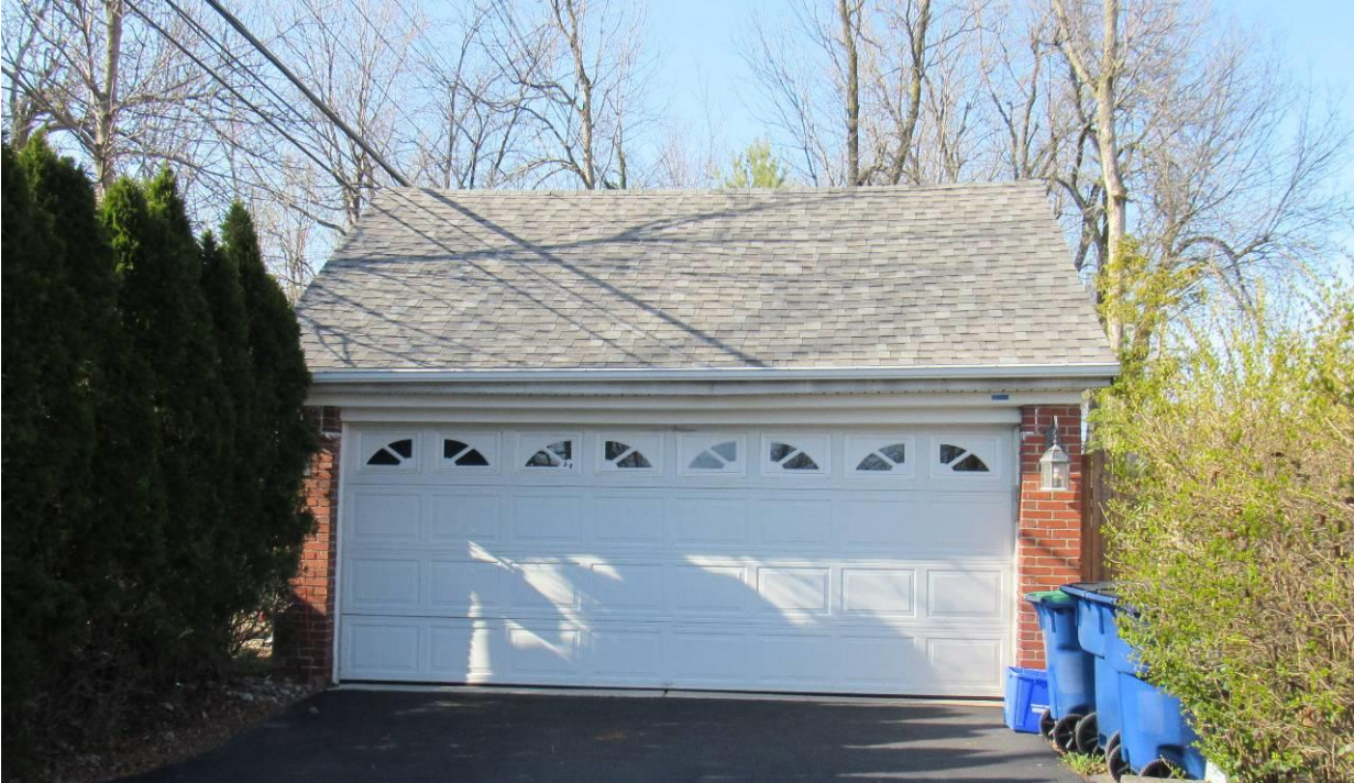
NY_Erie County_ Town of Amherst _460 Saratoga Road_Detached Garage
