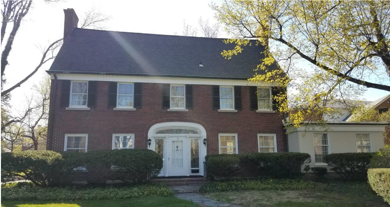
NY_Erie County_ Town of Amherst _5 Darwin Drive_East Elevation
