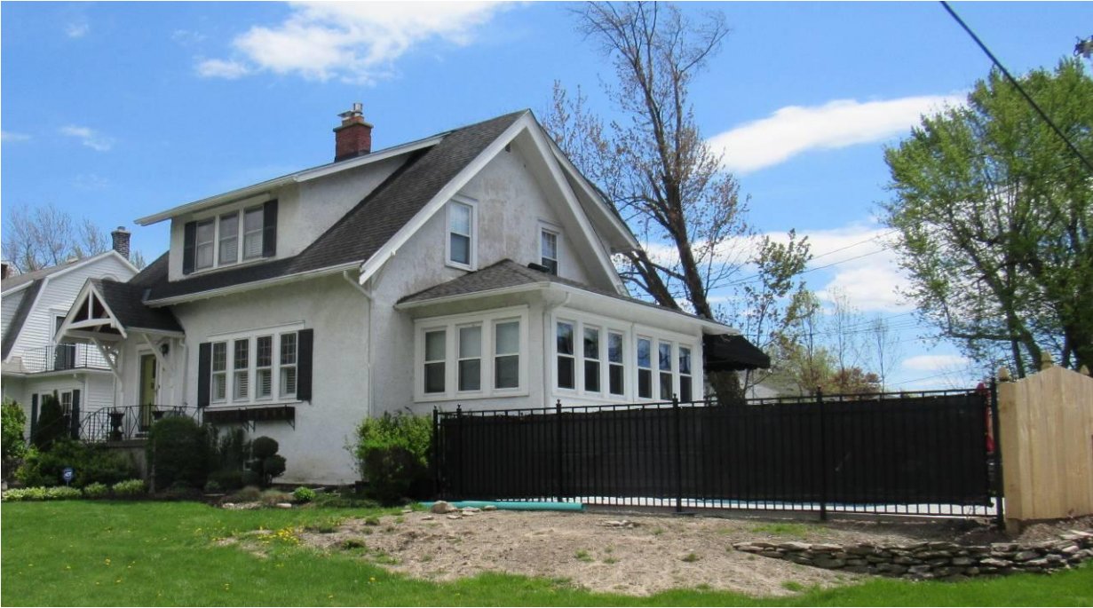
NY_Erie County_ Town of Amherst _151 Kings Highway_North and East Elevations
