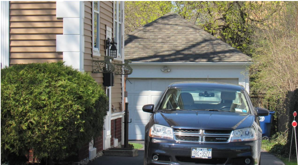
NY_Erie County_ Town of Amherst _79 Berryman Drive_North and East Elevations_Detached Garage
