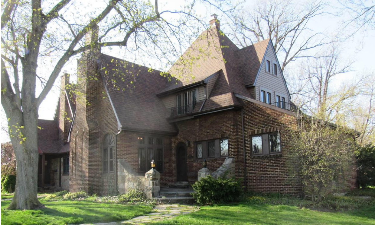
NY_Erie County_ Town of Amherst _114 Saratoga Road_North and East Elevations
