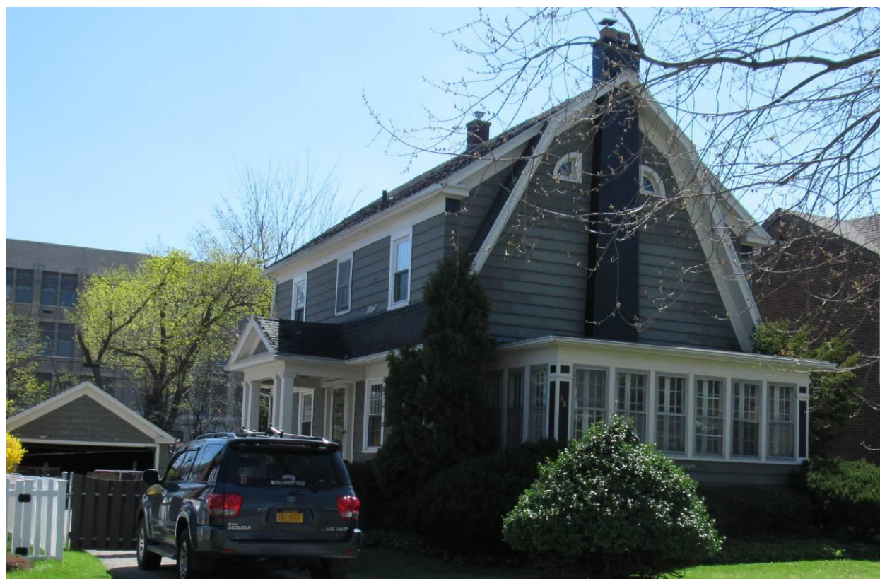
NY_Erie County_Town of Amherst_48 Berryman Drive_North and West Elevations
