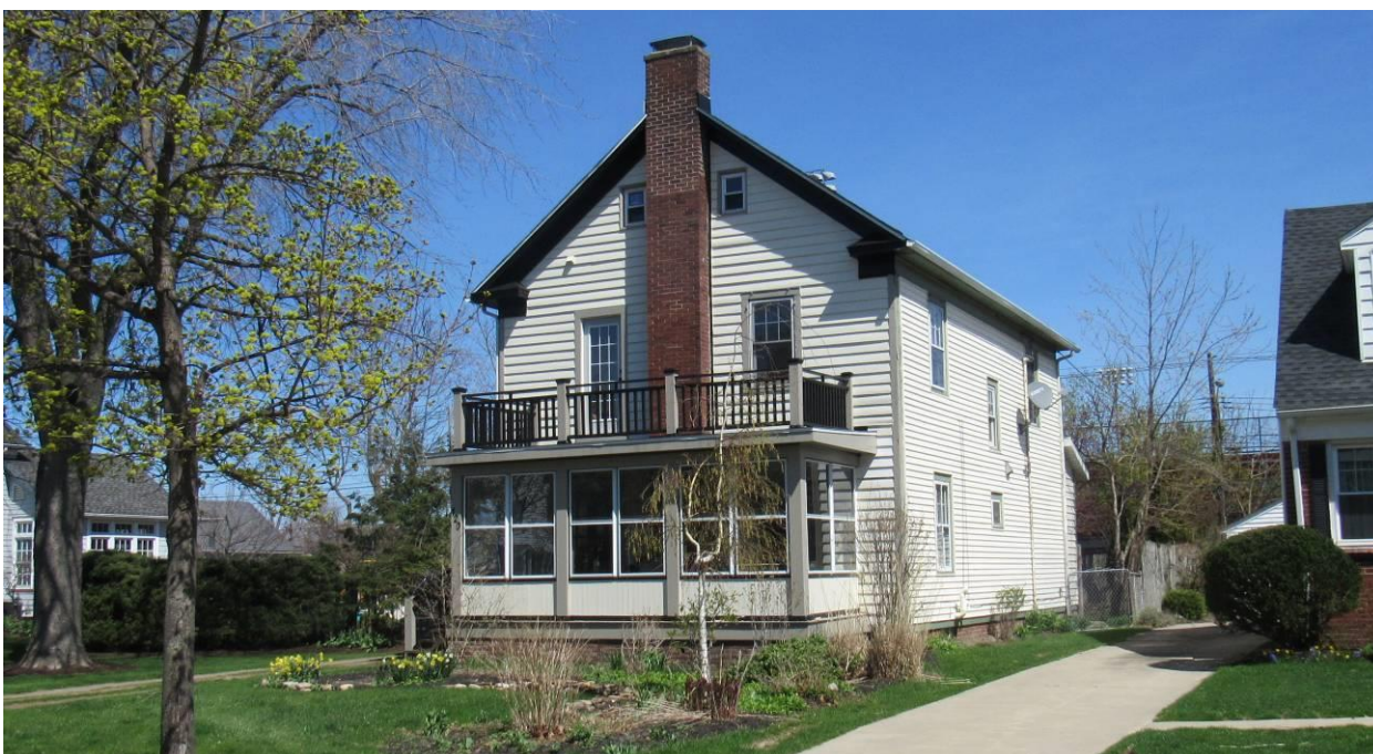
NY_Erie County_ Town of Amherst _120 Berryman Drive_South and West Elevations
