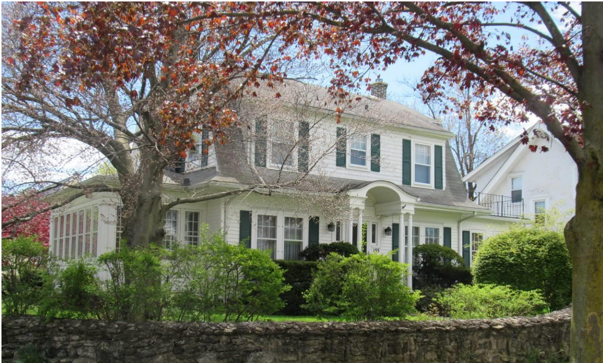
NY_Erie County_ Town of Amherst _155 Kings Highway_ North and East Elevations
