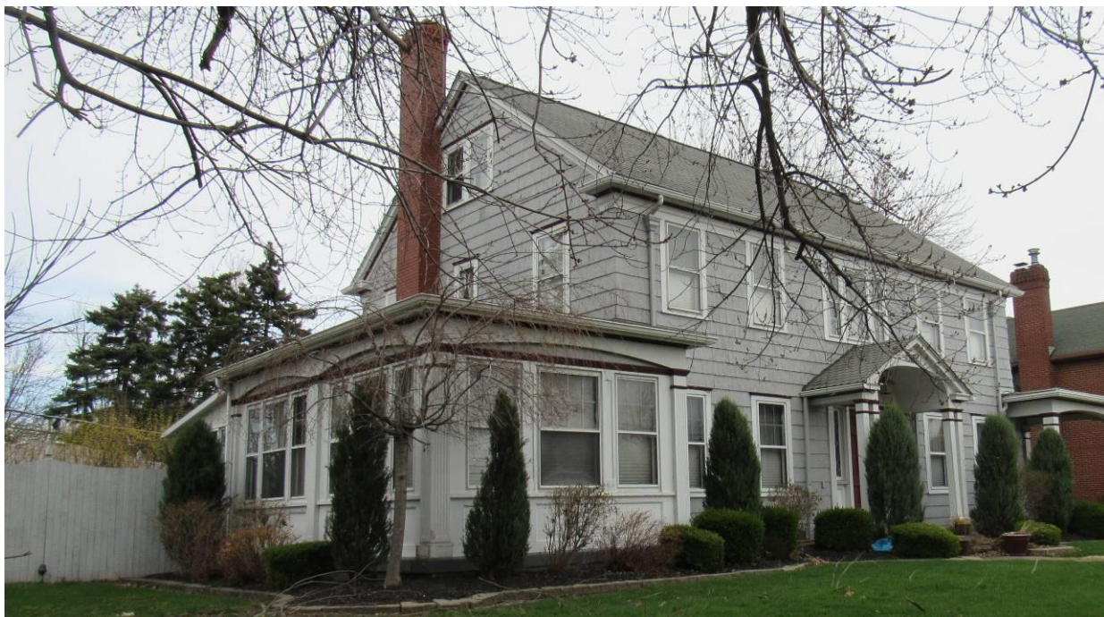
NY_Erie County_ Town of Amherst_3690 Main Street_South and West Elevations
