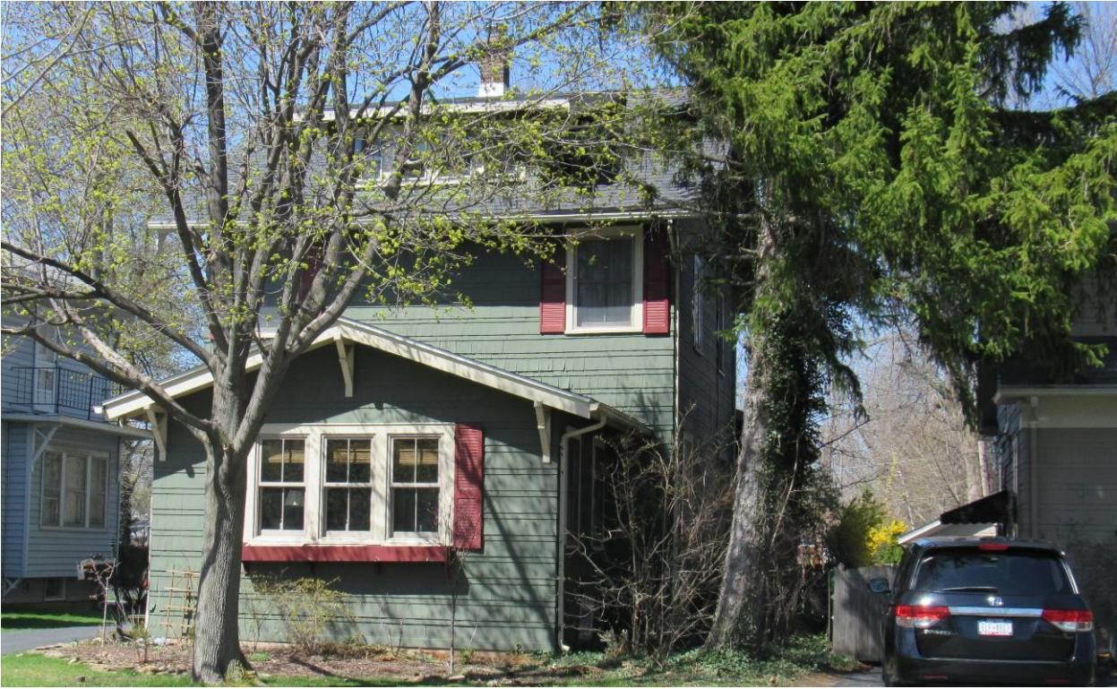
NY_Erie County_ Town of Amherst _178 Kings Highway_South and East Elevations
