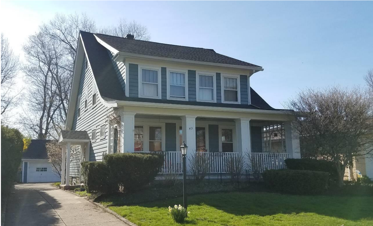
NY_Erie County_ Town of Amherst _45 Roycroft Boulevard_South and East Elevations
