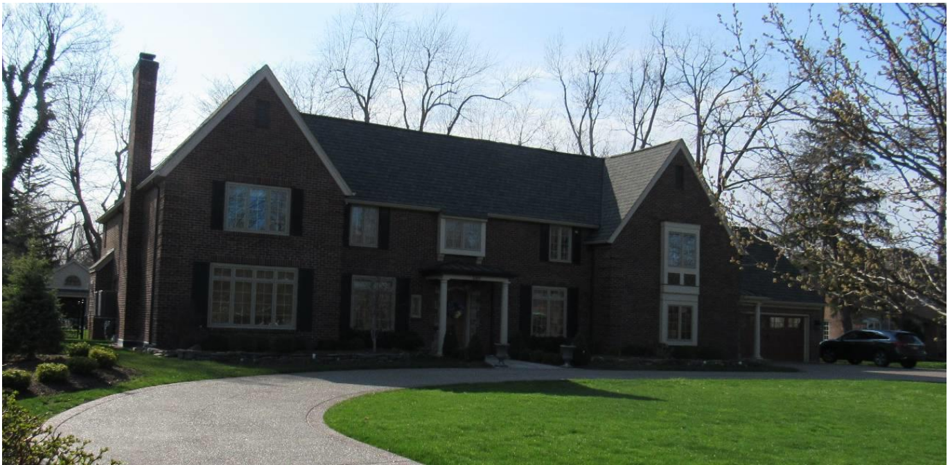
NY_Erie County_ Town of Amherst _880 Le Brun Road_South and East Elevation
