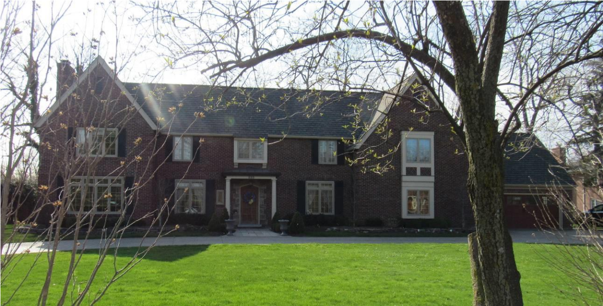
NY_Erie County_ Town of Amherst _880 Le Brun Road_East Elevation
