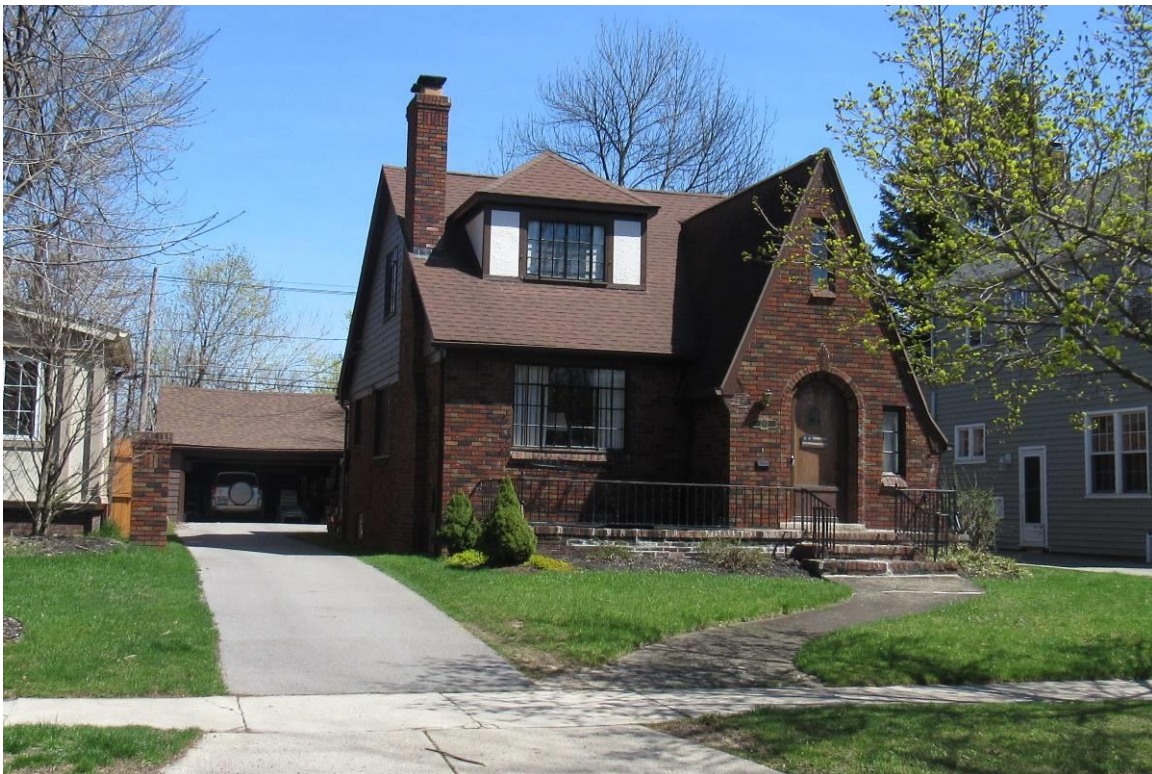
NY_Erie County_ Town of Amherst _212 Berryman Drive_North and West Elevations
