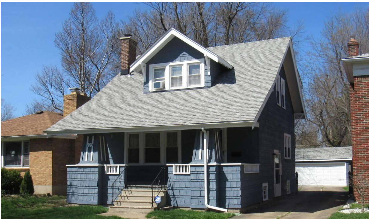
NY_Erie County_ Town of Amherst _190 Kings Highway_South and East Elevations
