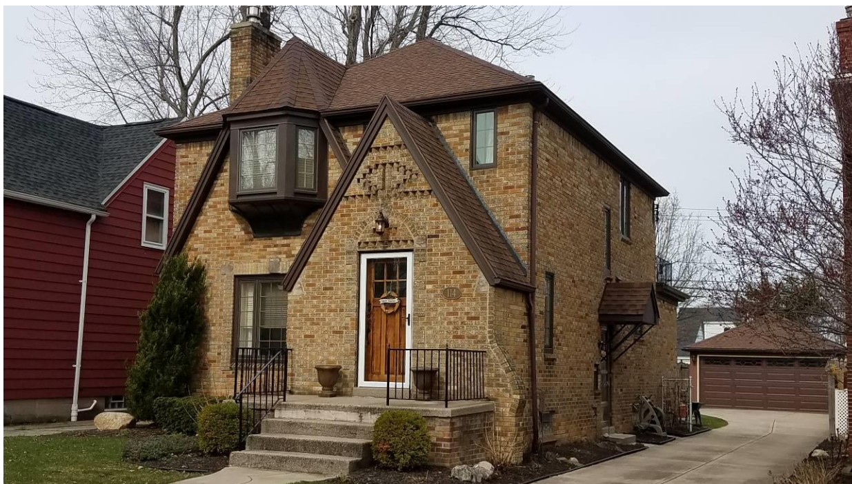
NY_Erie County_ Town of Amherst _114 Hendricks Boulevard_North and West Elevations
