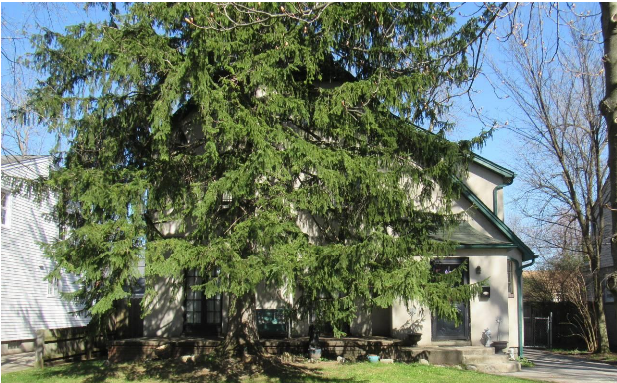
NY_Erie County_ Town of Amherst _244 Roycroft Boulevard_ West Elevation
