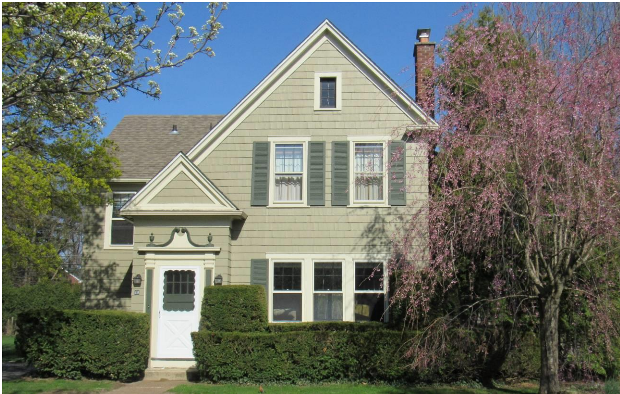
NY_Erie County_ Town of Amherst _48 Roycroft Boulevard_ West Elevation
