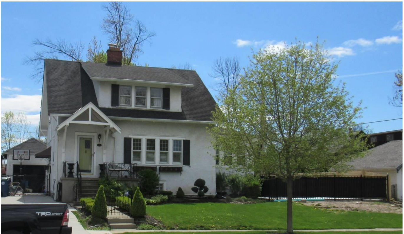
NY_Erie County_ Town of Amherst _151 Kings Highway_North Elevation
