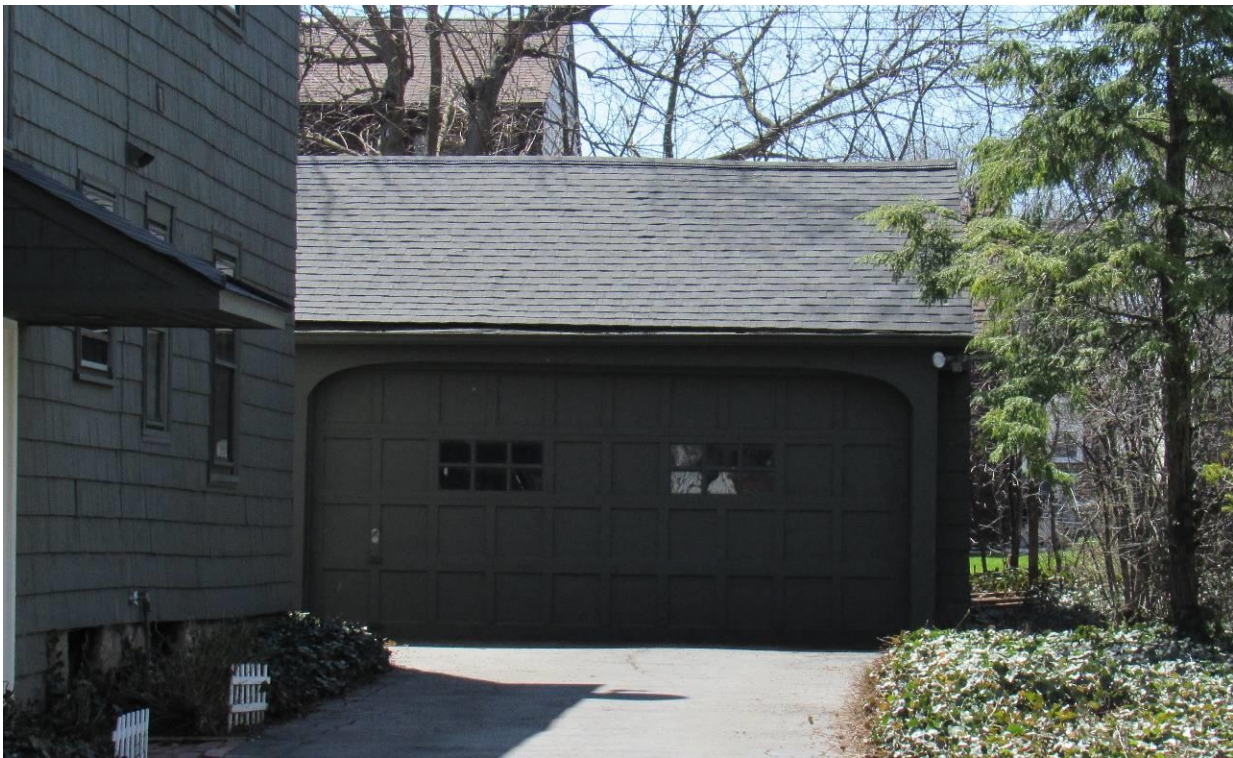
_Erie County_ Town of Amherst _31 Cornell Ave_ Detached Garage
