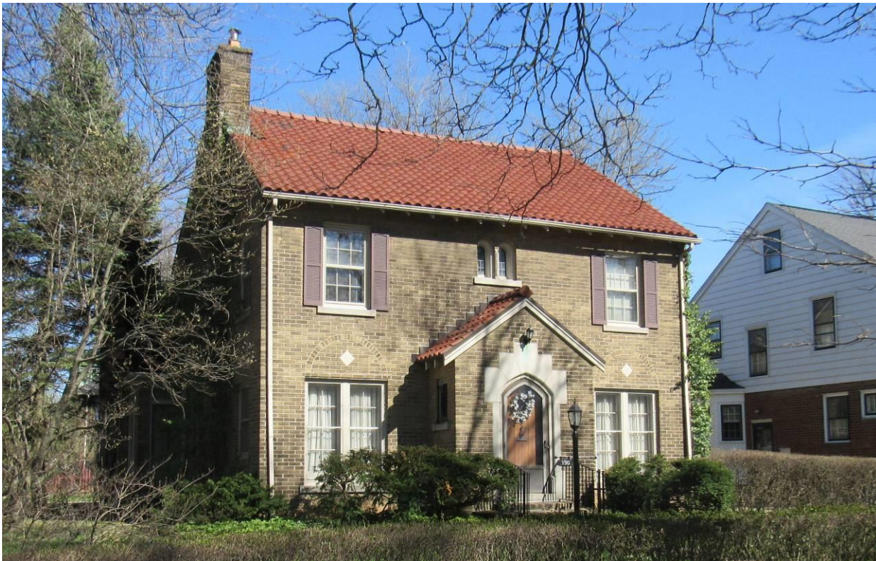
NY_Erie County_ Town of Amherst _190 Darwin Drive_North and West Elevations
