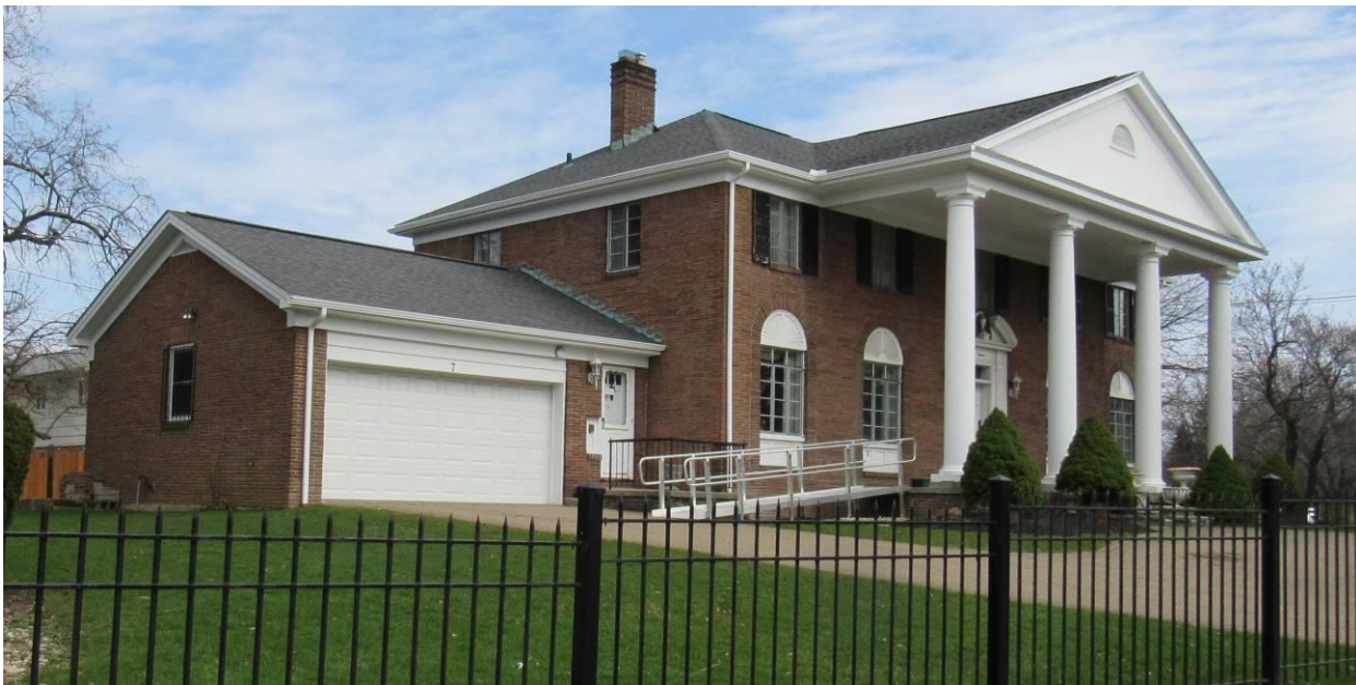
NY_Erie County_ Town of Amherst _3736 Main Street_South and West Elevations
