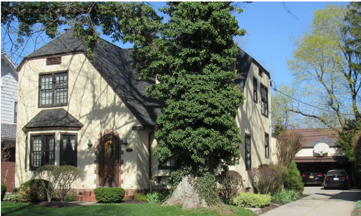
NY_Erie County_ Town of Amherst _144 Darwin Drive_ South and West Elevations
