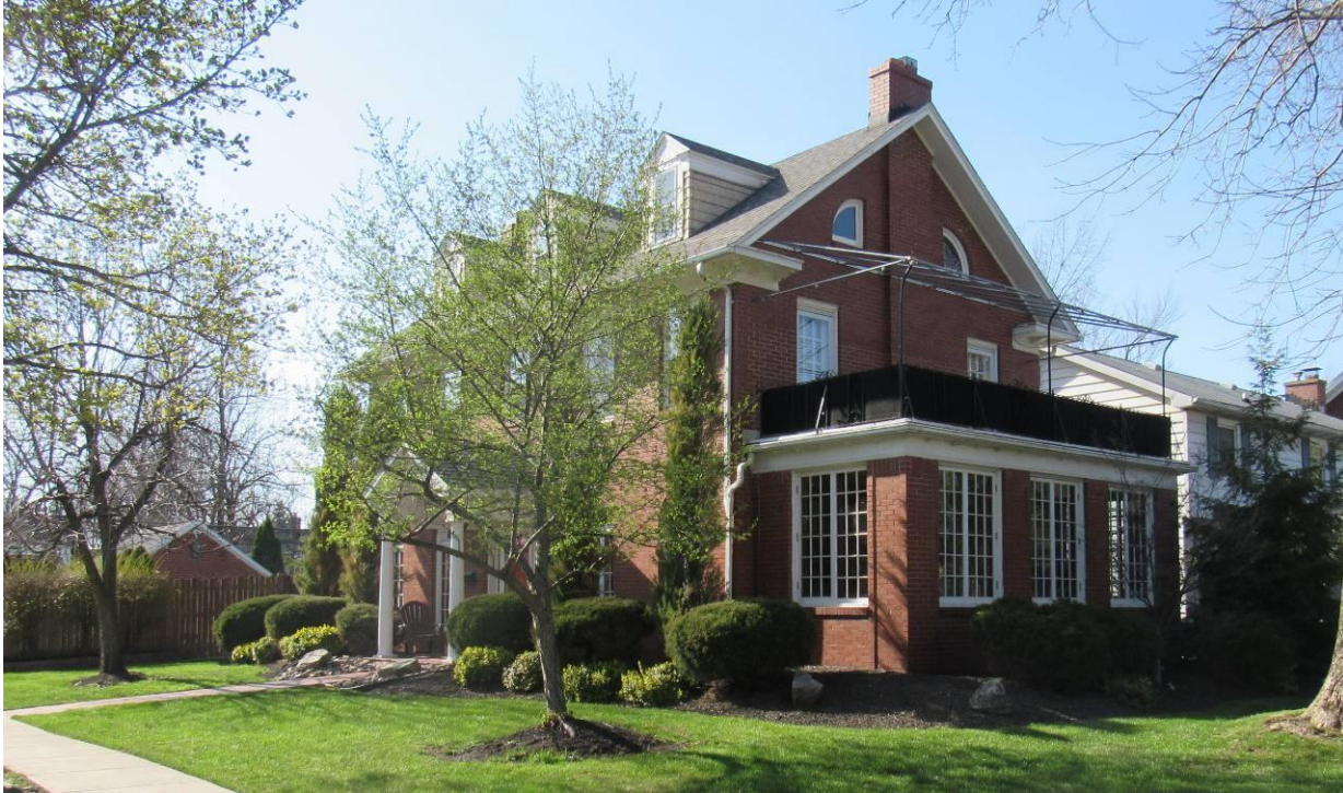
NY_Erie County_ Town of Amherst _460 Saratoga Road_South and East Elevations
