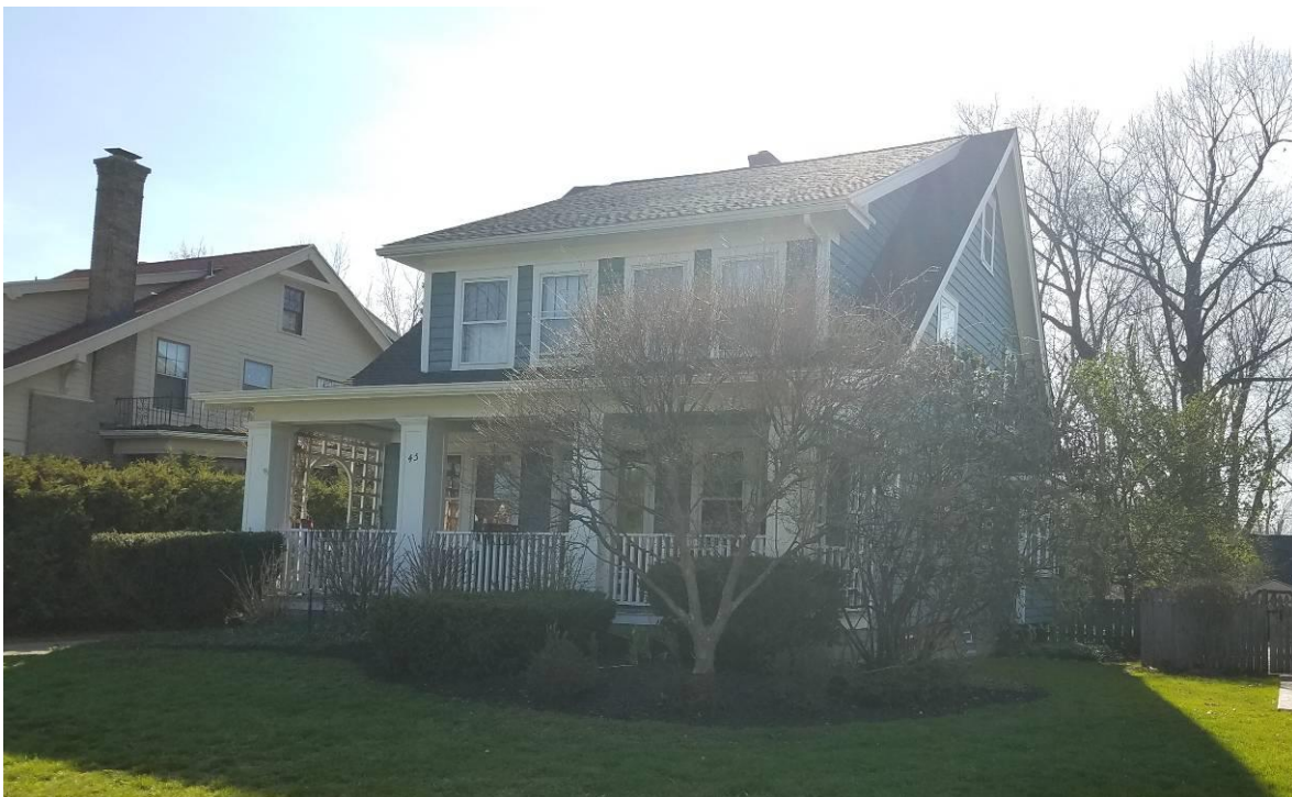
NY_Erie County_ Town of Amherst _45 Roycroft Boulevard_North and East Elevations
