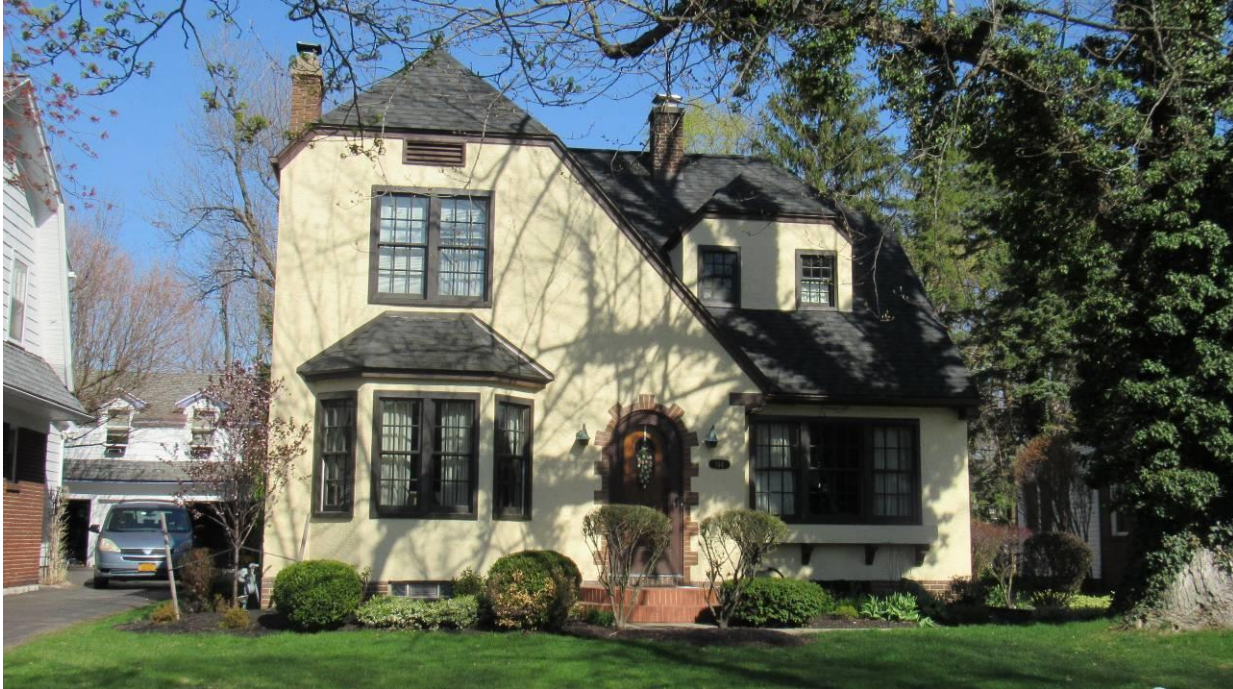
NY_Erie County_ Town of Amherst _144 Darwin Drive_ West Elevation
