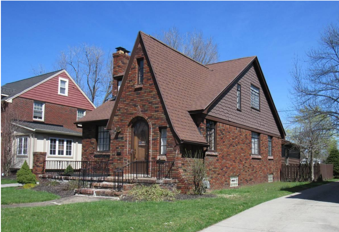
NY_Erie County_ Town of Amherst _212 Berryman Drive_South and West Elevations
