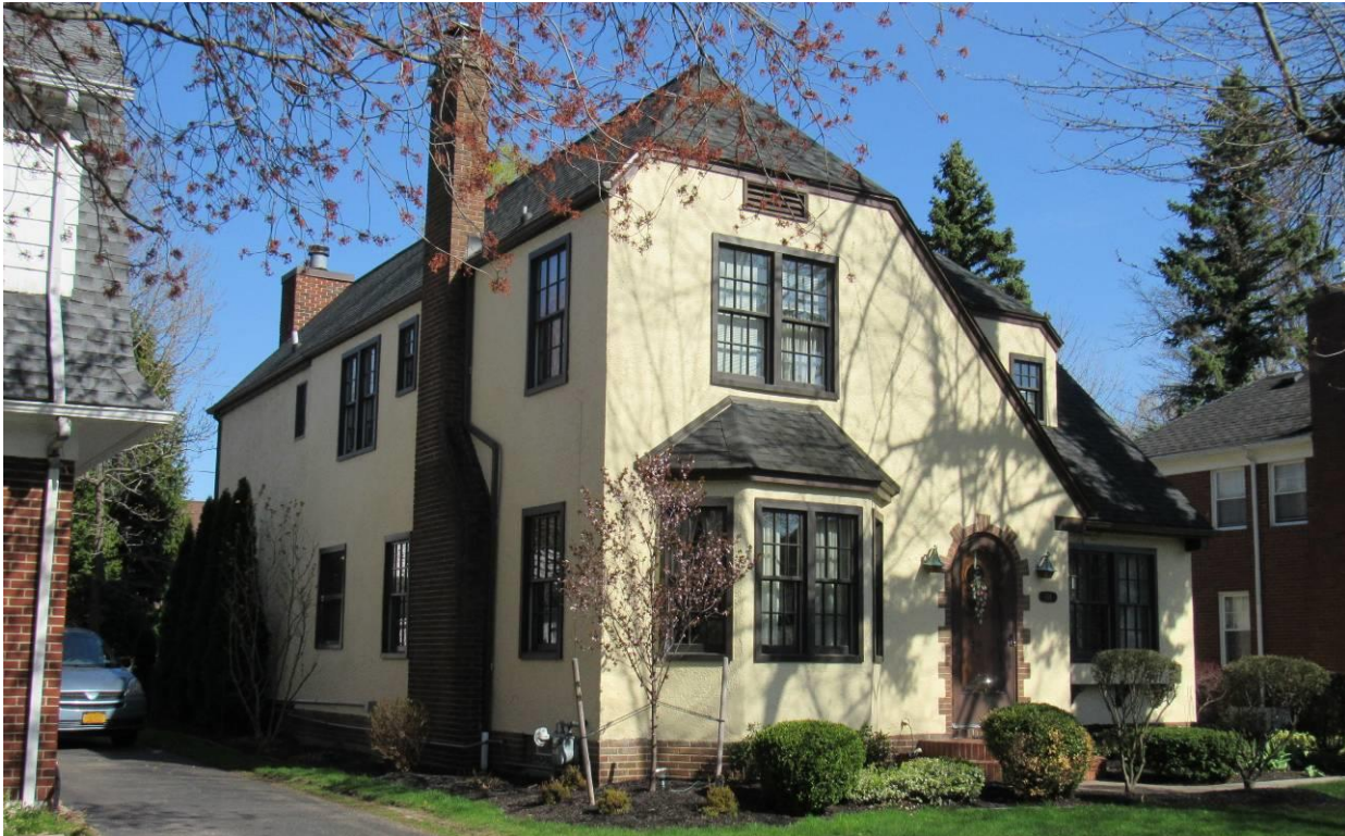
NY_Erie County_ Town of Amherst _144 Darwin Drive_North and West Elevations
