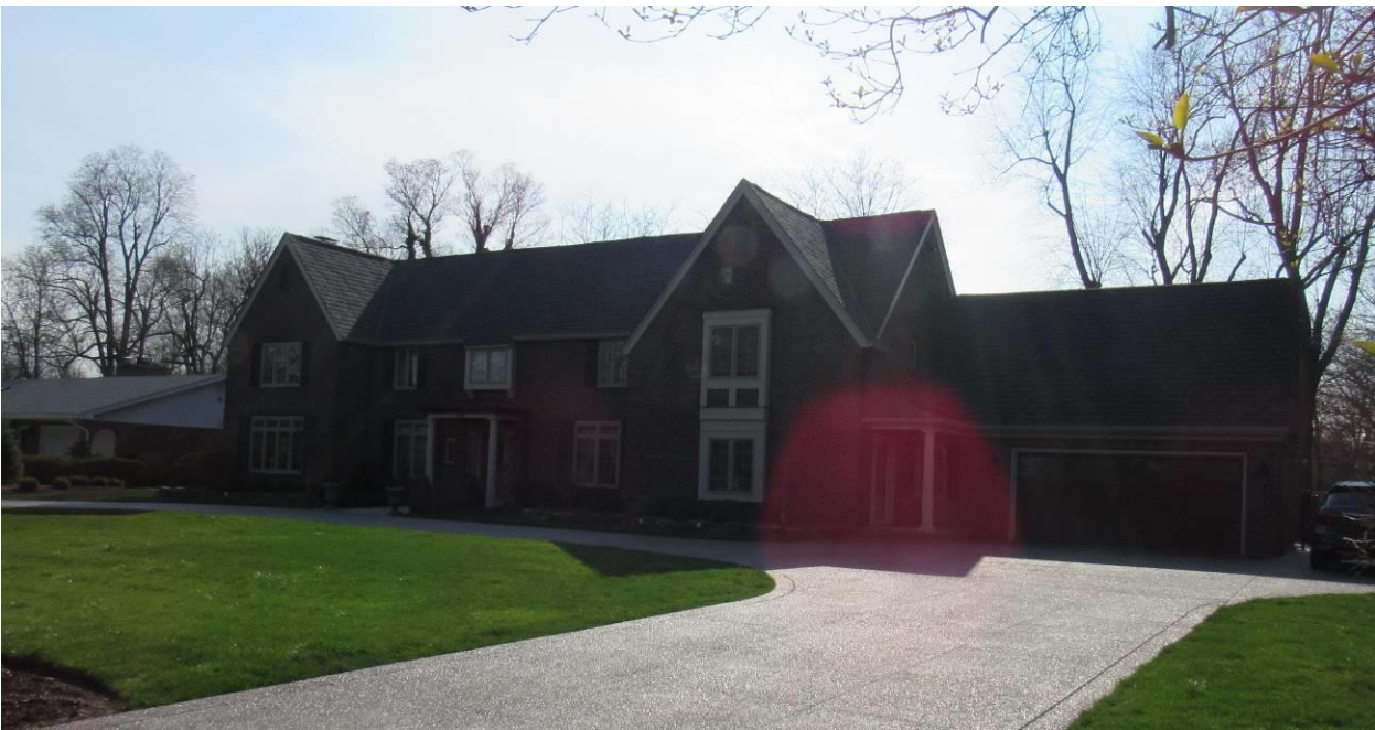
NY_Erie County_ Town of Amherst _880 Le Brun Road_North and East Elevations
