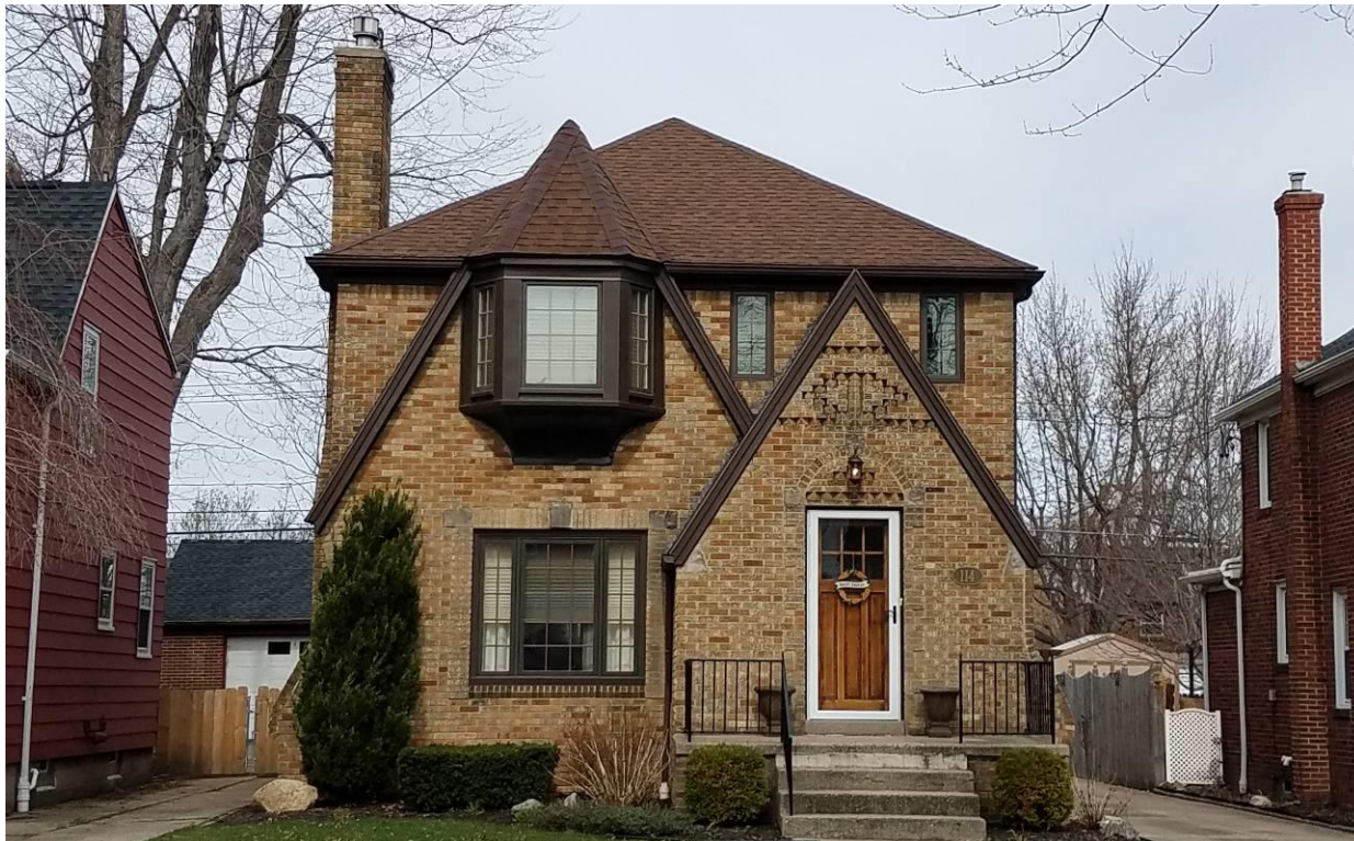
NY_Erie County_ Town of Amherst _114 Hendricks Boulevard_Southwest Elevation
