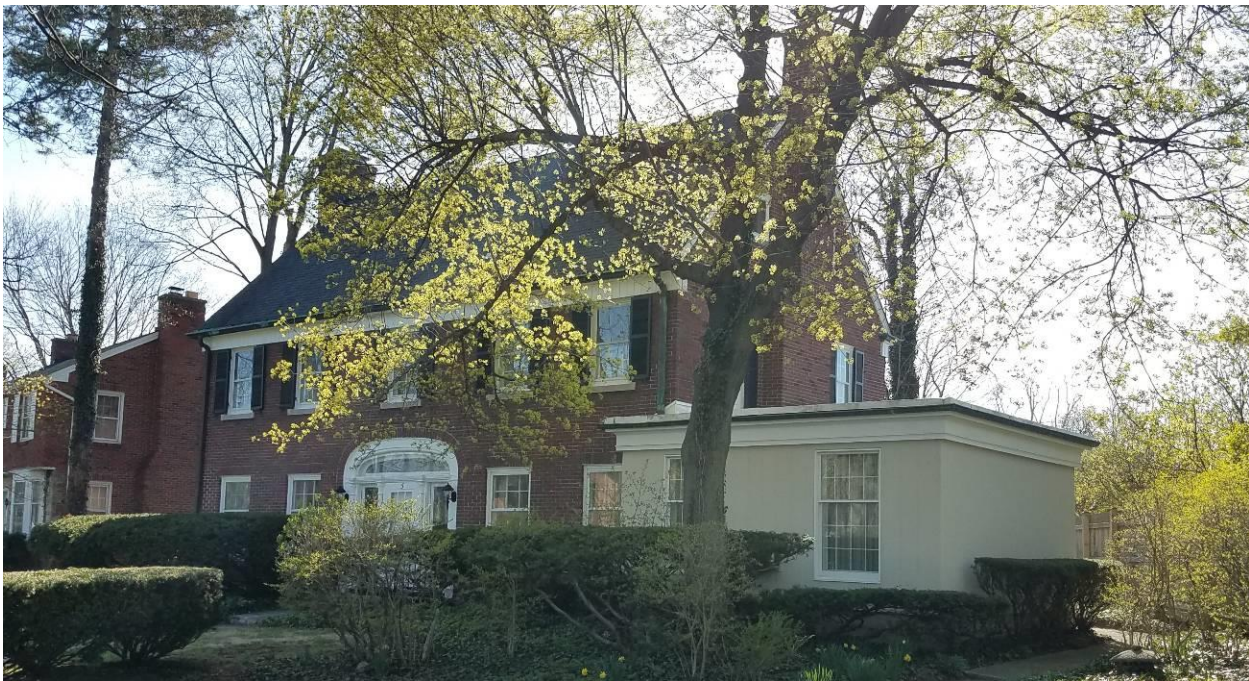
NY_Erie County_ Town of Amherst _5 Darwin Drive_South and East Elevations
