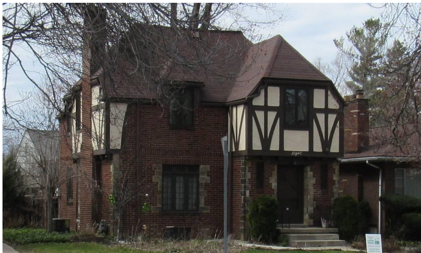
NY_Erie County_ Town of Amherst_8 Hendricks Boulevard_South and West Elevations
