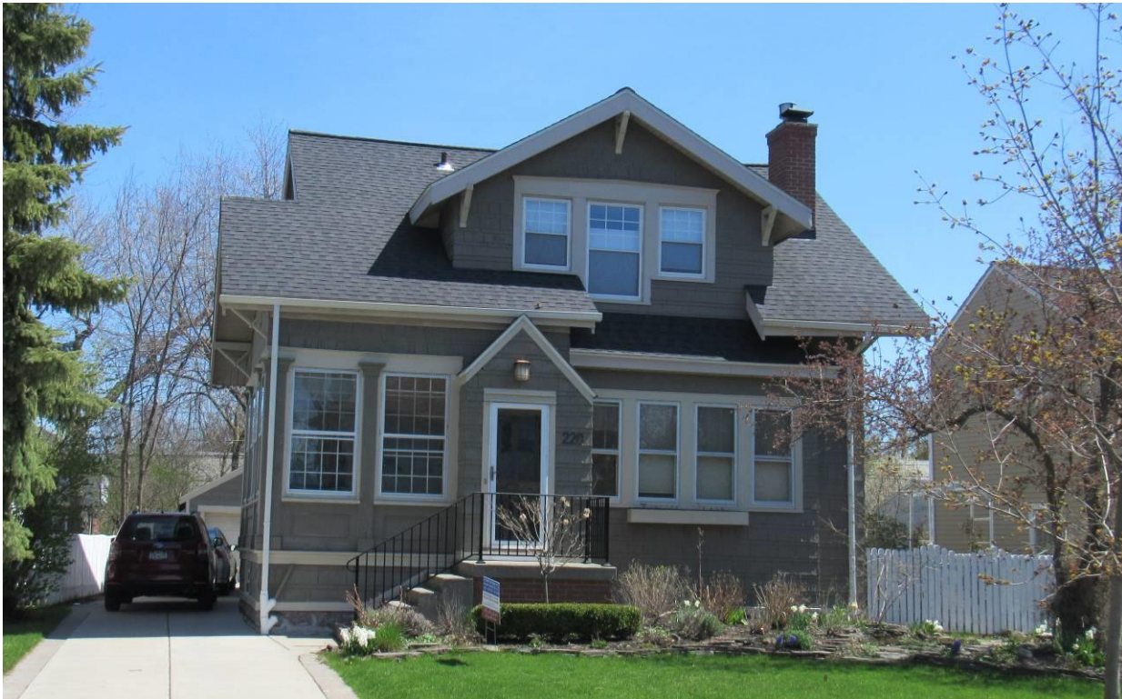
NY_Erie County_ Town of Amherst _220 Washington Highway_North and West Elevations
