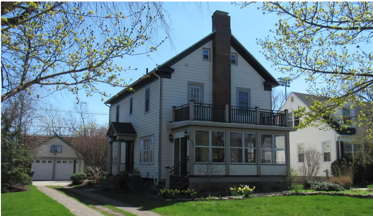
NY_Erie County_ Town of Amherst _120 Berryman Drive_North and West Elevations
