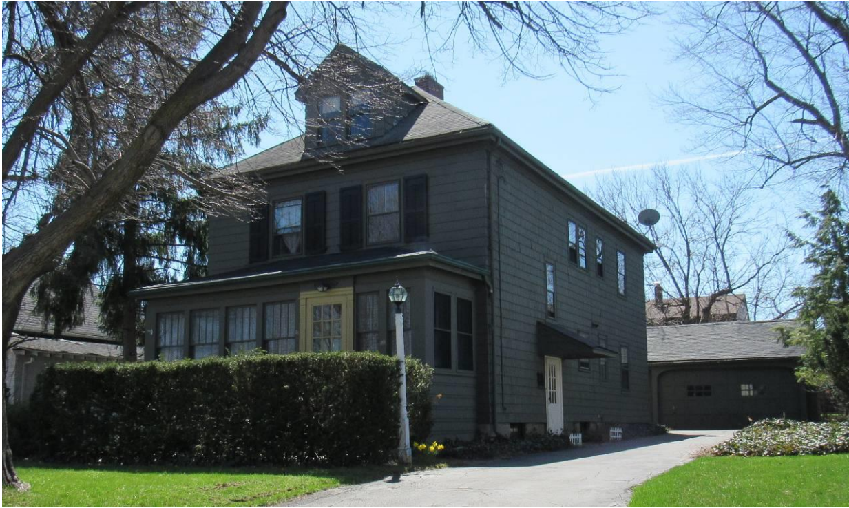
_Erie County_ Town of Amherst _31 Cornell Ave_ North and West Elevations
