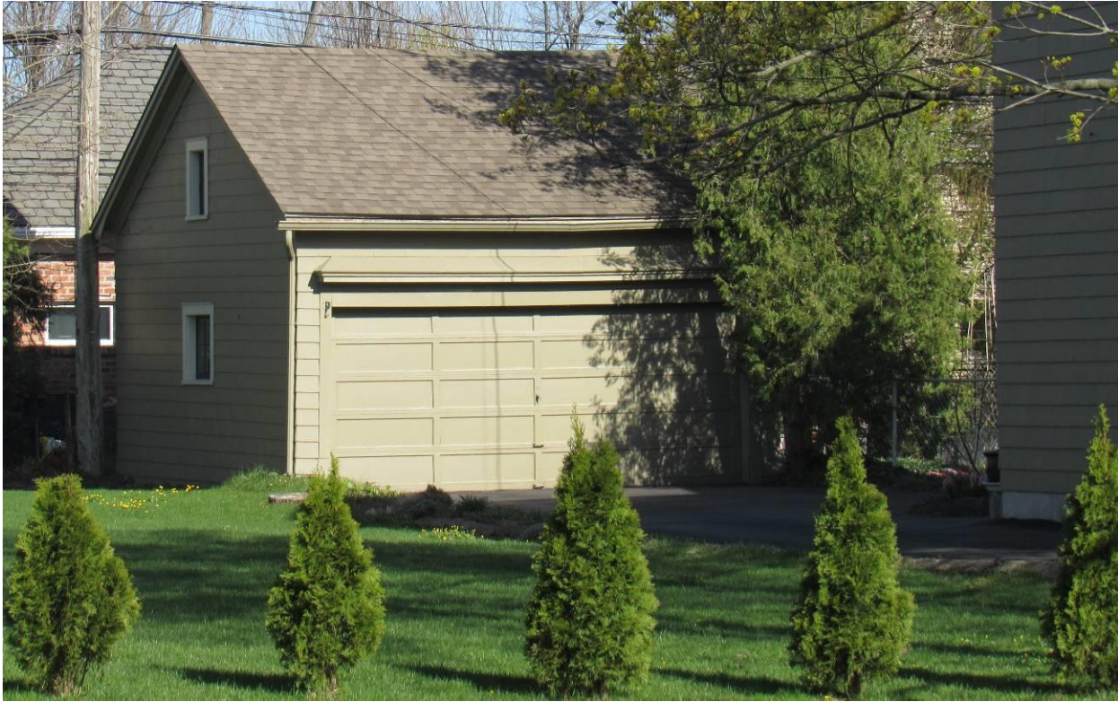
NY_Erie County_ Town of Amherst _48 Roycroft Boulevard_Detached Garage
