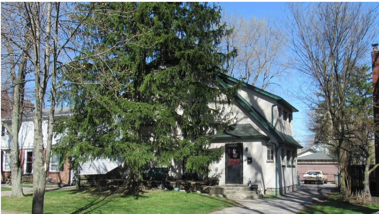
NY_Erie County_ Town of Amherst _244 Roycroft Boulevard_West and South Elevations
