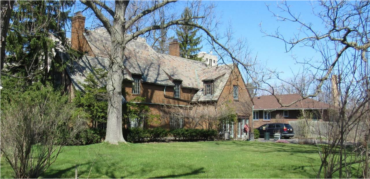
NY_Erie County_ Town of Amherst _107 Le Brun Road_South and West Elevations
