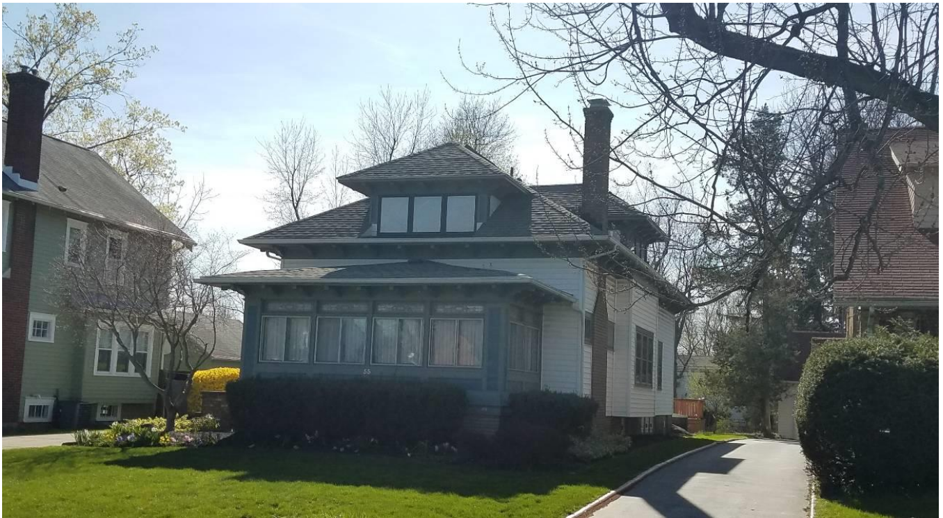
NY_Erie County_ Town of Amherst _55 Roycroft Boulevard_North and East Elevations
