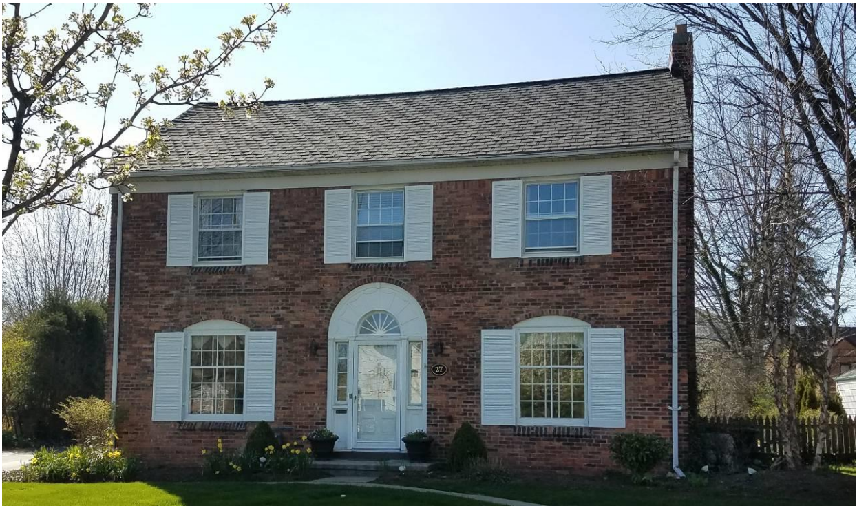
NY_Erie County_ Town of Amherst _27 Darwin Drive_East Elevation
