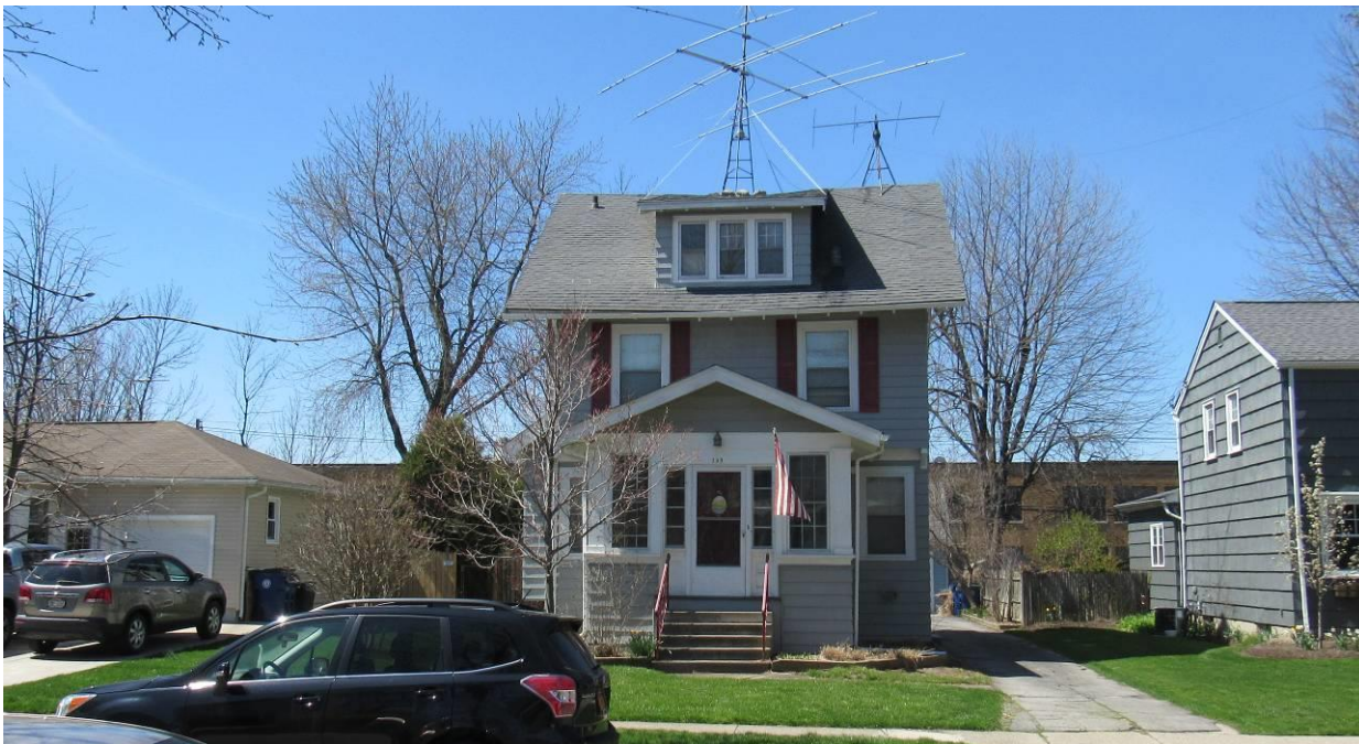
NY_Erie County_Town of Amherst_309 Washington Highway_East Elevation
