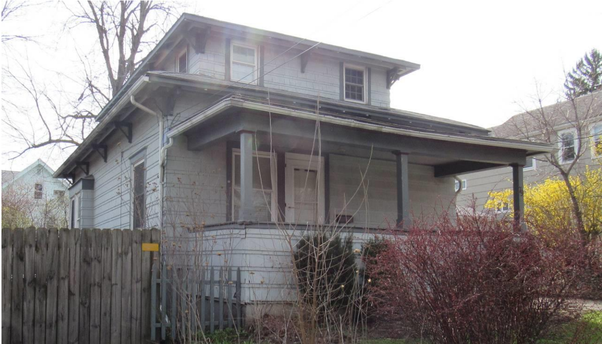
NY_Erie County_ Town of Amherst _79 Callodine Avenue_North and West Elevations
