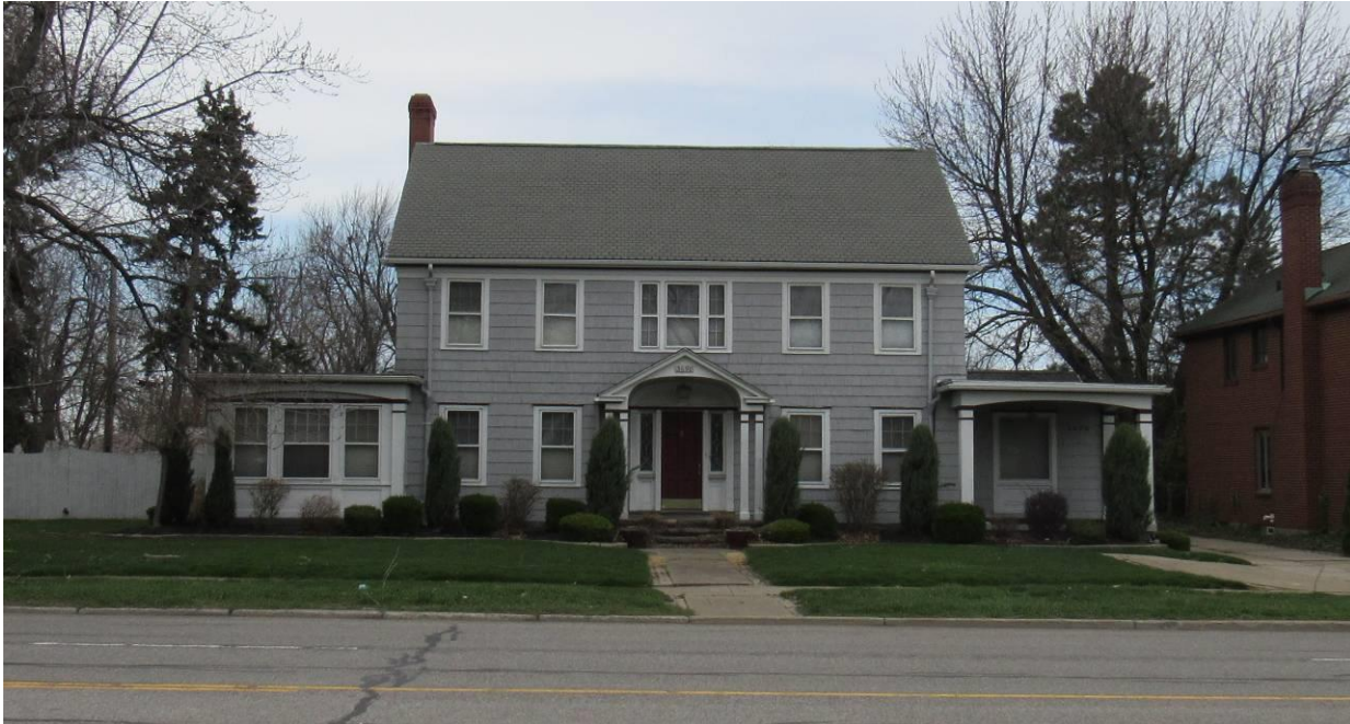
NY_Erie County_ Town of Amherst _3690 Main Street_South Elevation
