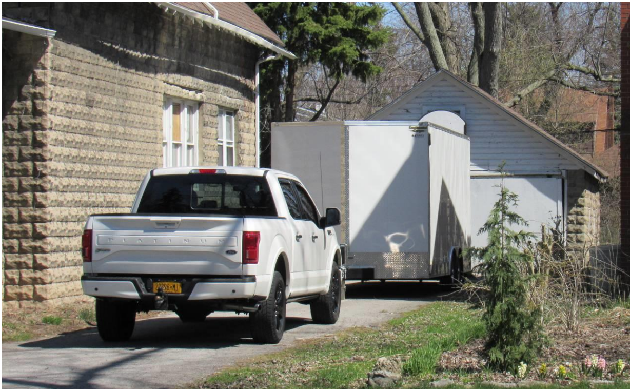
NY_Erie County_ Town of Amherst _125 Westfield Road_South and West Elevations_Detached Garage
