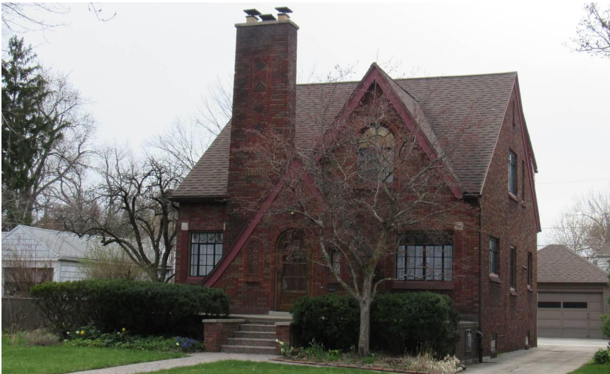
NY_Erie County_ Town of Amherst _38 Endicott Drive_Northeast and Northwest Elevations
