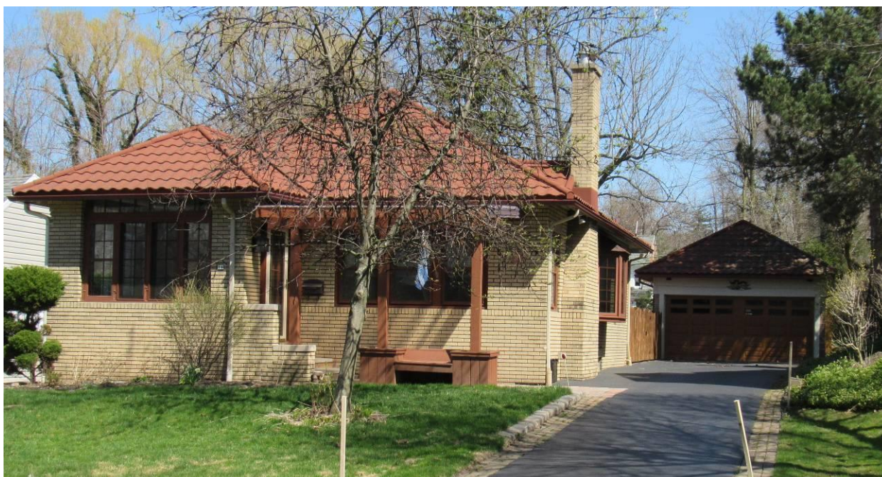
NY_Erie County_ Town of Amherst _79 Ivyhurst Road_South and West Elevations
