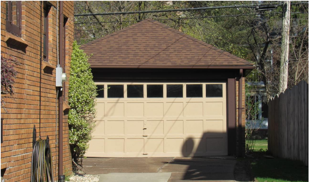
NY_Erie County_ Town of Amherst _32 Roycroft Boulevard_Detached Garage
