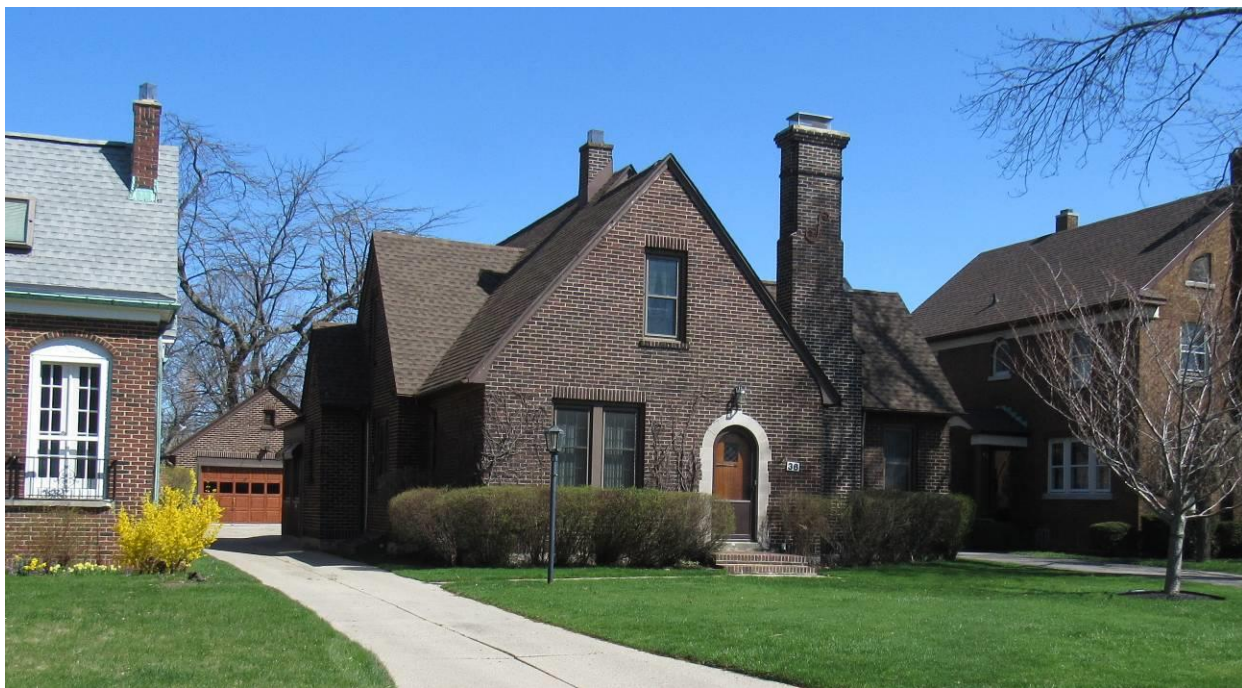
NY_Erie County_ Town of Amherst_36 South Drive_South and West Elevations
