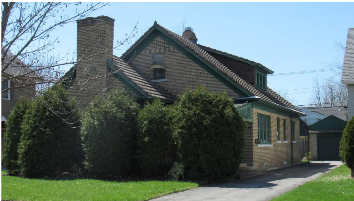
NY_Erie County_ Town of Amherst _133 Berryman Drive_North and East Elevaitons
