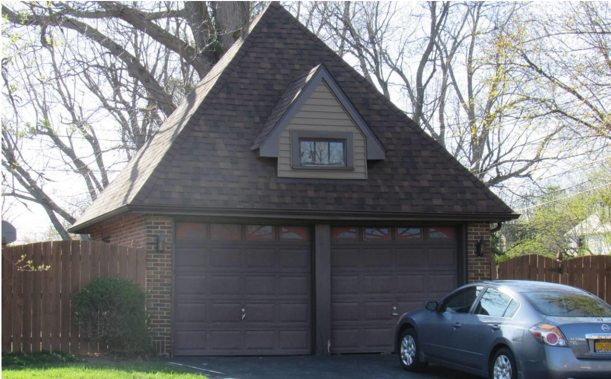
NY_Erie County_ Town of Amherst _114 Saratoga Road_East Elevation_Detached Garage
