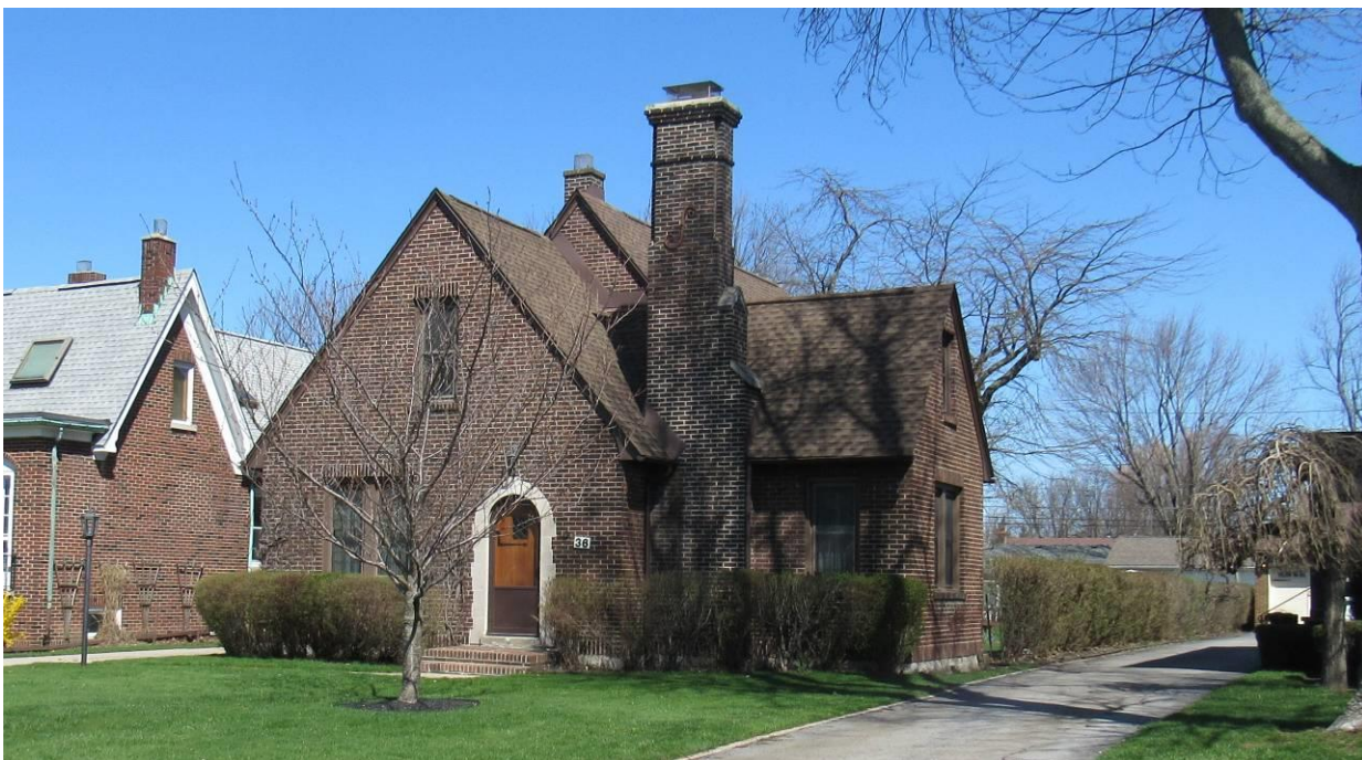
NY_Erie County_ Town of Amherst _36 South Drive_South and East Elevations
