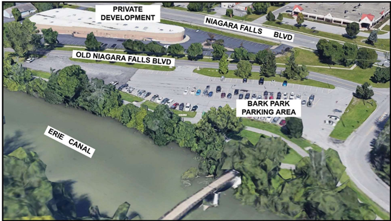
OLD NIAGARA FALLS BOULEVARD EXISTING CONDITIONS
