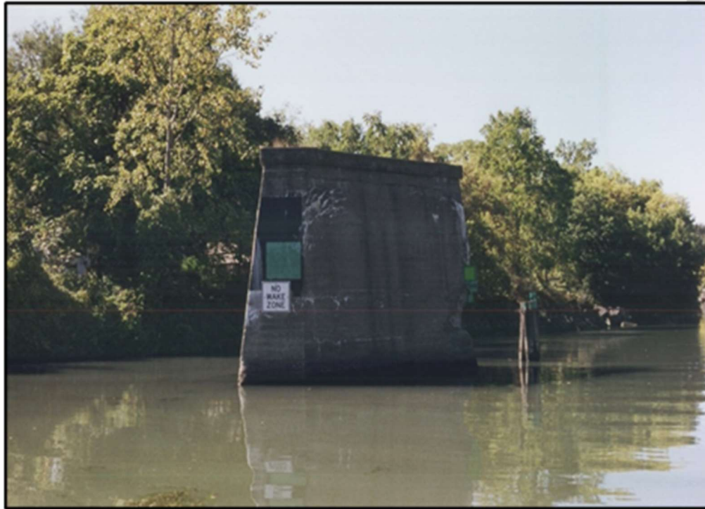
Figure 2.44 – Old bridge abutment west of Bear Ridge Road
