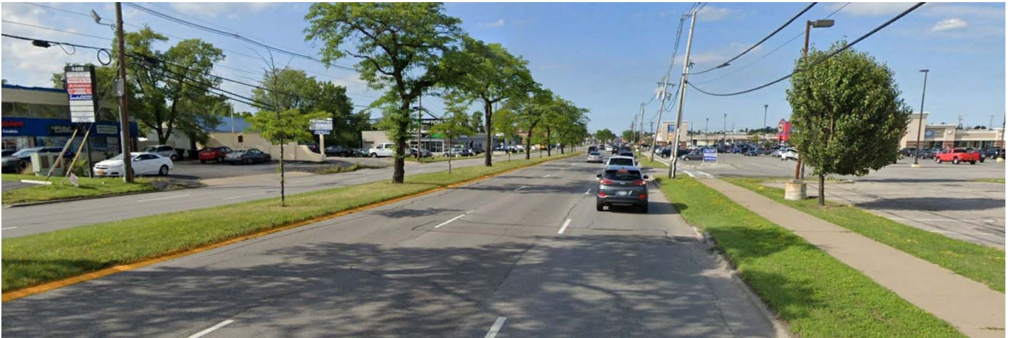
Figure 13: Niagara Falls Boulevard (north of Maple Road)
