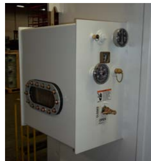
Figure 7. External visible break with gauges
