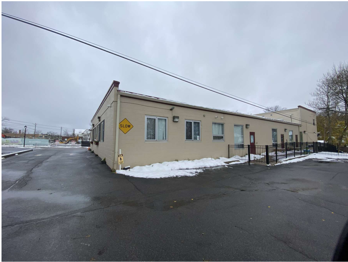
Southeast Corner of Building
