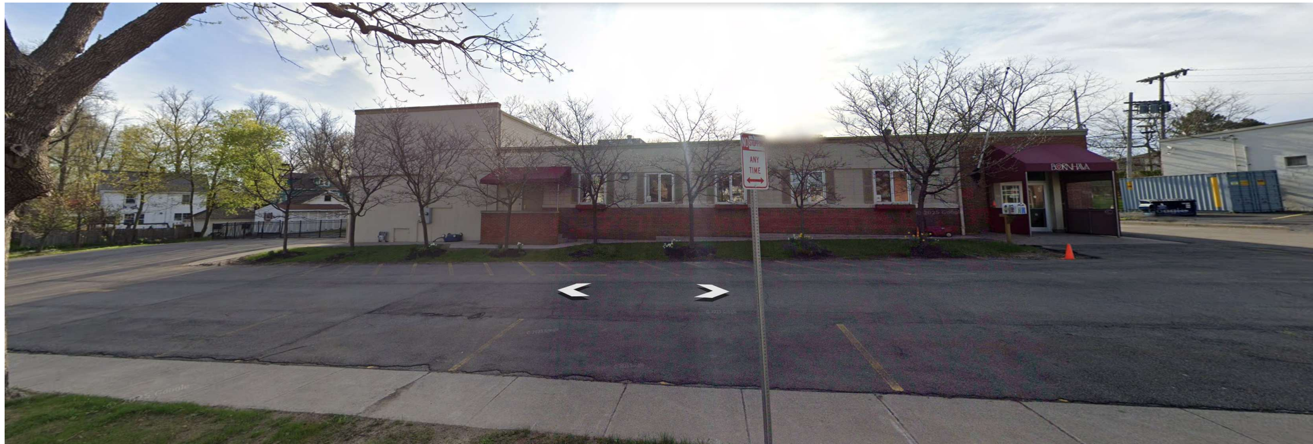
West Building Elevation - Street View
