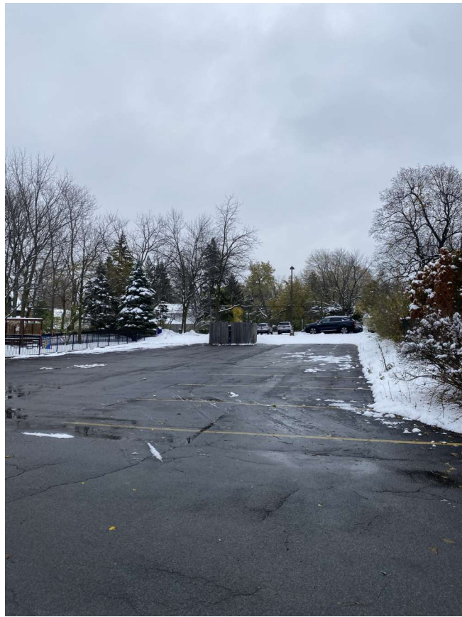
Rear Parking Lot
