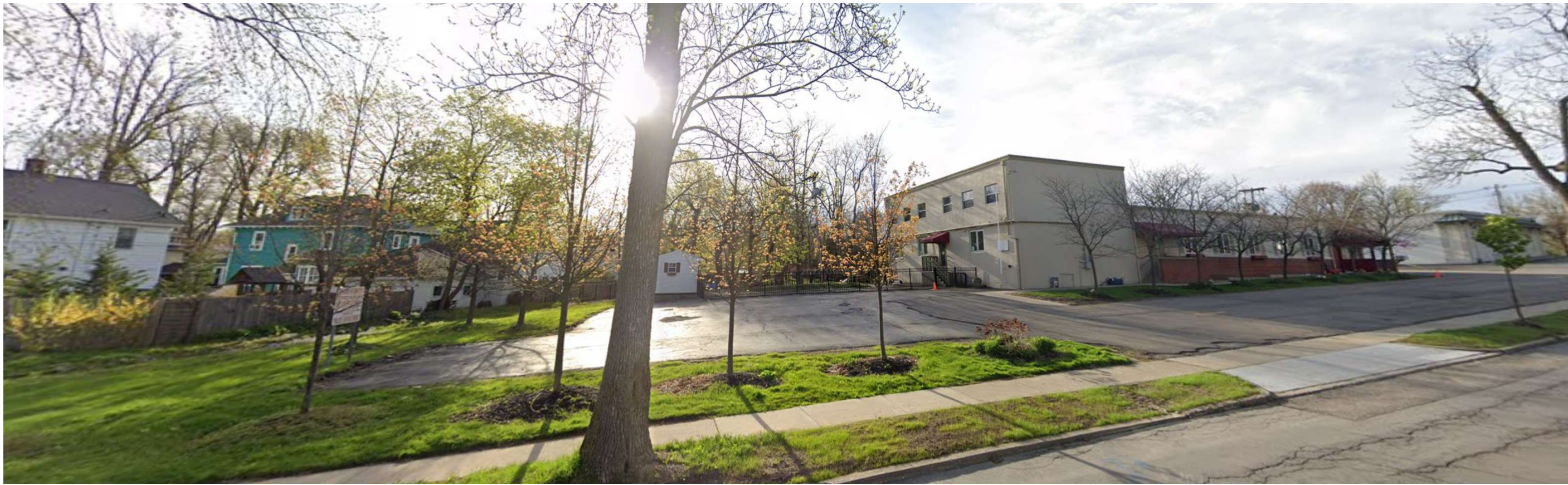
Northwest Corner of Building - Street View
