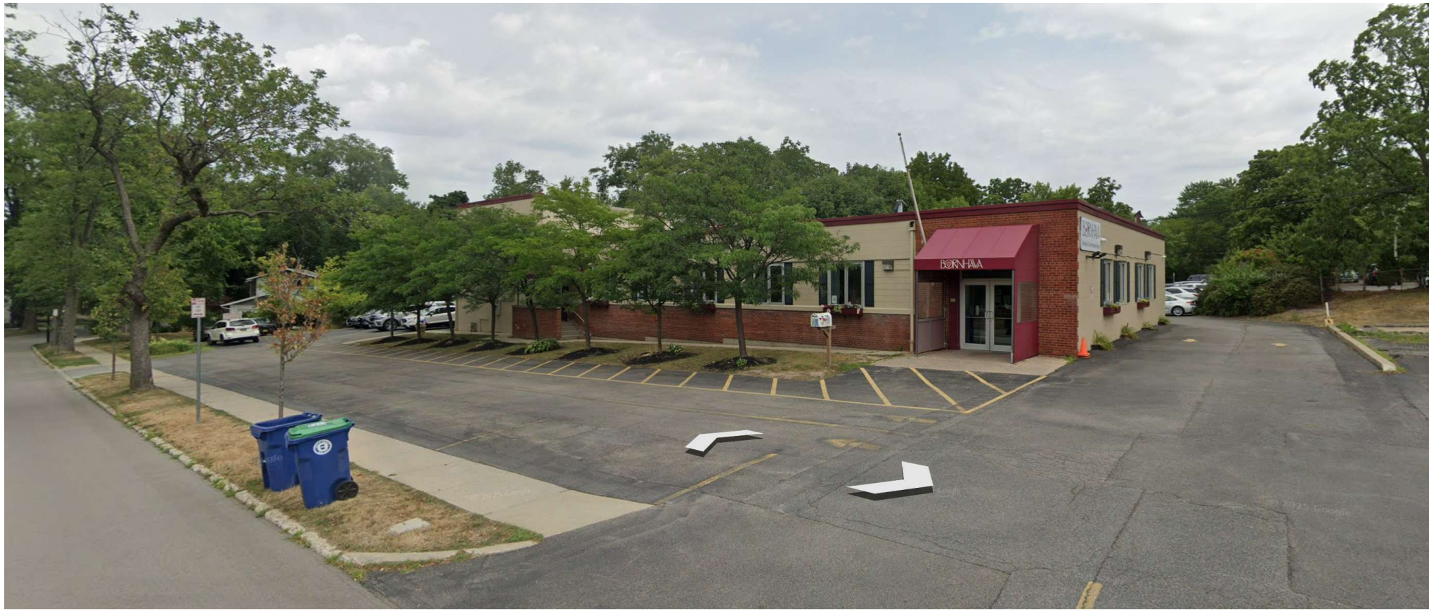
Southwest Corner of Building - Street View
