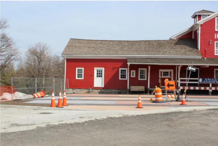
The old mill site is a stormwater project in the Village. Permeable brick pavers help to capture stormwater runoff.
