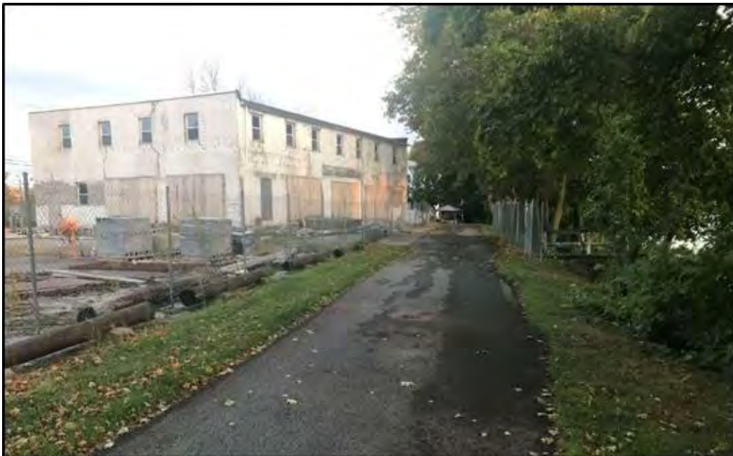
Figure 2.27 - Old Niagara Falls Boulevard Underused Parcel
