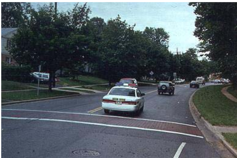
Example of alternatively paved crosswalk. Local examples exist along Main Street in the University Heights district of Buffalo and in the Village of Lewiston.
