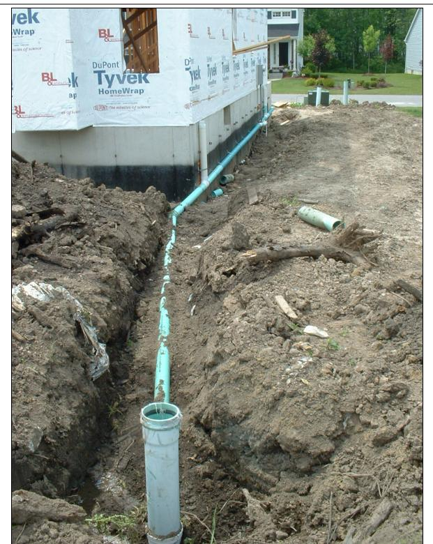
Photo 3. Downspout drainage system discharging to rear yard collector in north Amherst , NY (June 2004). Damage from construction, frost, soil subsidence, and clogging are common reported problems.
