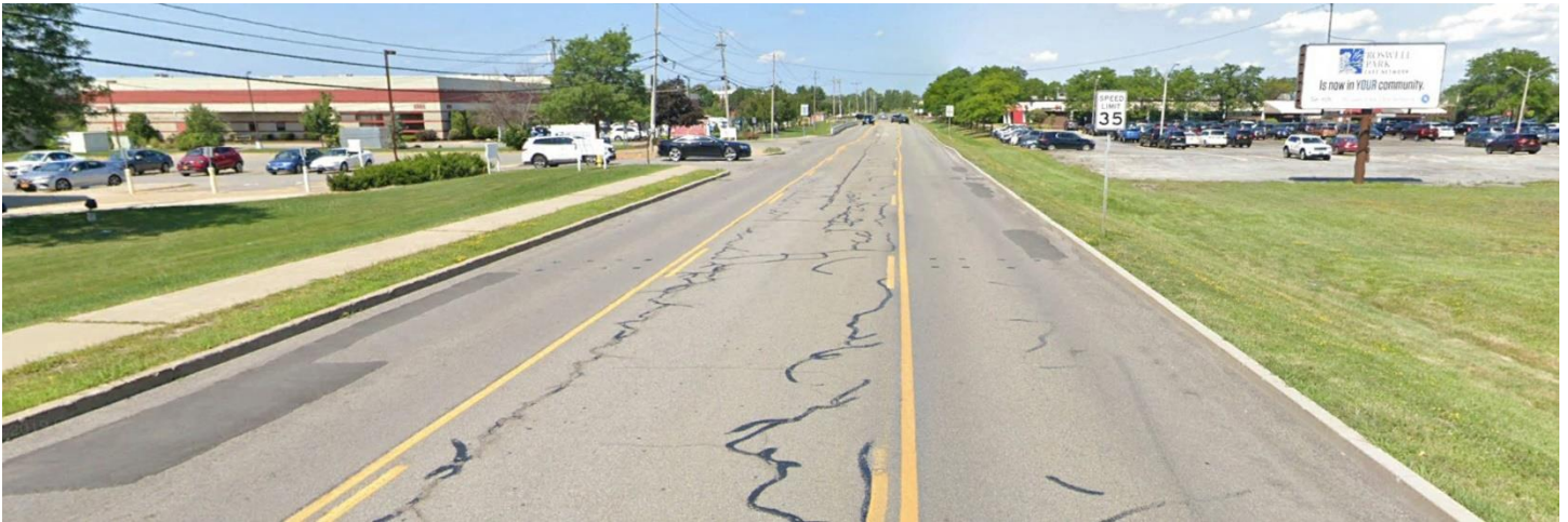
Figure 15: Bailey Avenue (north of Maple Road)
