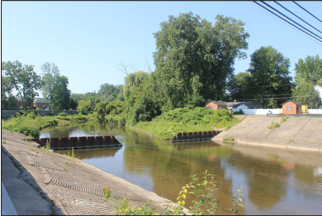
Figure 2.38 - USACE Channelized Creek at Bottom of Channel 579.0' Elevation, south of Maple St.
