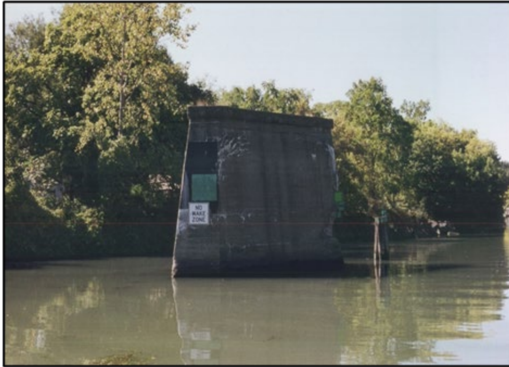
Figure 2.44 – Old bridge abutment west of Bear Ridge Road
