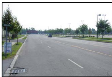
Direct access to commercial development from collector street avoids the need to access the arterial.
